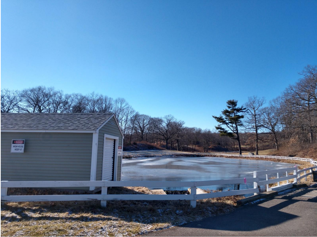
Photo 1: Pump House and Unnamed Pond in January 2019
