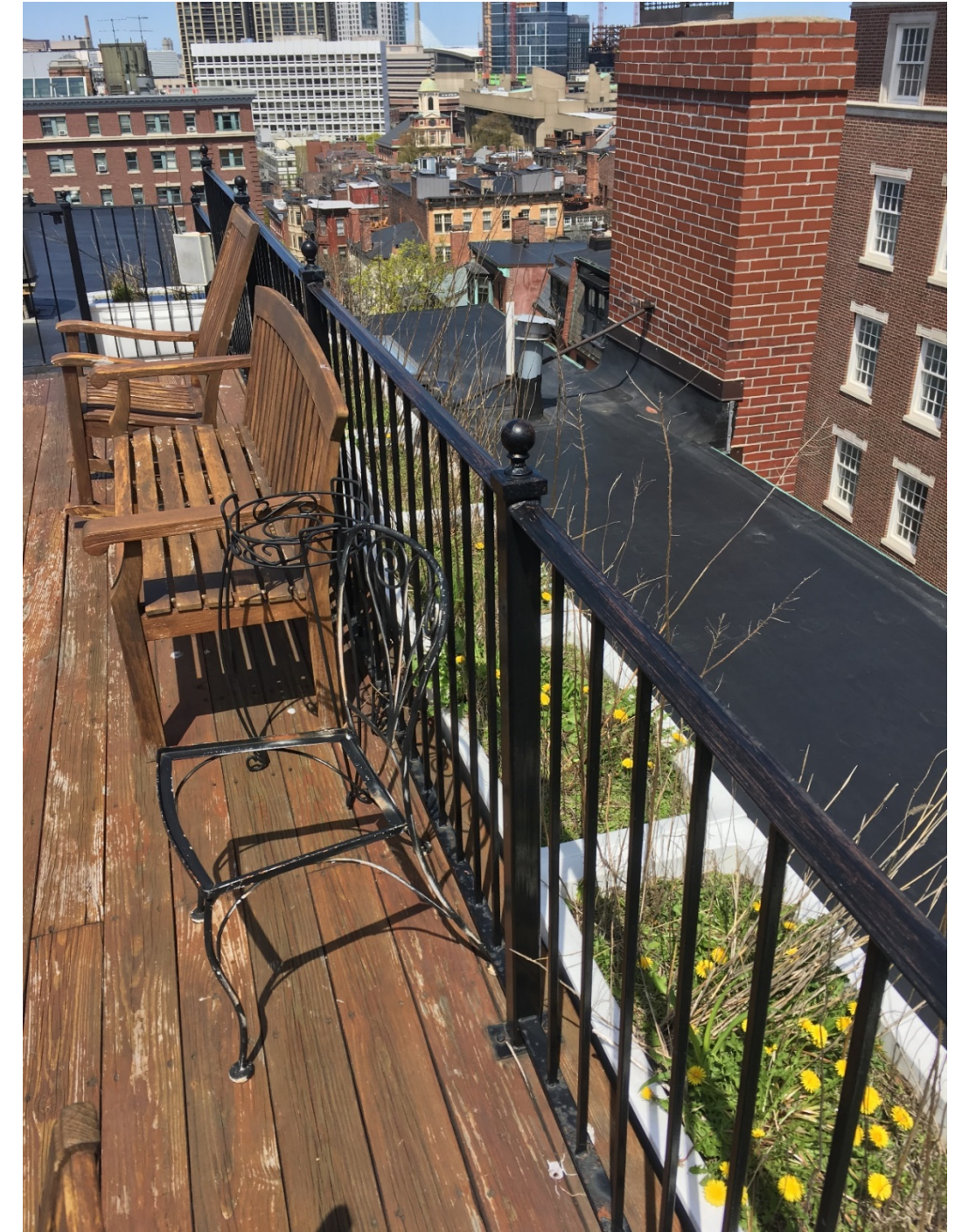
View 3 : Joy St. side from deck
