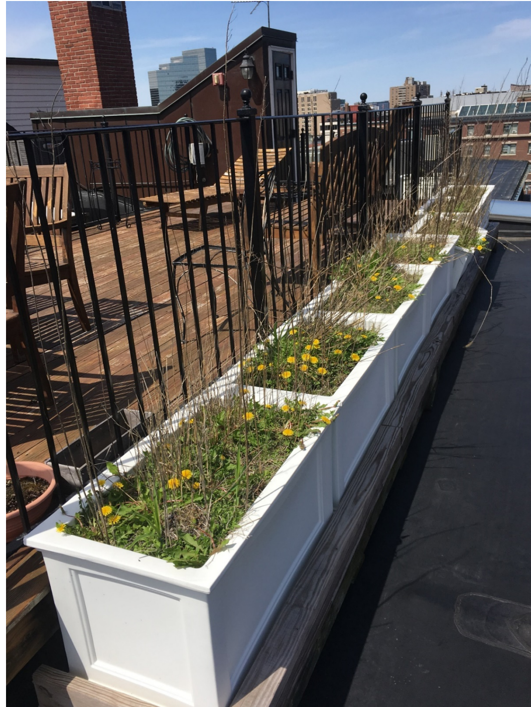
View 2 : Joy St. side of deck
