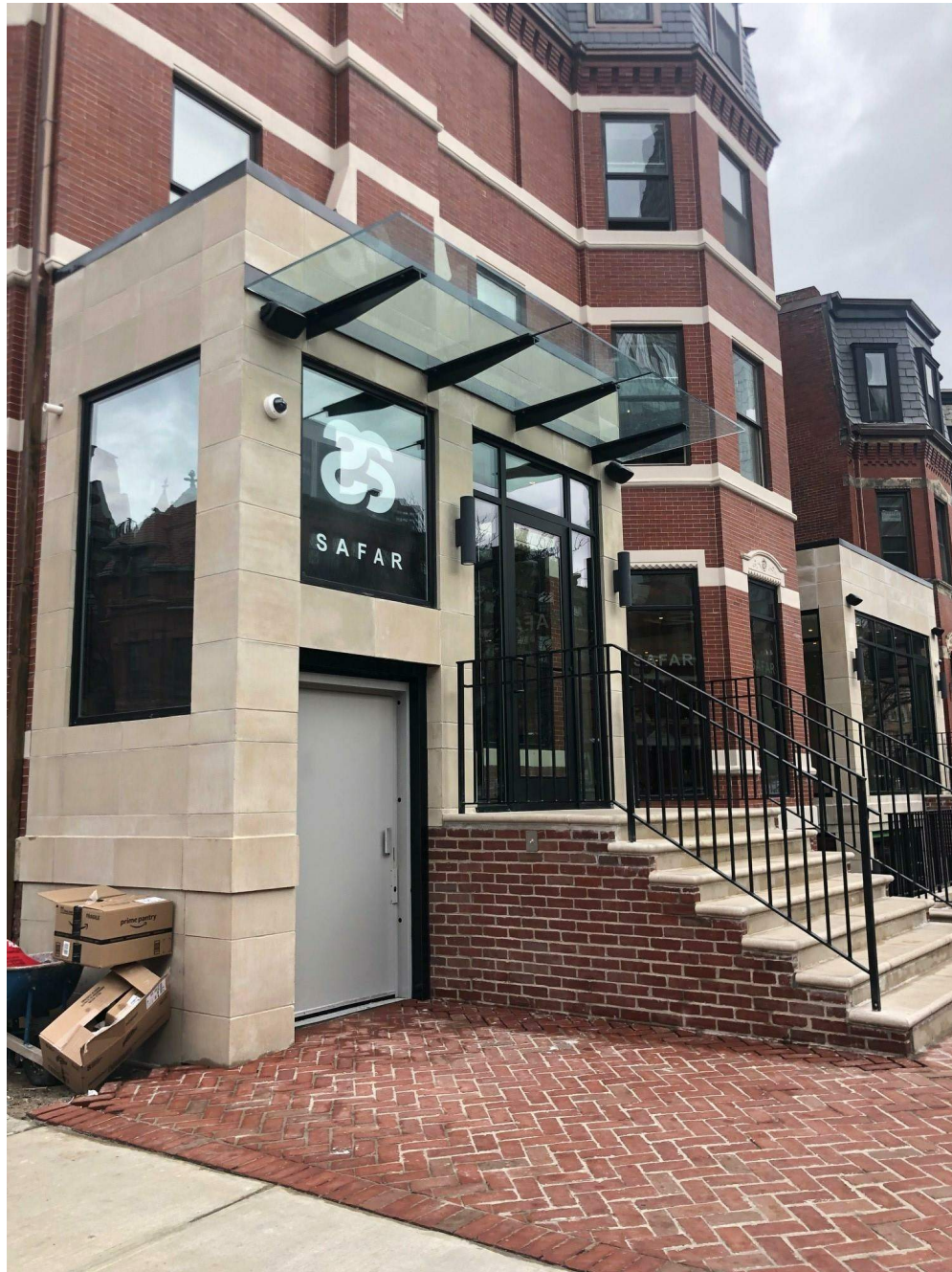
VIEW OF PATIO AREA 'A'
