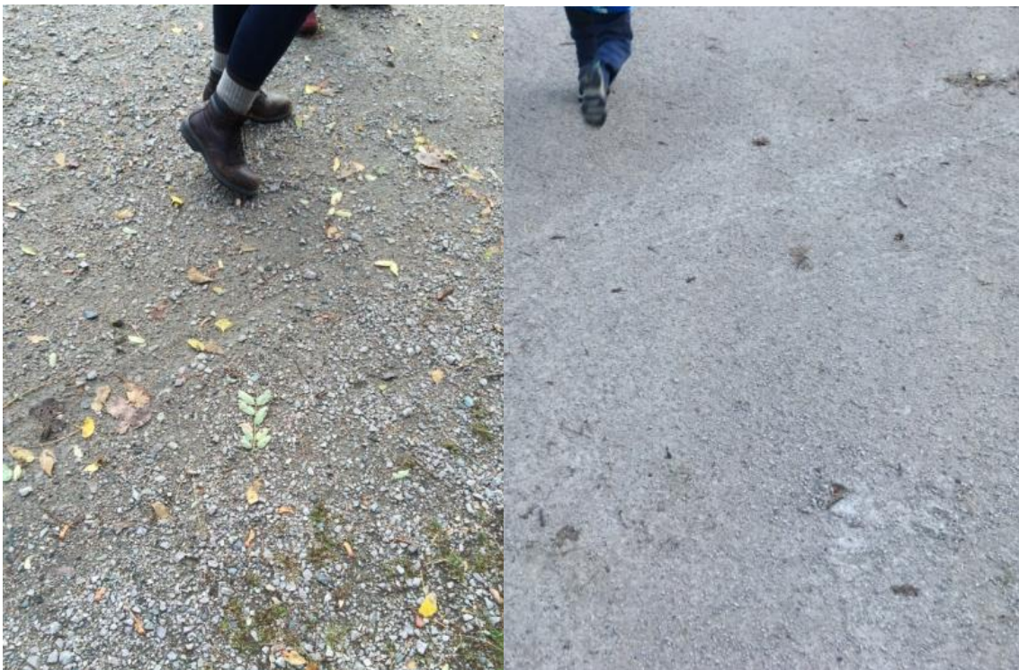
Photo 8. Photos of dense grade stone along the Blackwell Footpath (left) and stabilized soil in Quincy, MA (right).
