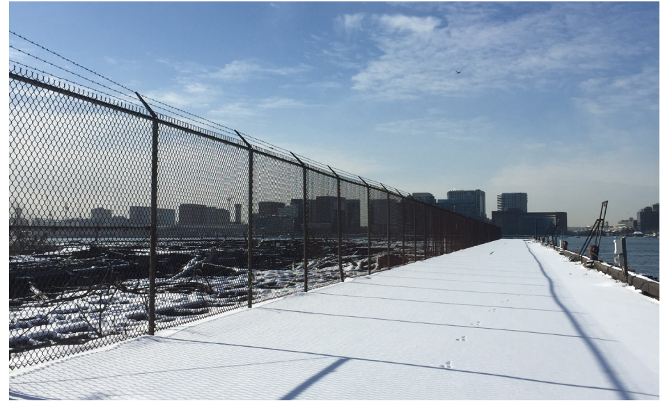
View 2: Looking Southwest along Concrete Apron
