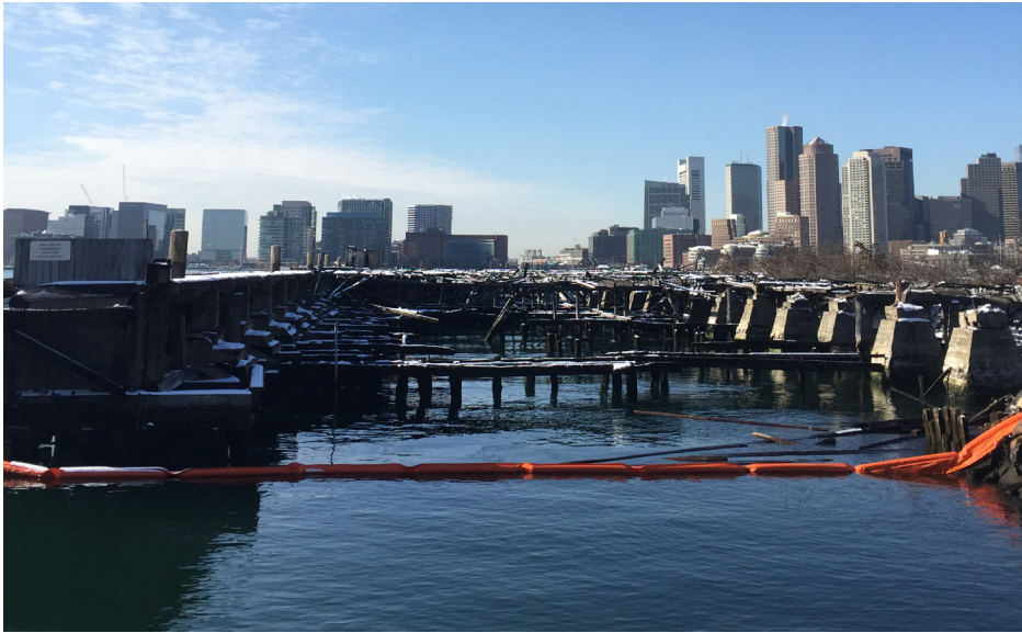
View 1: Looking Southwest toward Project Site
