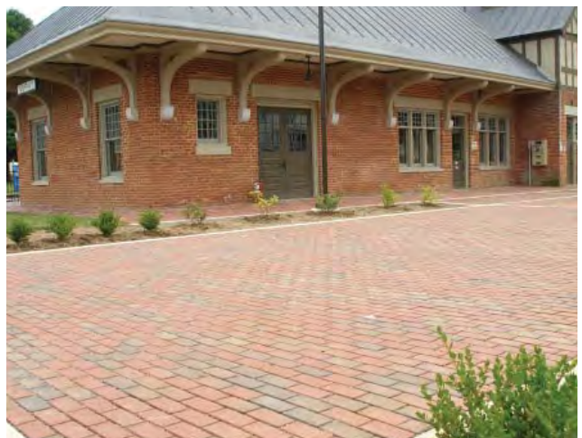
Photo courtesy Pine Hall Brick Company, Inc.
