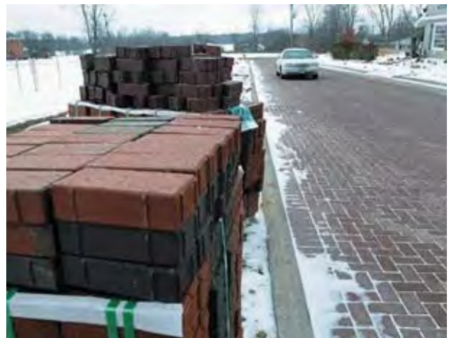
Photo 3 Permeable Clay Brick Street Installed as Part of a CSO Reduction Program
