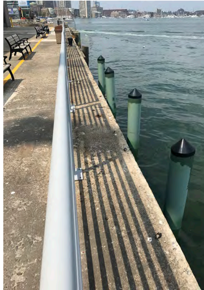
Fender piles on the north end of the pier
