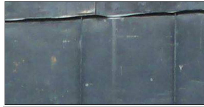
Existing Metal Panel System (Rear Facade)
