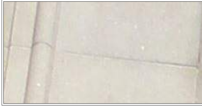
Existing Stone Veneer (Front Facade)
