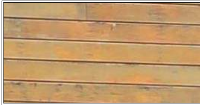
Existing Wood Facade (Front Facade)
