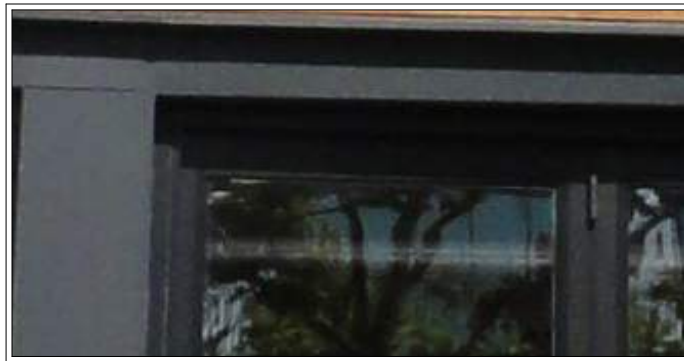
Existing Storefront System (Front Facade)
