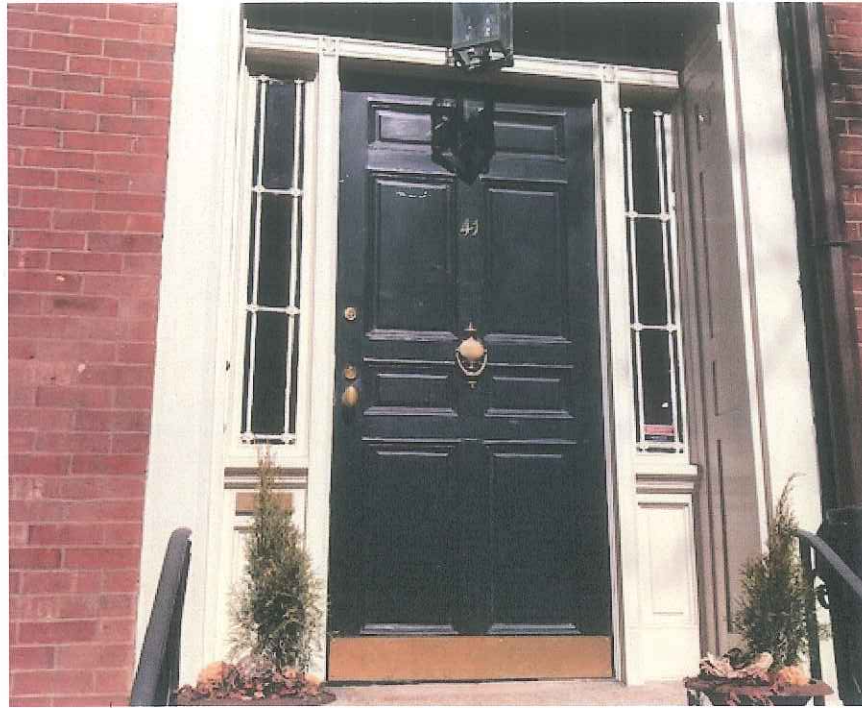
1. EXISTING DOOR AT 41 CHESTNUT STREET
