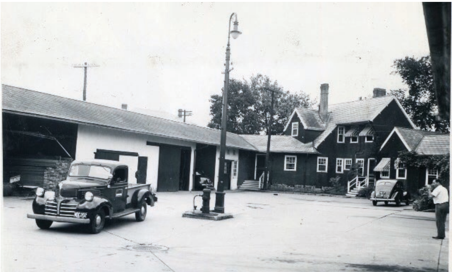
Figure 86: upper Courtyard Photo cir. 1946
