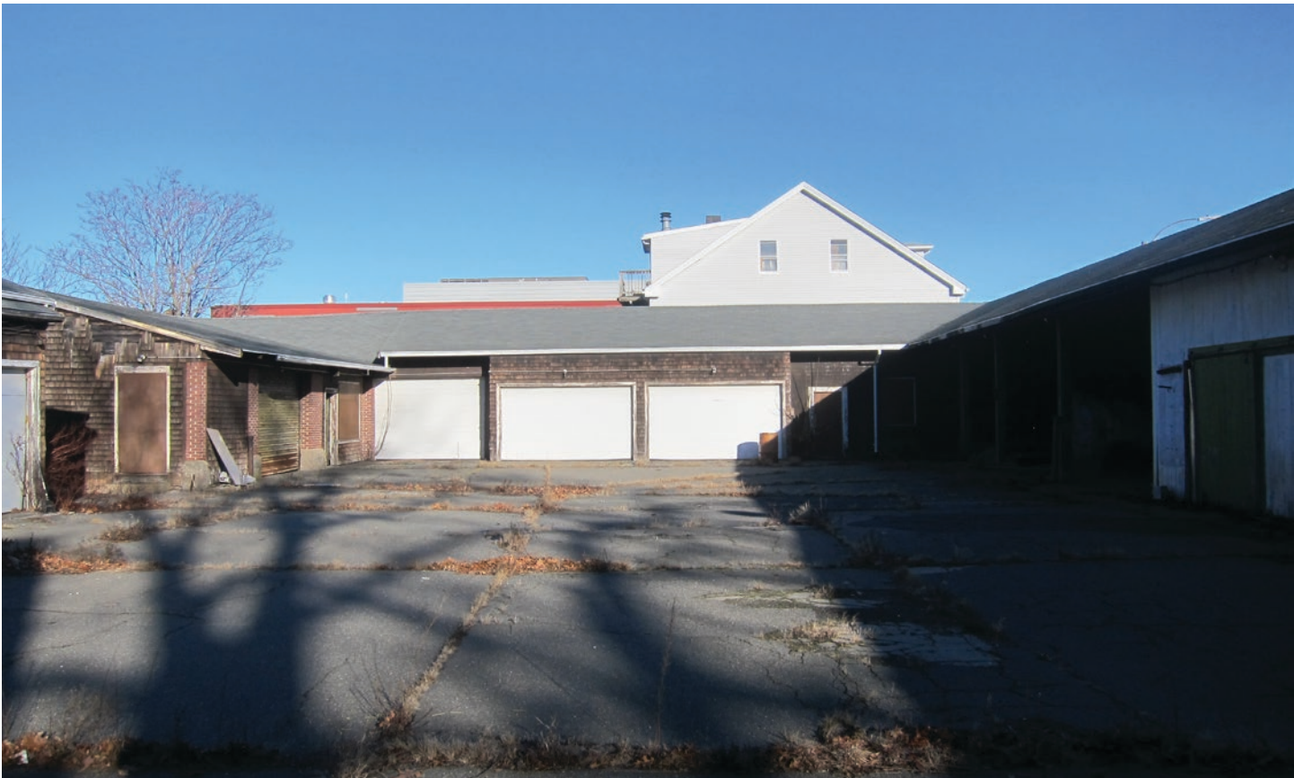
Figure 27: Building D Garage Additions
