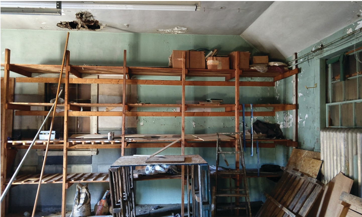
Figure 78: Building H Interior
