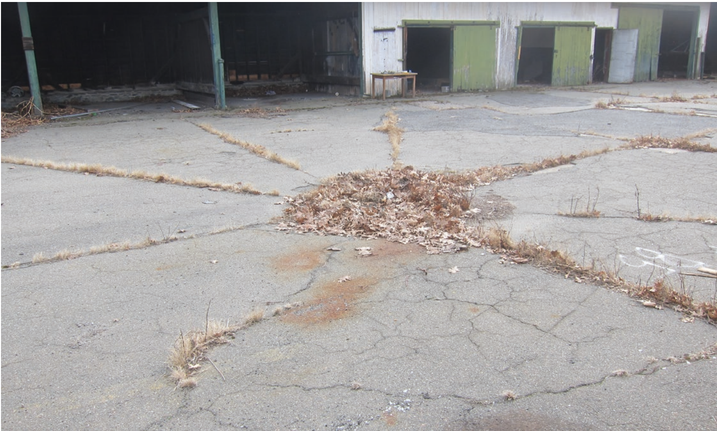
Figure 85: upper Courtyard Catch Basin
