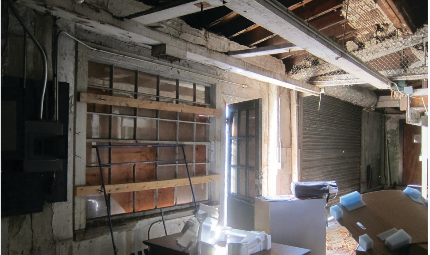
Figure 68: Building D Interior
