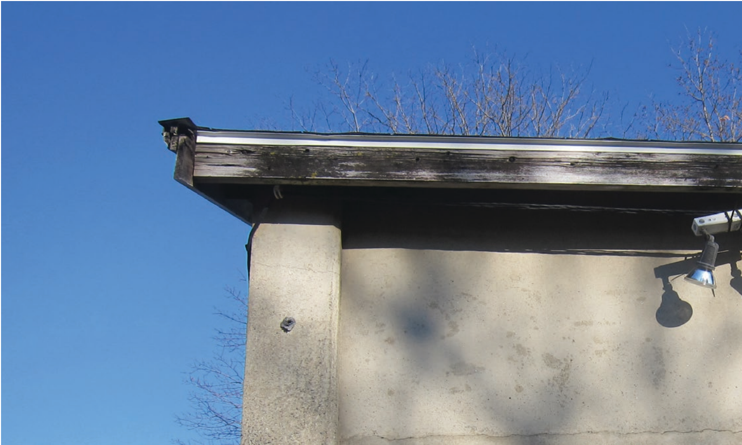
Figure 17: Building B Fascia
