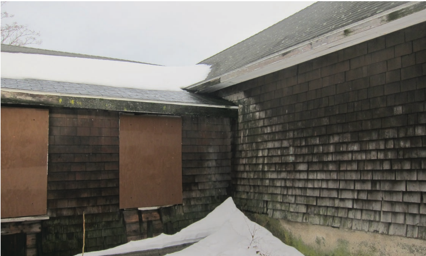
Figure 53: Building C and D Roofs
