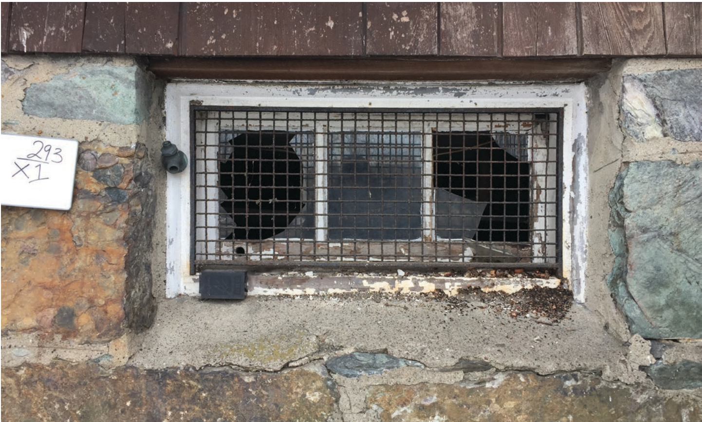
Figure 48: Building H Basement Hopper Window
