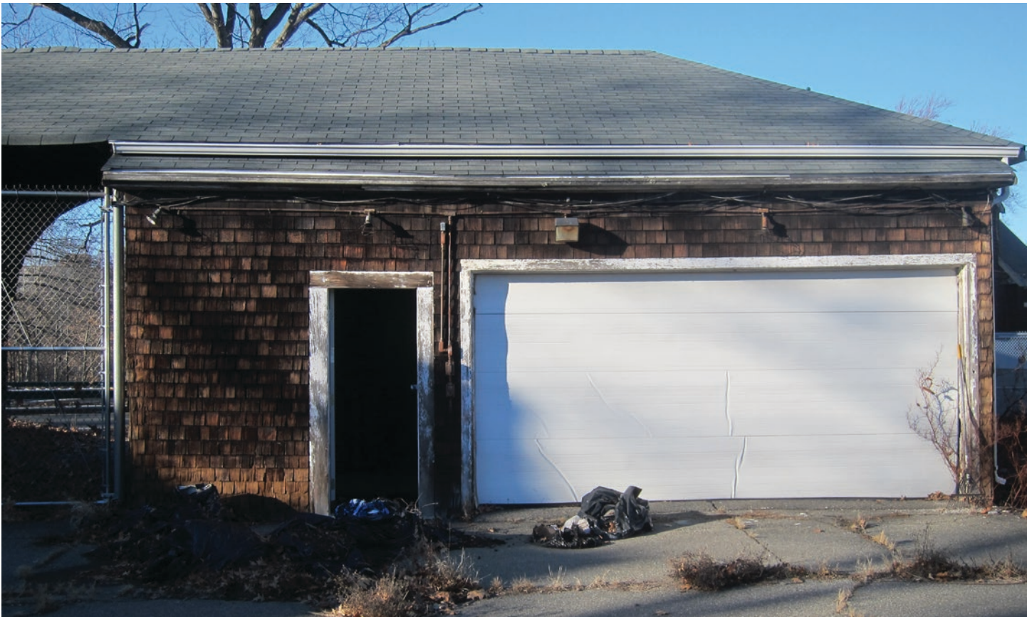
Figure 35: Building H Garage Door Addition
