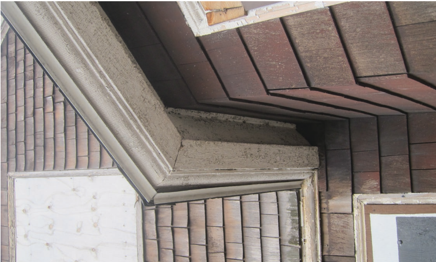
Figure 22: Building F Exterior Wood Trim
