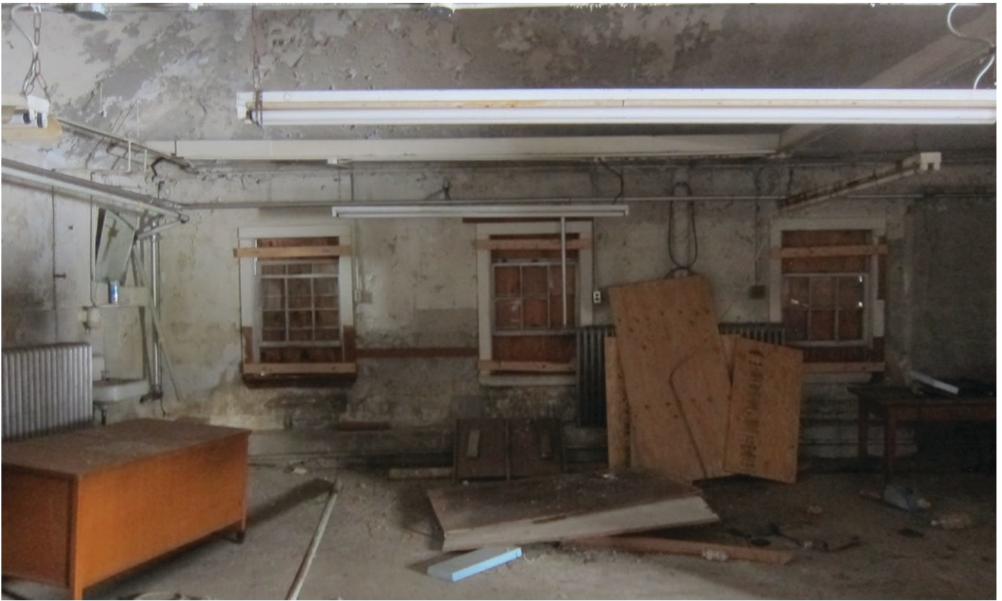
Figure 67: Building D Interior
