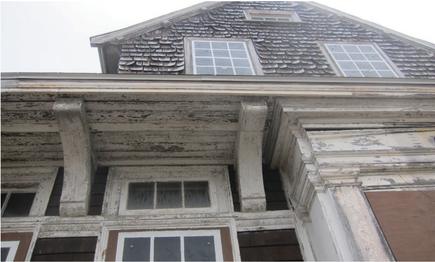
Figure 23: Building H Exterior Wood Trim
