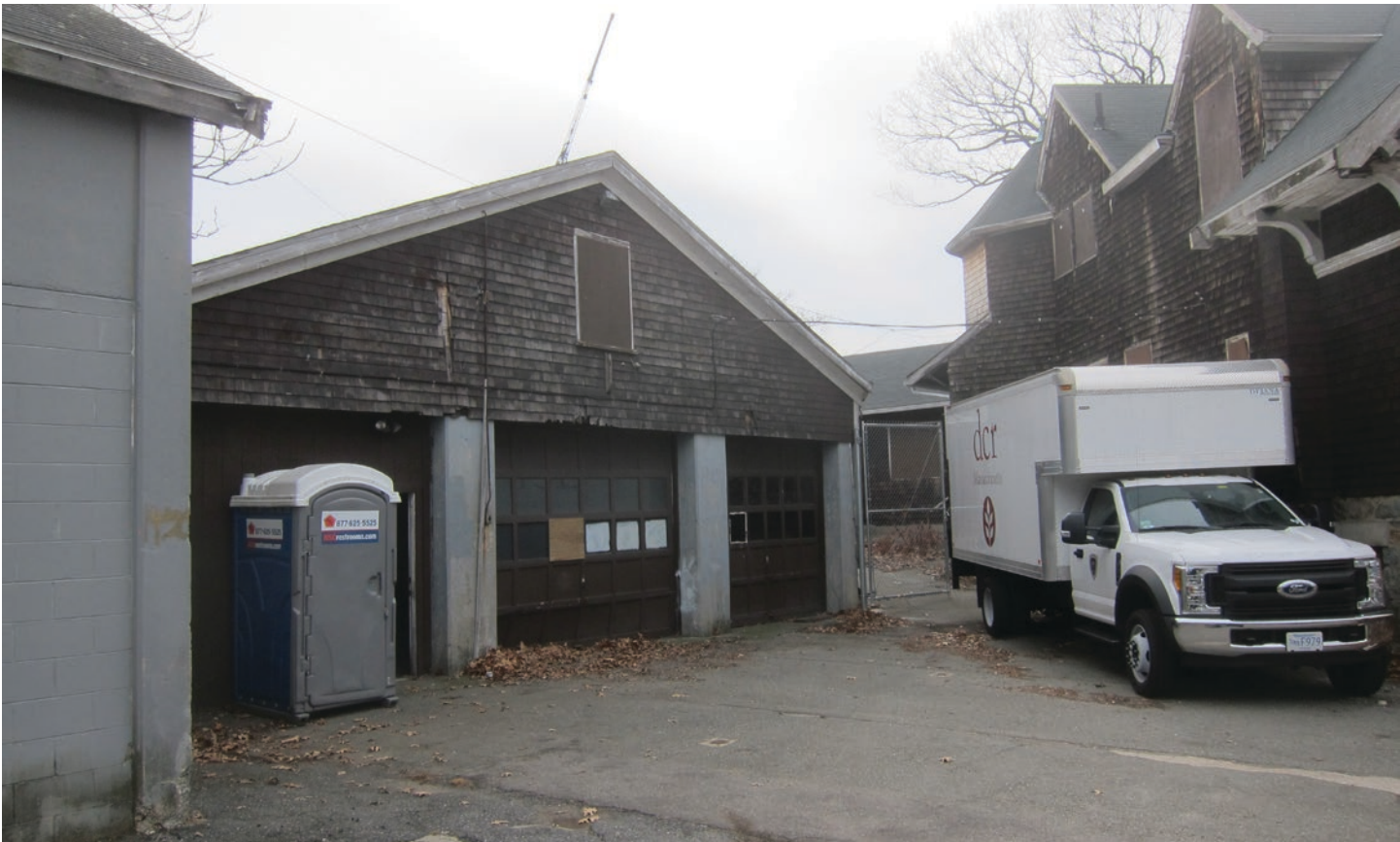
Figure 3: Building C Exterior
