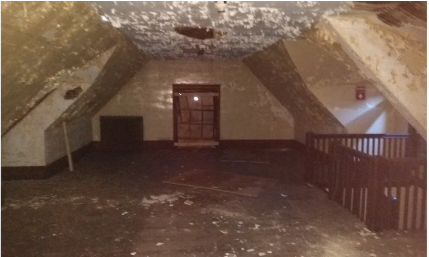
Figure 81: Building H Interior 2nd Floor
