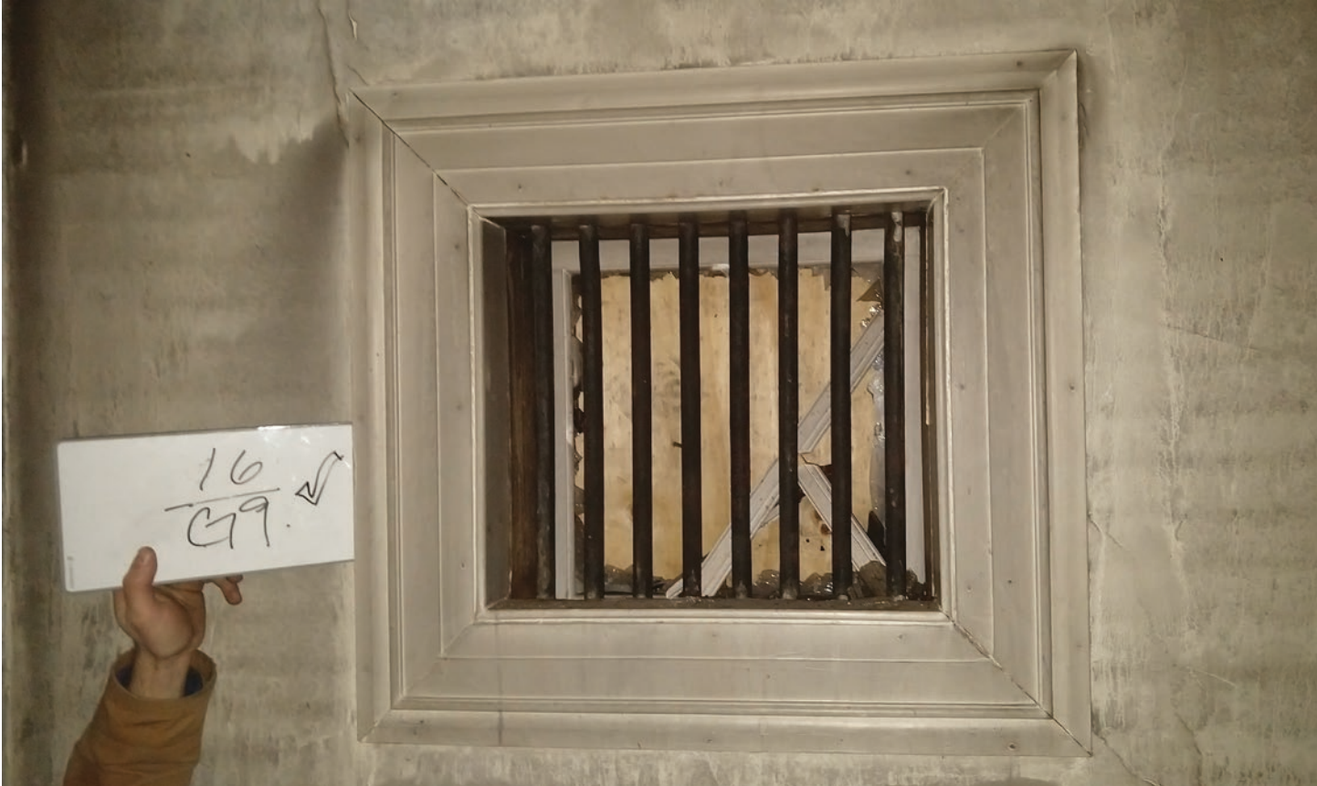
Figure 44: Building G Barred Window at Jail
