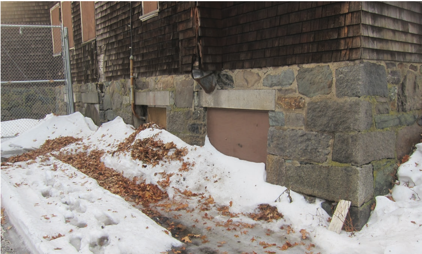
Figure 16: Building H Foundation with Lintels
