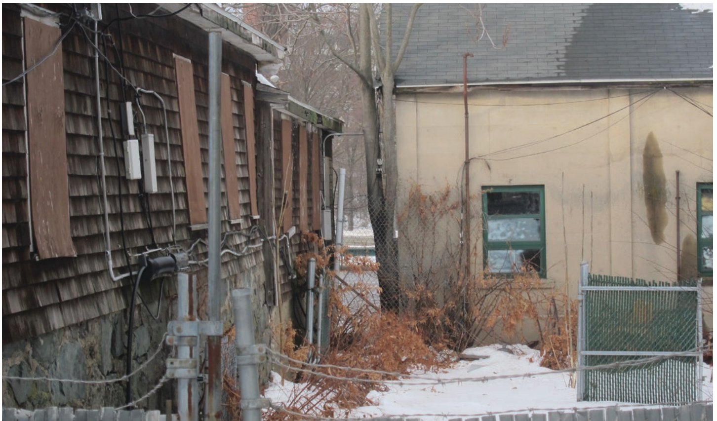
Figure 52: Building B Roof
