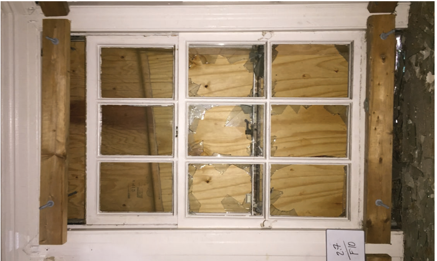
Figure 41: Building F Window
