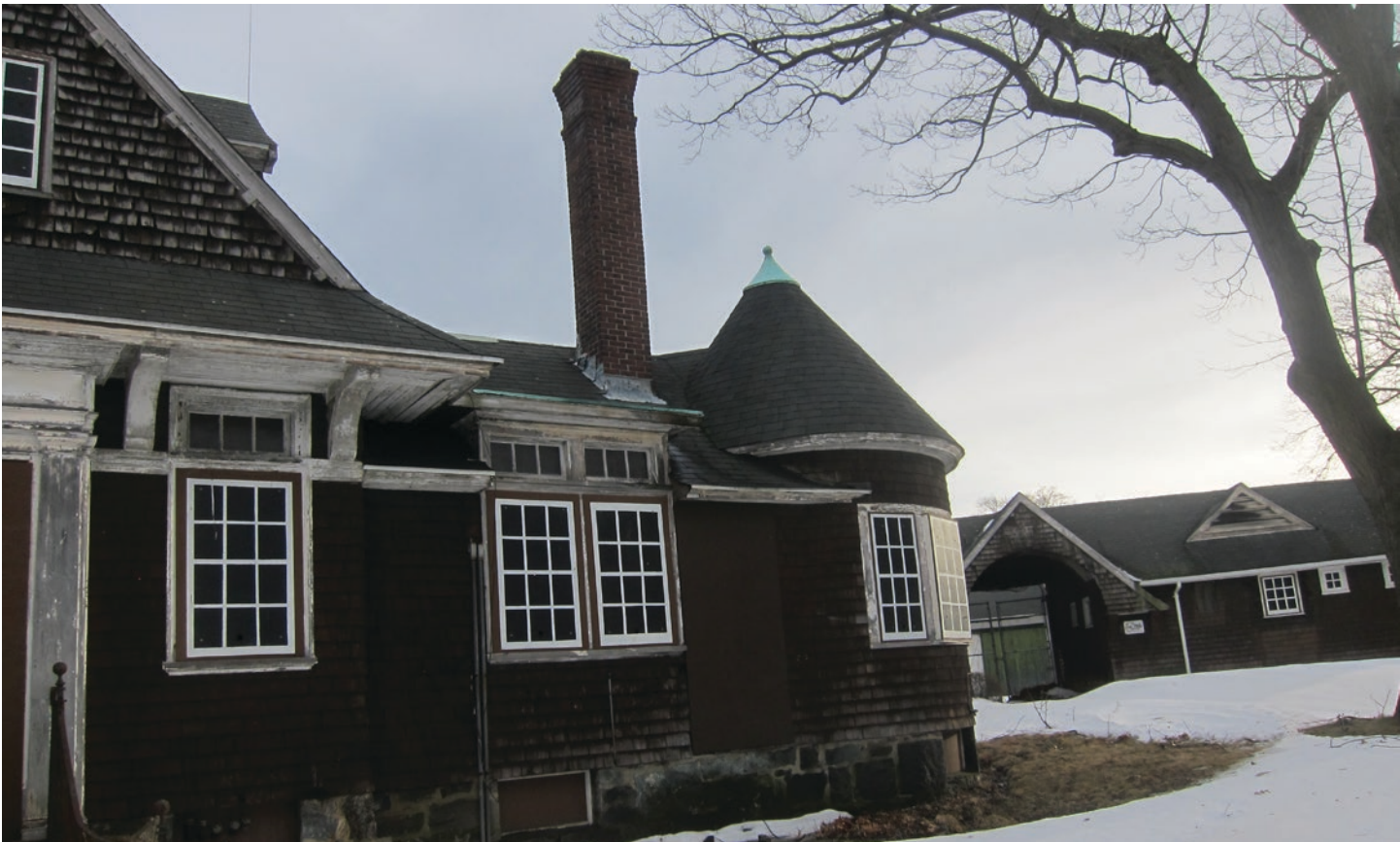
Figure 62: Building H Chimney
