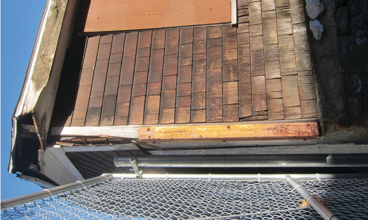
Figure 18: Building C Wood Trim
