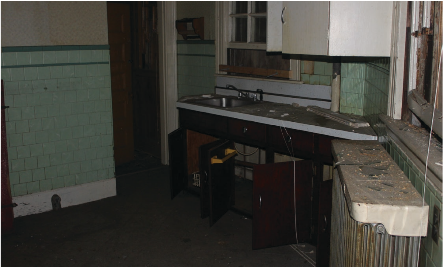
Figure 71: Building F Interior
