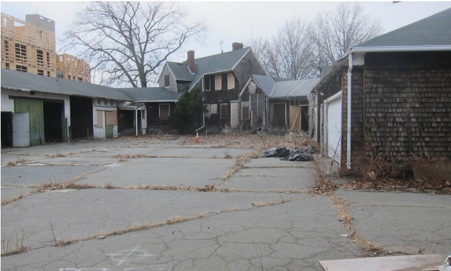
Figure 84: upper Courtyard Looking East
