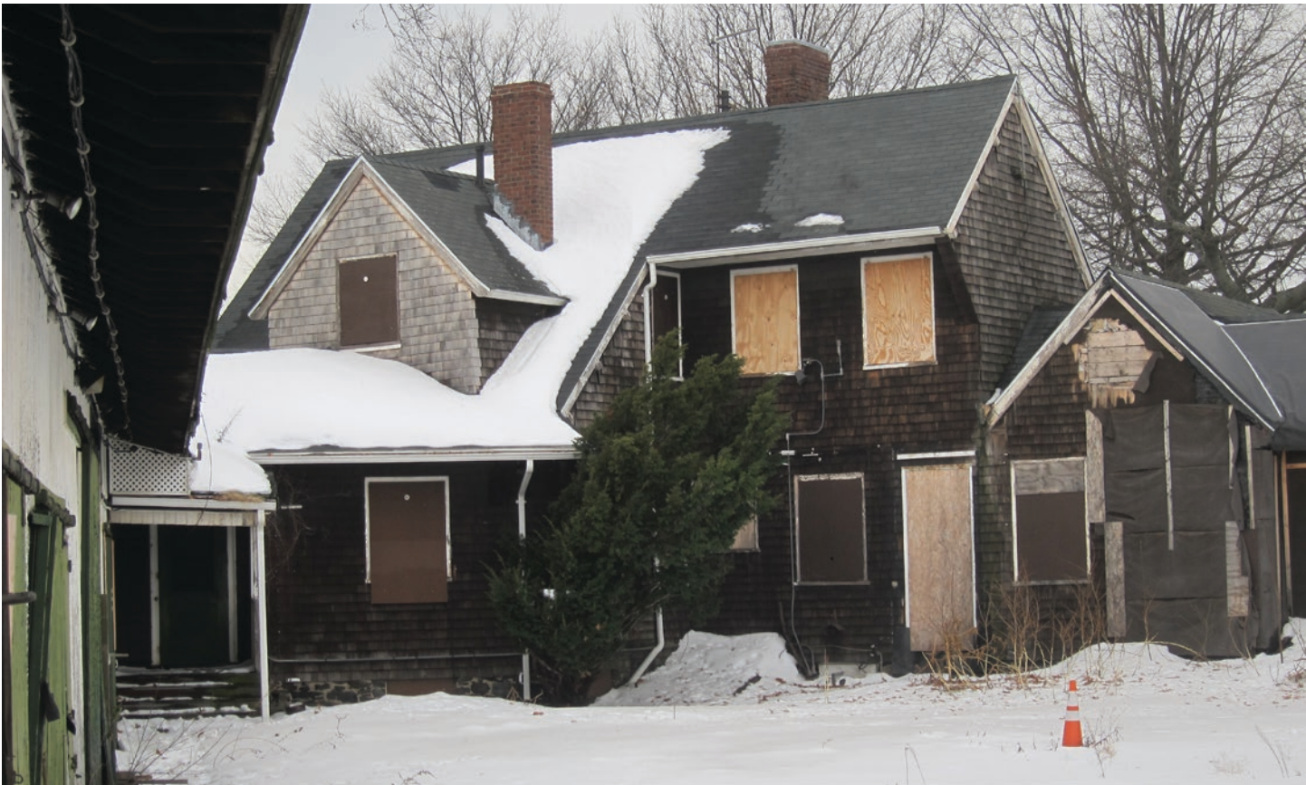
Figure 55: Building F Roof
