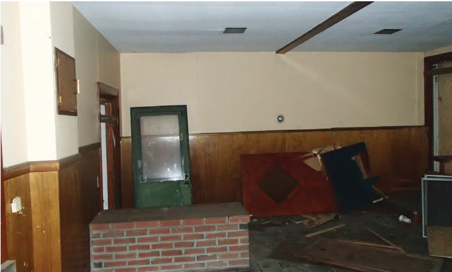
Figure 77: Building H Interior
