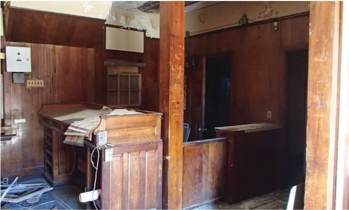
Figure 79: Building H Interior
