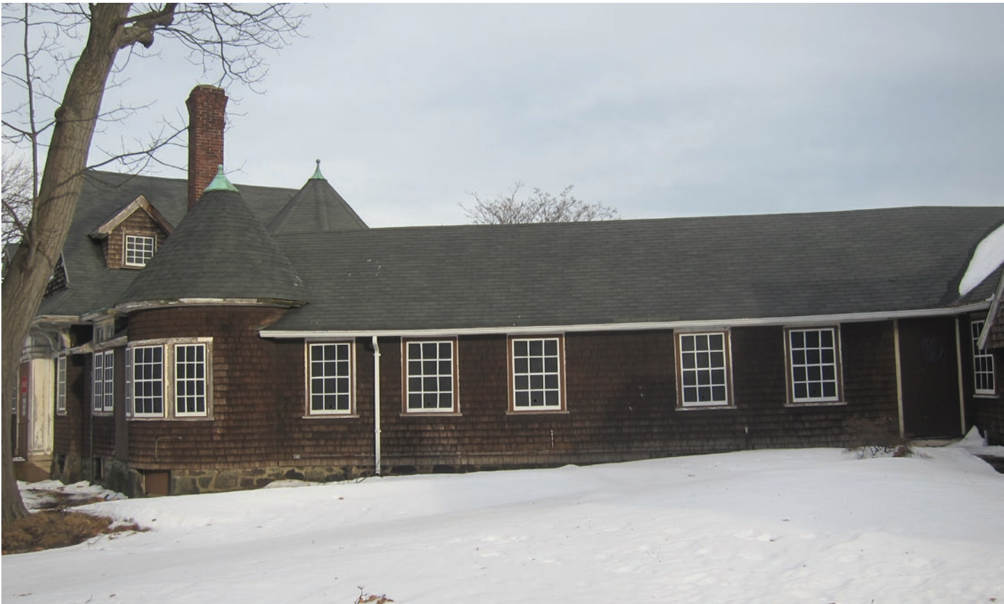
Figure 57: Building H Roof
