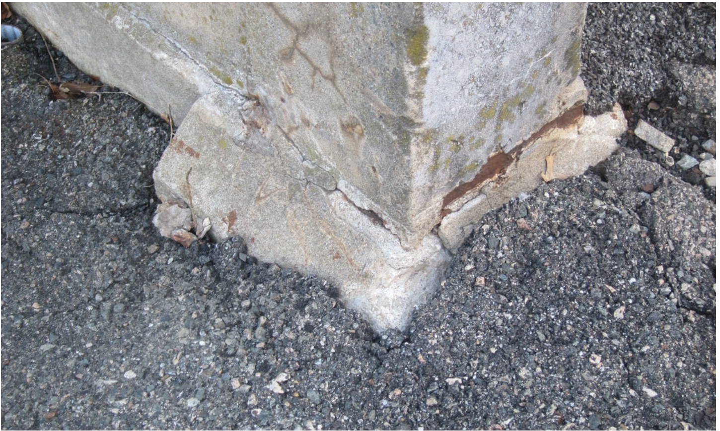
Figure 11: Building B Steel Column Baseplate
