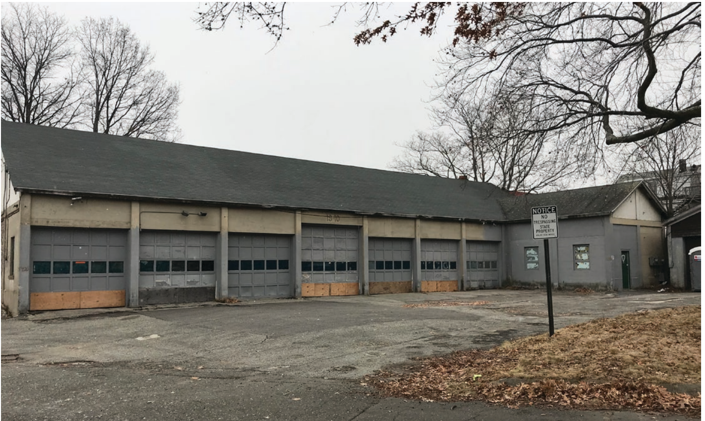
Figure 2: Building B Exterior
