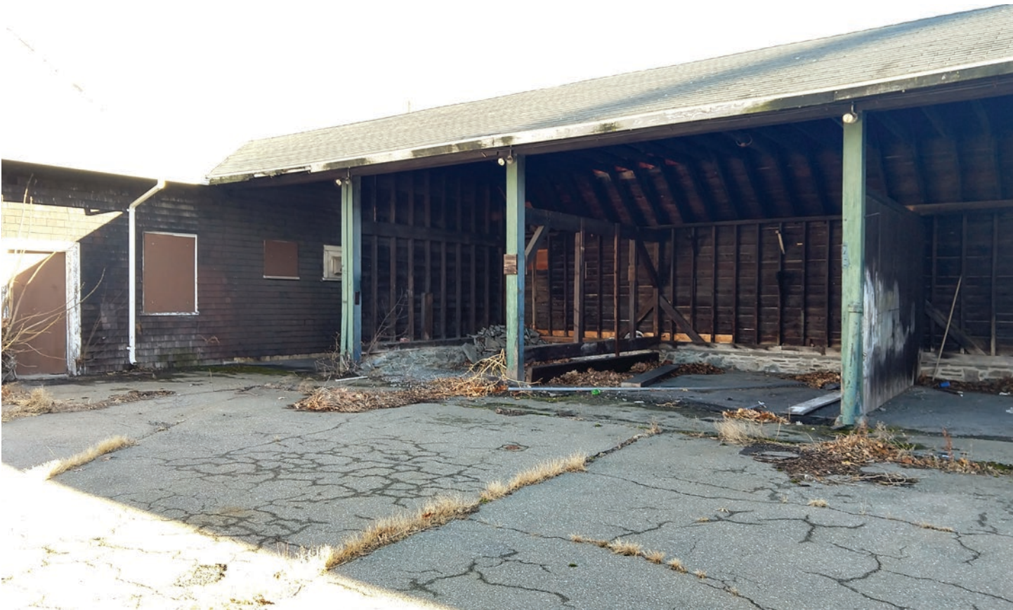
Figure 69: Building E Interior of Stable Bays
