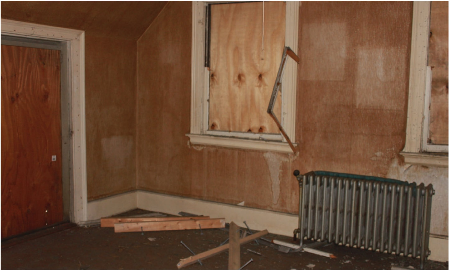
Figure 73: Building F Interior
