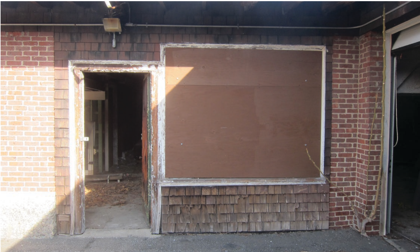
Figure 4: Building D Exterior
