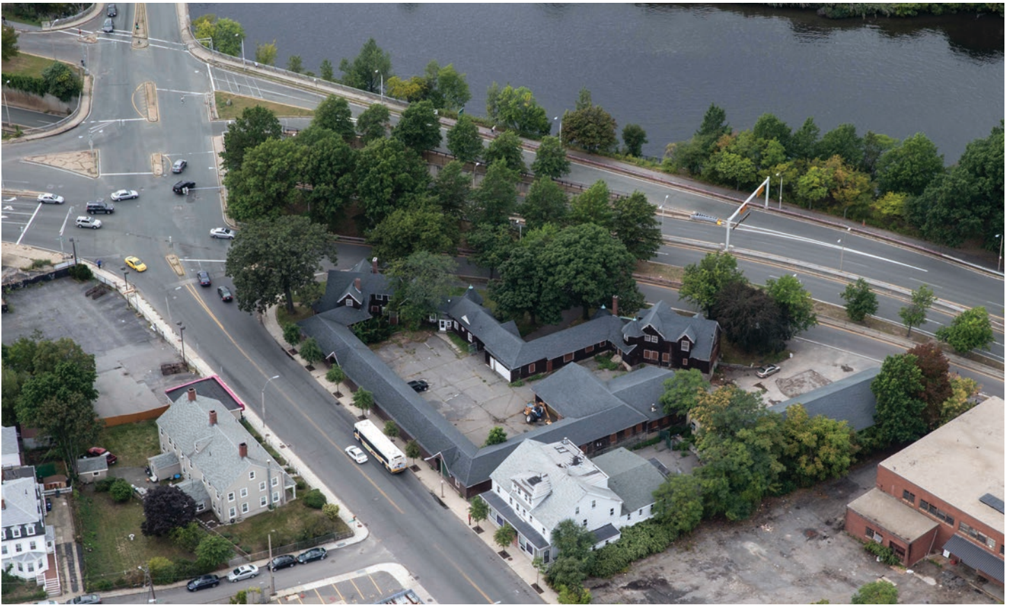
Figure 1: Aerial View of the Speedway cir. 2013
