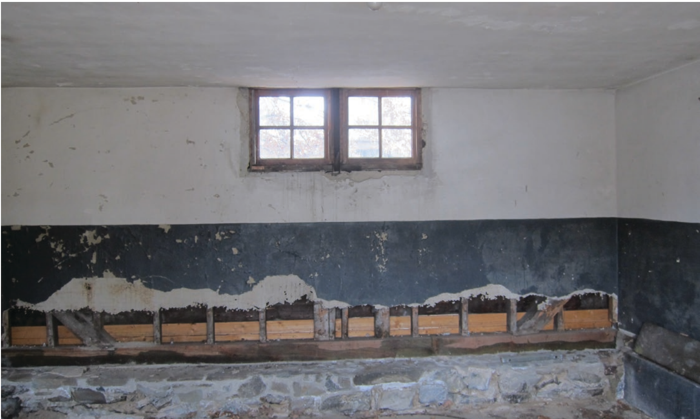
Figure 70: Building E Interior Enclosed Bay
