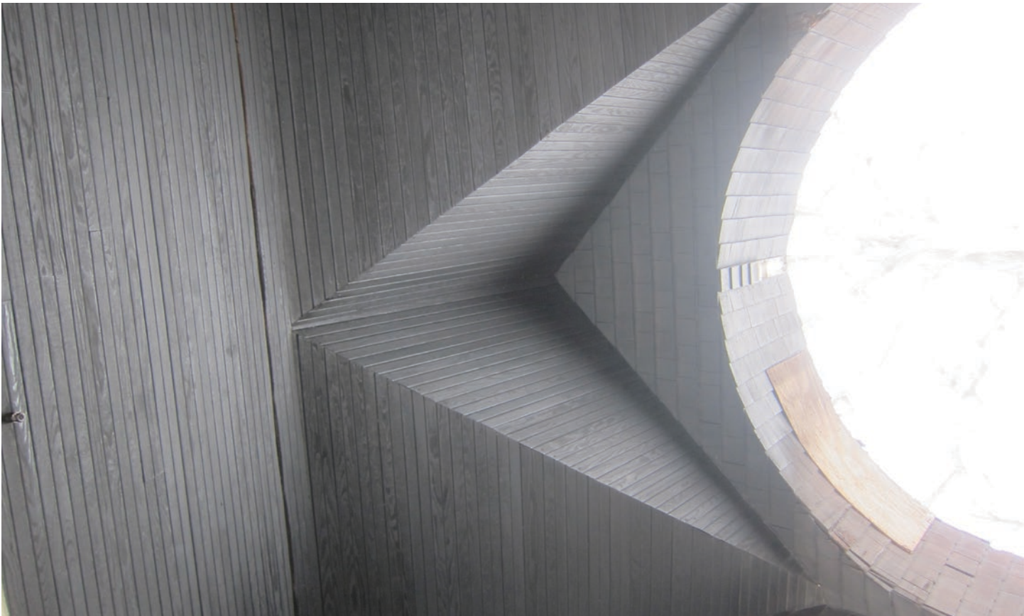
Figure 19: Building E Ceiling T&G
