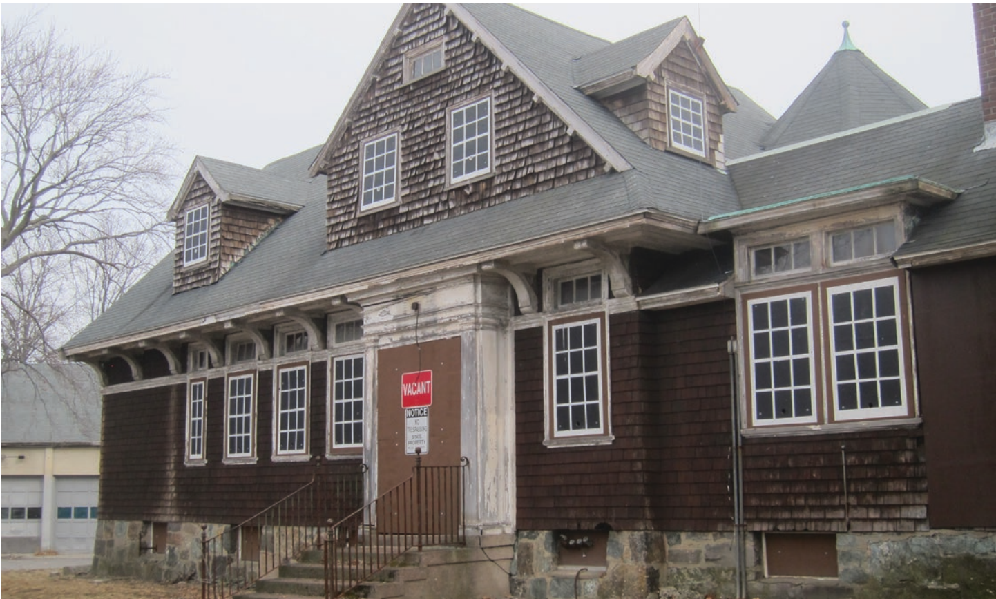
Figure 8: Building H Exterior
