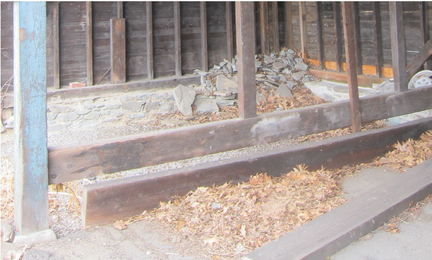
Figure 14: Building E Restored Foundation and Post Base
