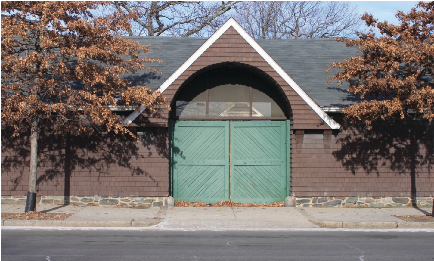
Figure 28: Building E Portal Door
