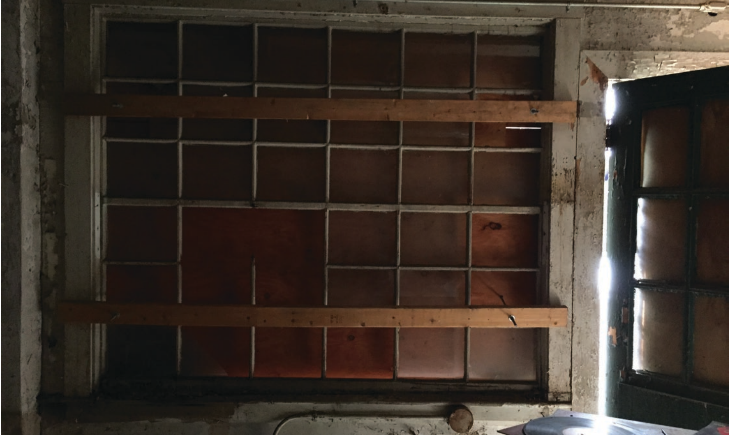
Figure 40: Building D Large Infill Window
