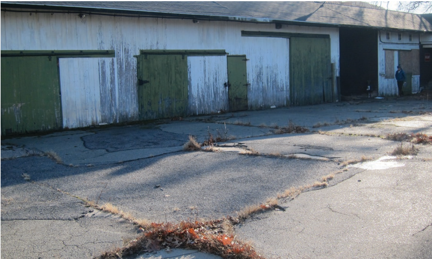
Figure 9: Building E Courtyard Exterior towards Building F
