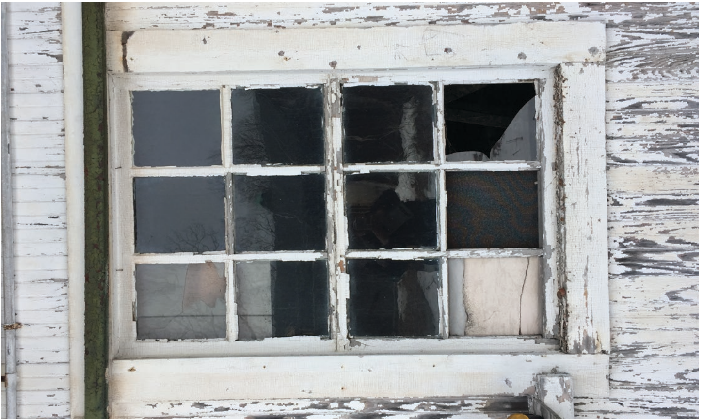
Figure 40: Building F Window at Sliding Courtyard Door
