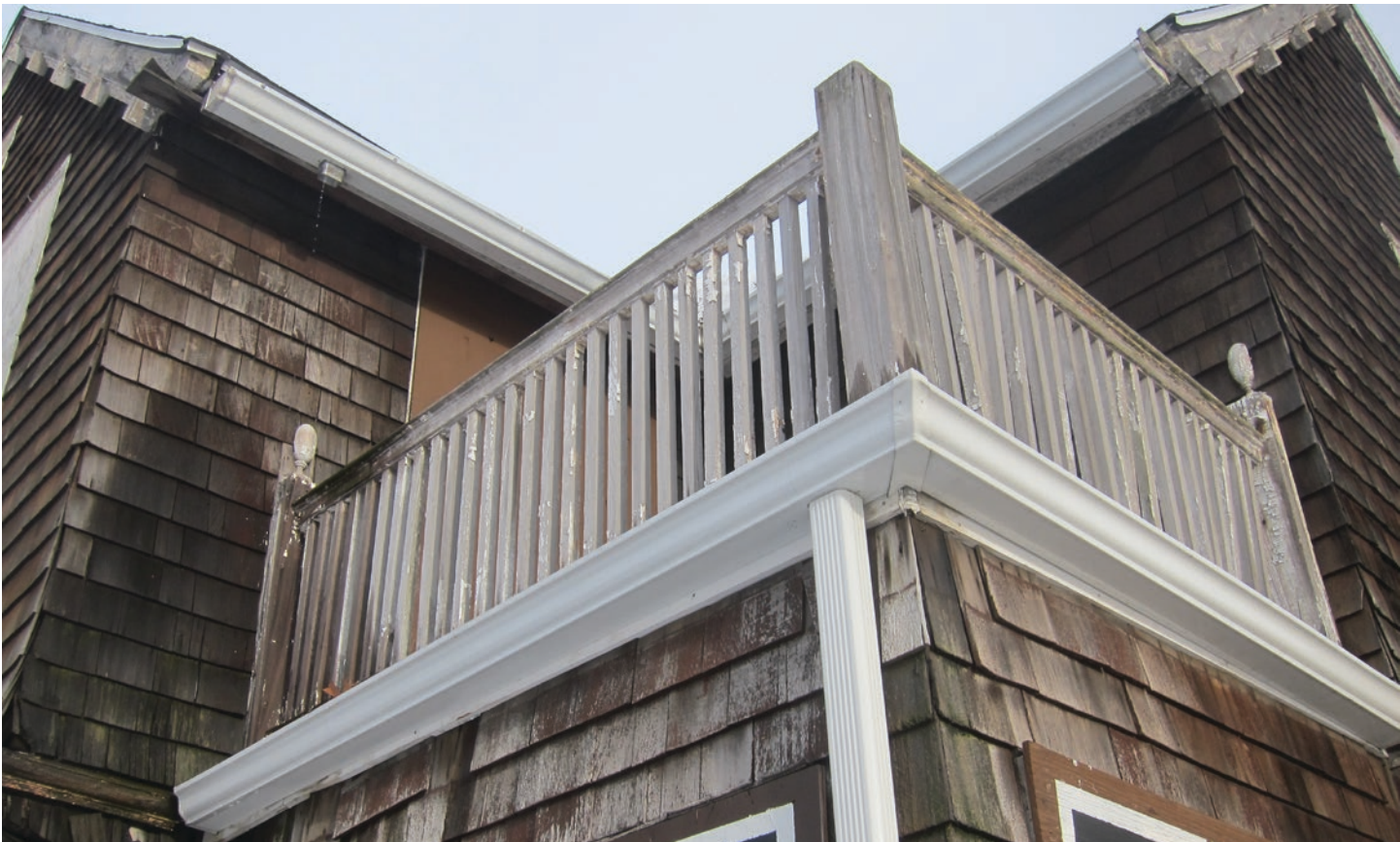
Figure 20: Building F 2nd Floor Porch and Eaves
