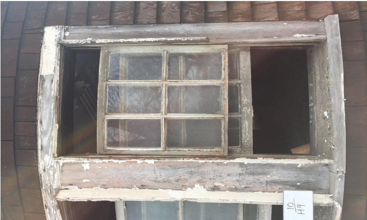
Figure 45: Building H Curved Sash
