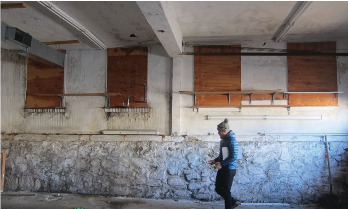
Figure 37: Building C Windows
