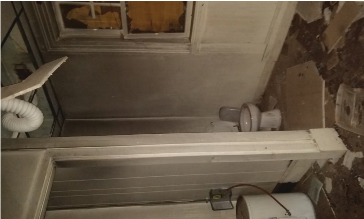
Figure 75: Building G Interior
