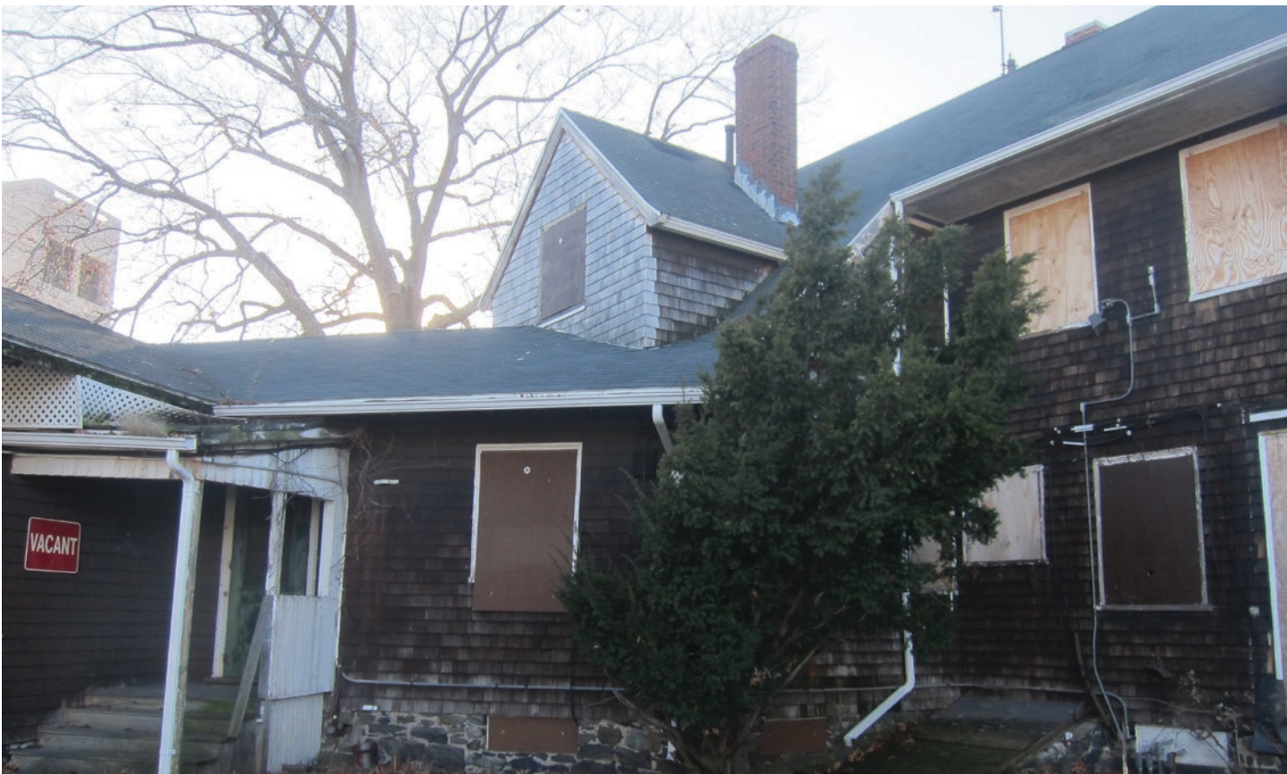
Figure 60: Building F Chimneys
