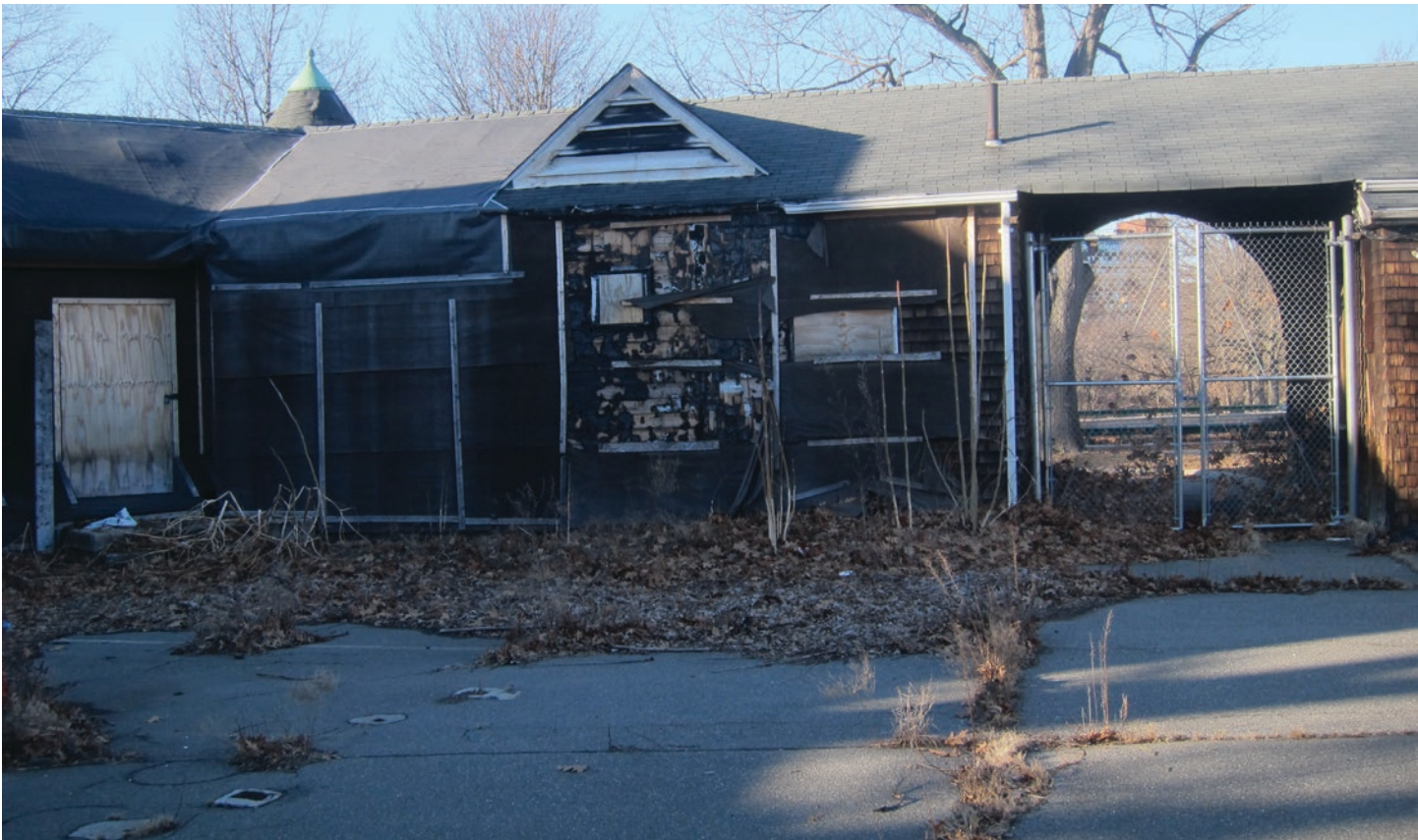
Figure 56: Building G Roof
