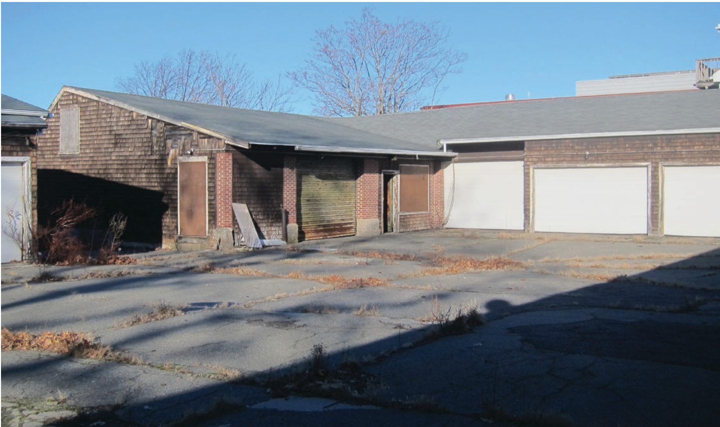
Figure 54: Building D Roof
