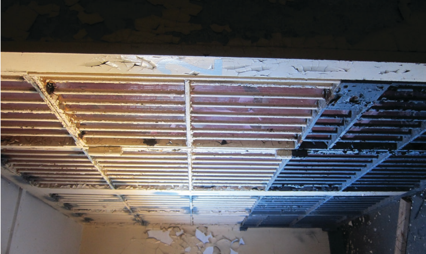
Figure 80: Building H Interior Jail Bars
