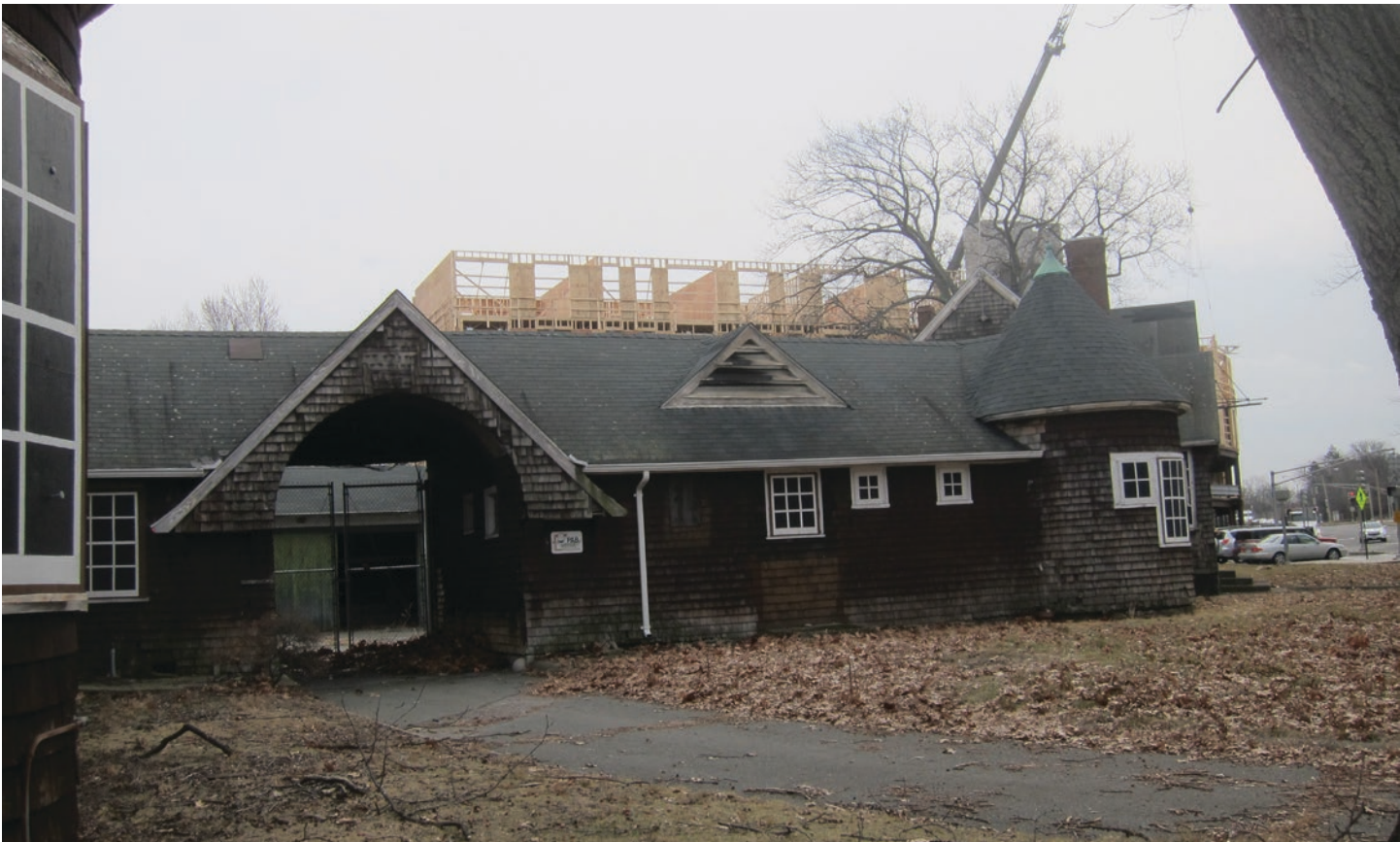
Figure 7: Building G Exterior
