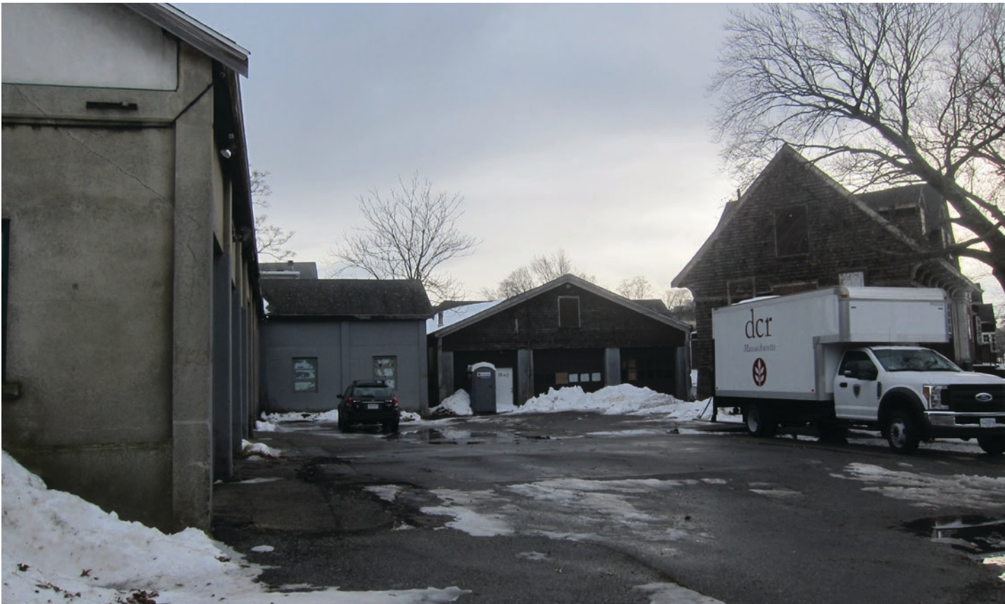
Figure 83: Lower service Courtyard
