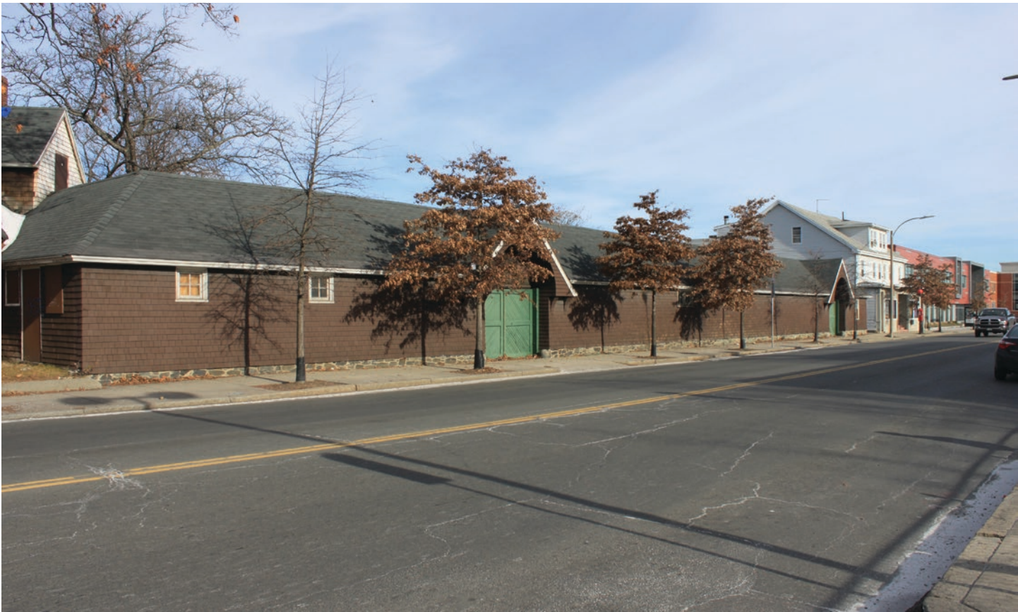
Figure 5: Building E Exterior
