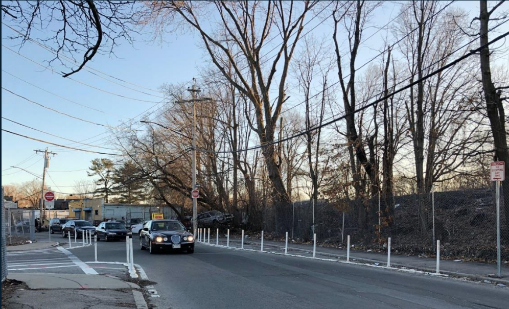
Parking restriction with paint and flex posts
