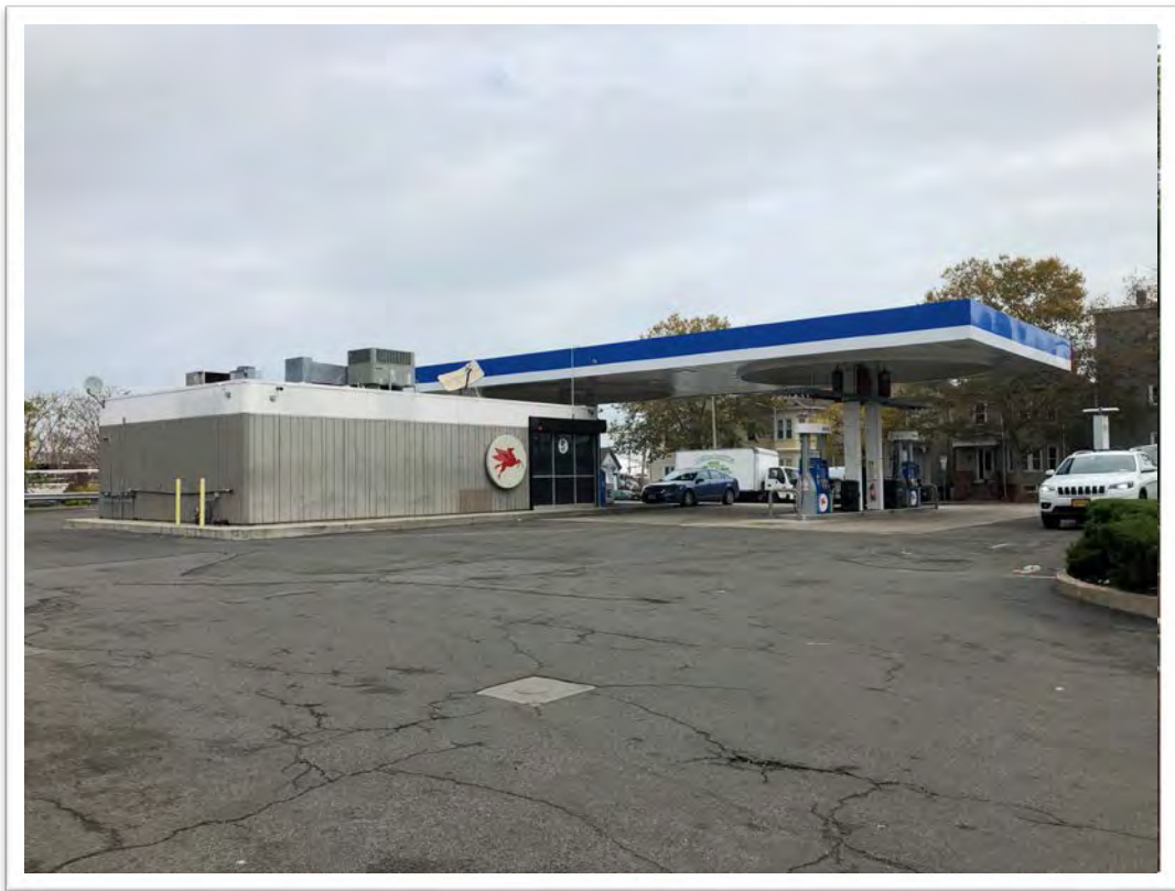
Photo 1: Representative photo of Mobil station, looking northeast.
