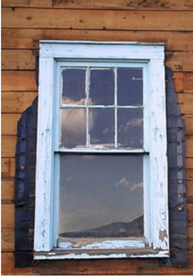
No evidence there is anything wrong with this window.
