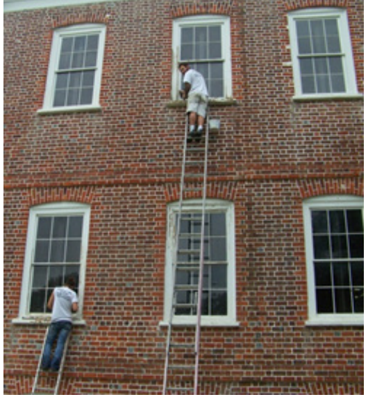
Which window is being replaced?
