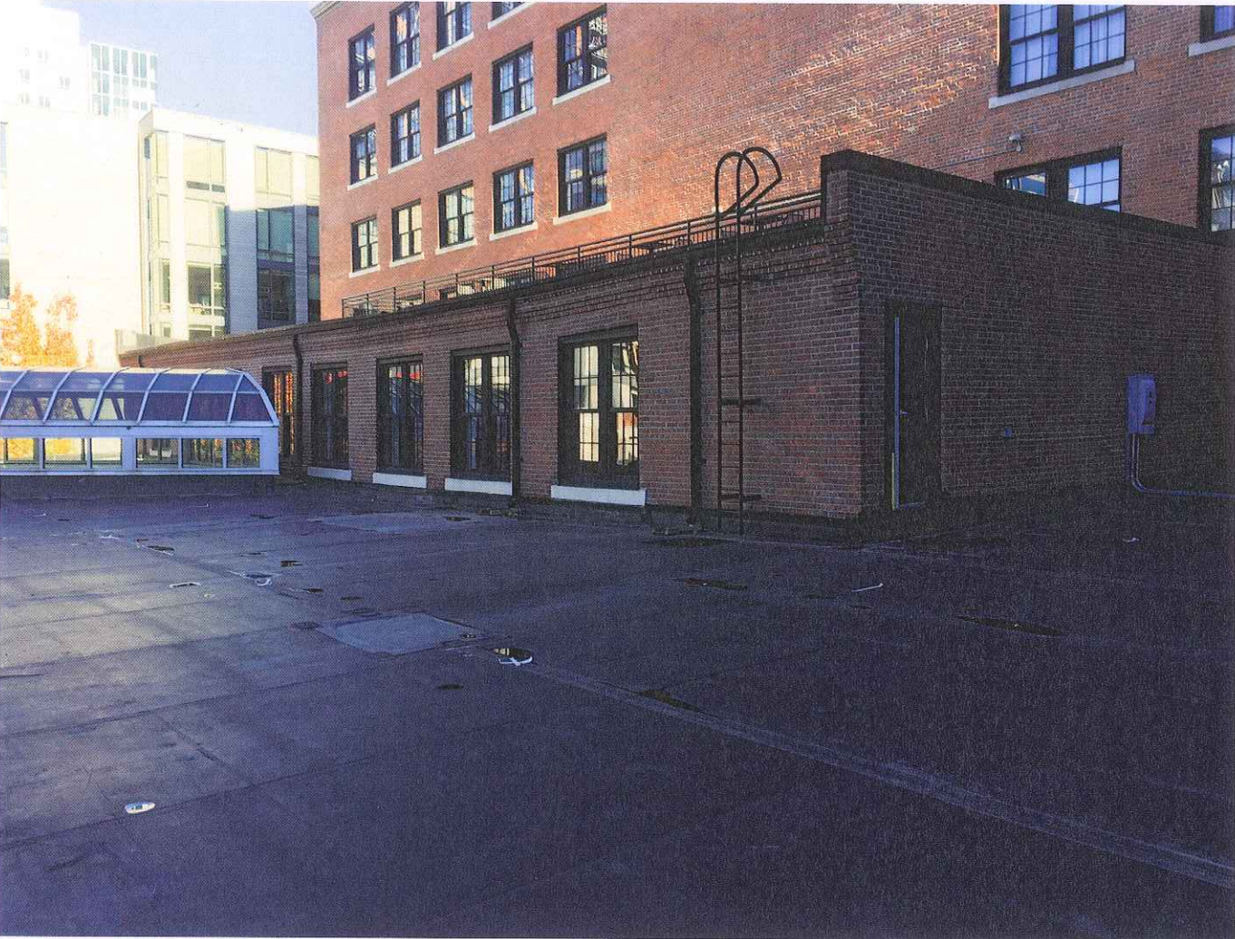
Existing Roof Conditions
