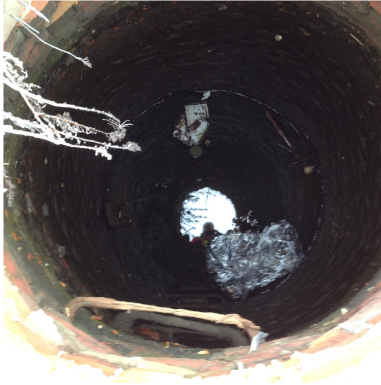
Figure 3-2. Looking inside Somerville Outfall H
