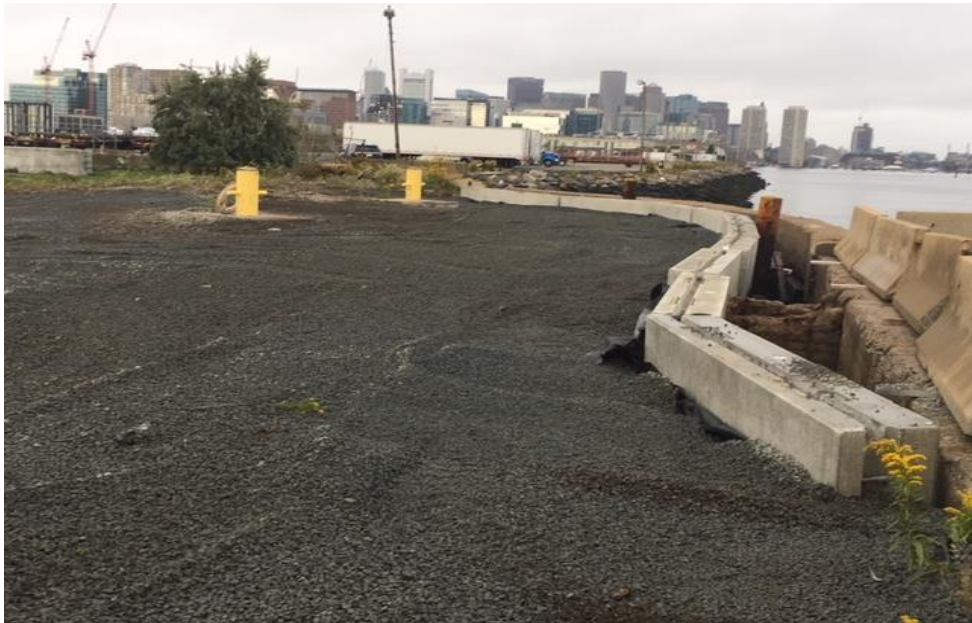
Photo 3: Stabilization of existing bollards
