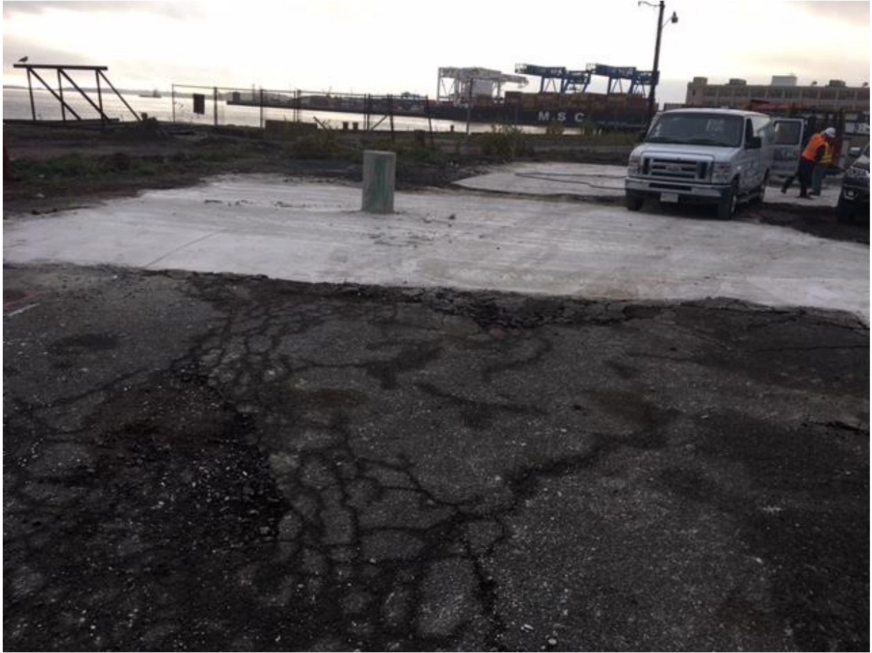
Photo 1: Installation of new bollards
