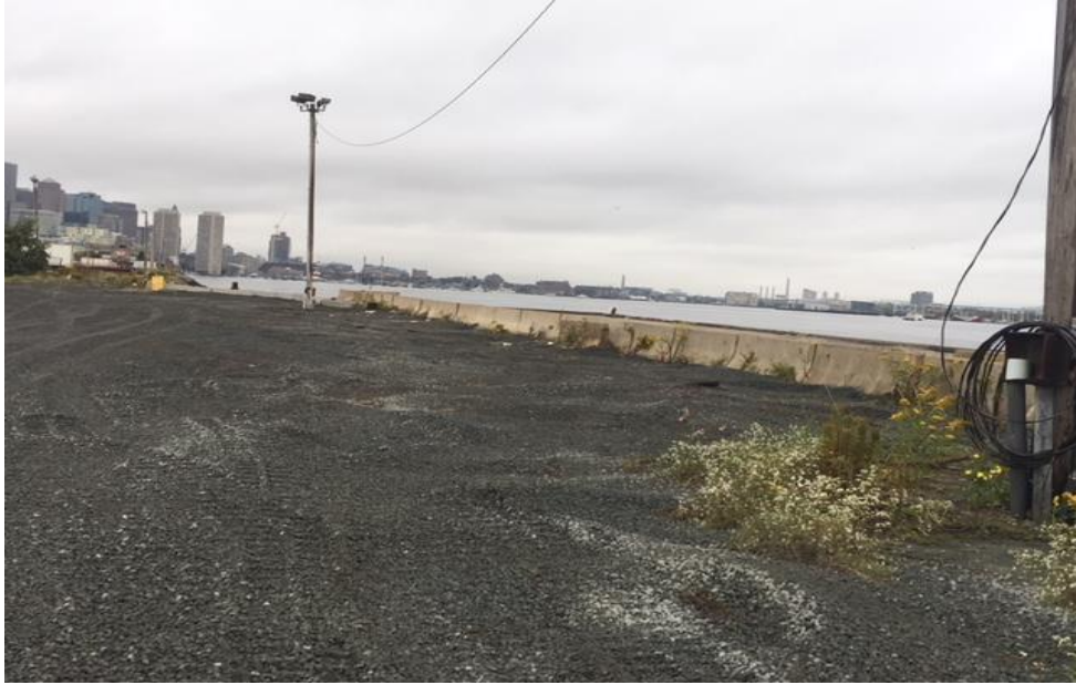
Photo 2: Area graded with crushed stone
