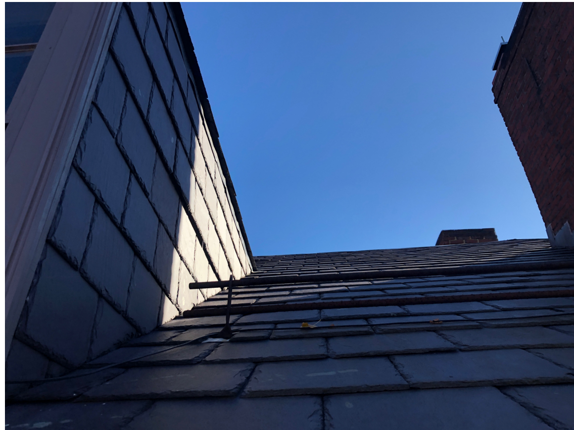
EXISTING SLATE ROOF AND SIDE WALL OF DORMER
