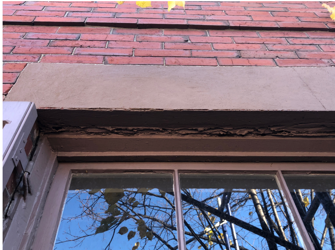
CRACKED LINTEL
