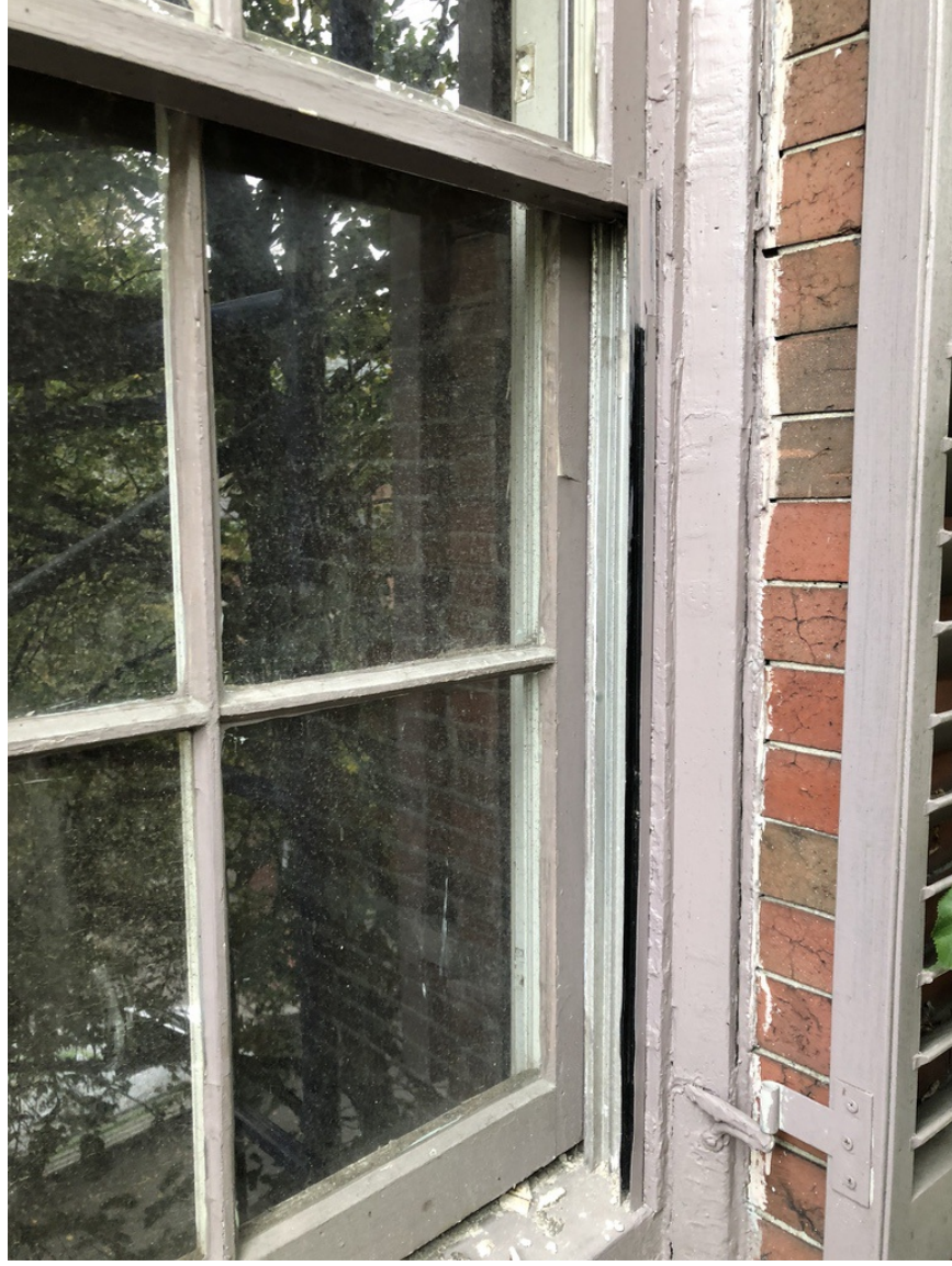
EXISTING DOUBLE HUNG WINDOWS (SASHES HAVE BEEN REPLACED)
