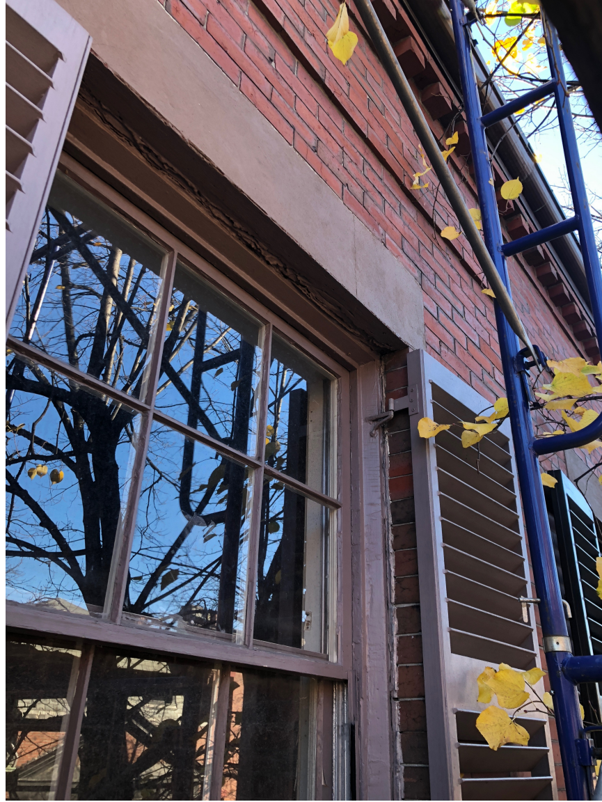
EXISTING WINDOW AND LINTEL
