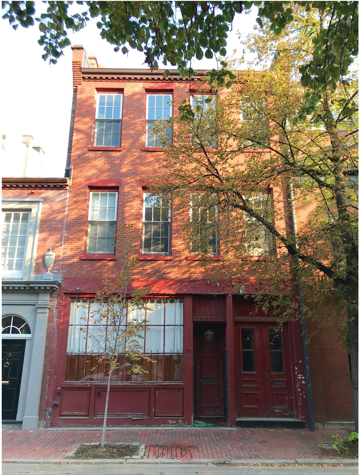
① EXISTING FRONT FACADE
