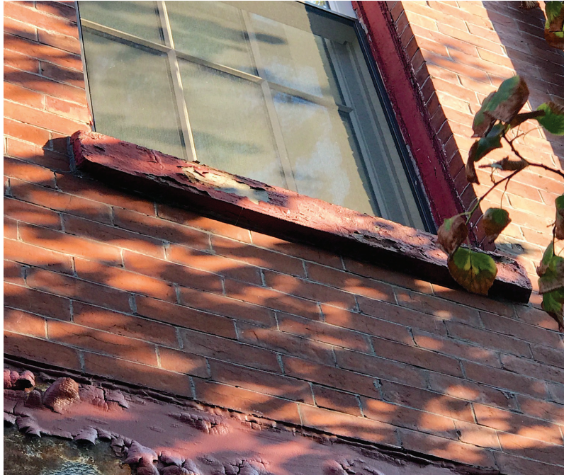
LINTEL & STEEL BEAM DETAIL
