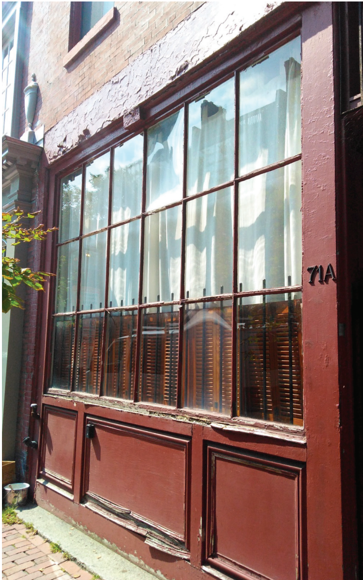
FIRST FLOOR FIXED WINDOW SASH & STEEL BEAM
