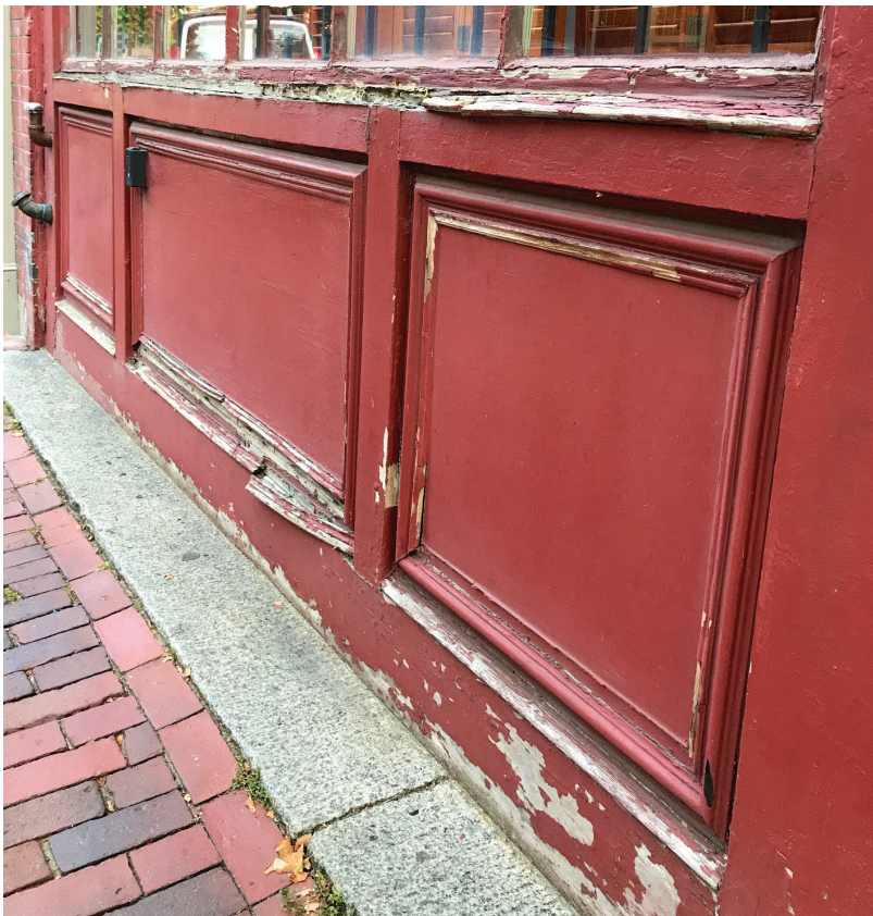
WOODWORK & EXTERIOR TRIM
