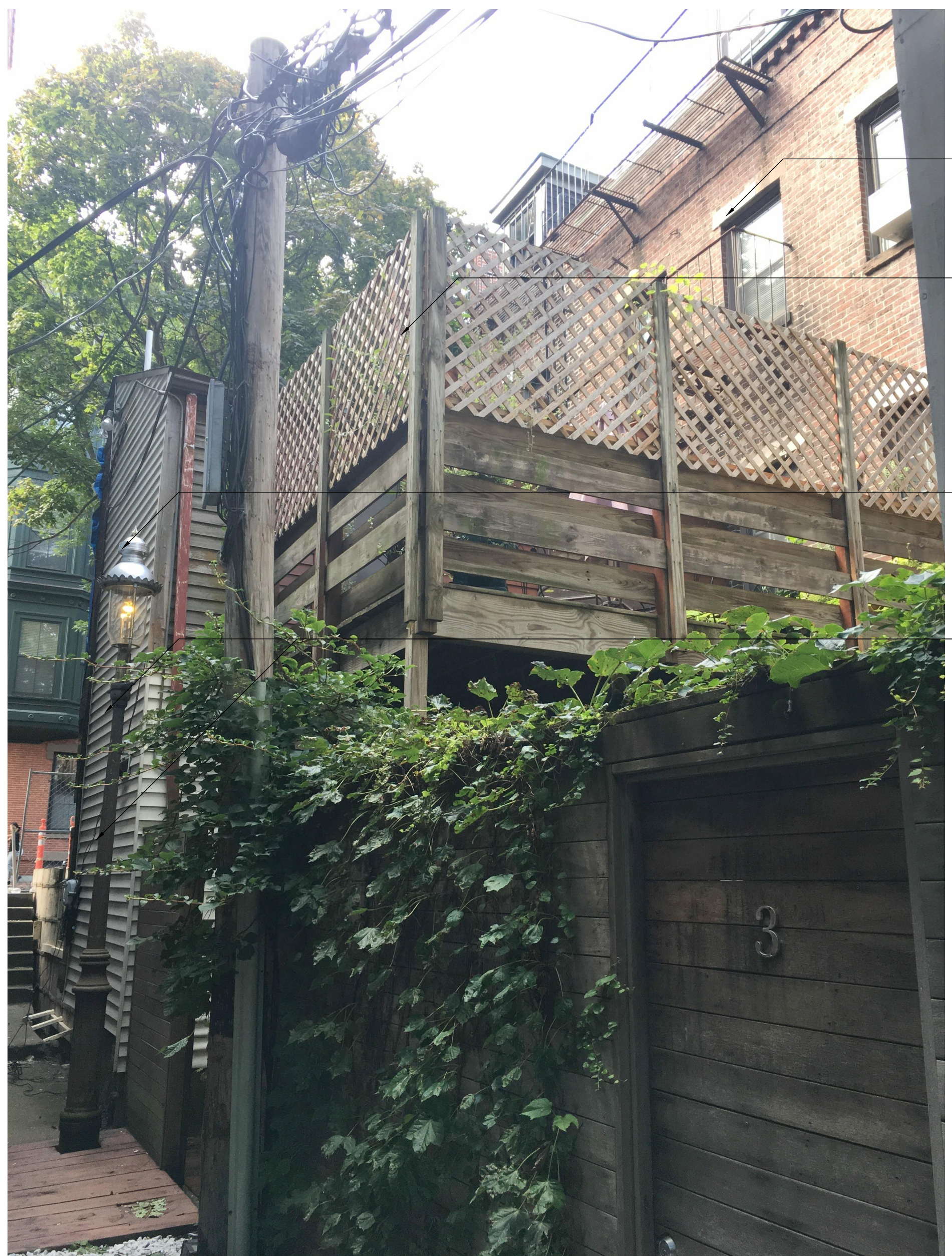
2 Existing Rear Facade Public Alley View
