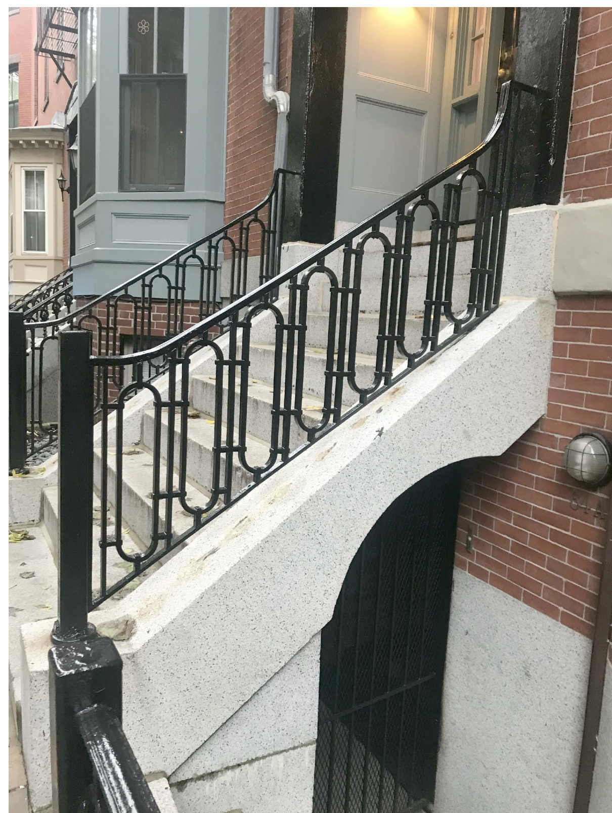
2 84 Waltham St. Boston, MA Front Stair and Railing Precedent Image
