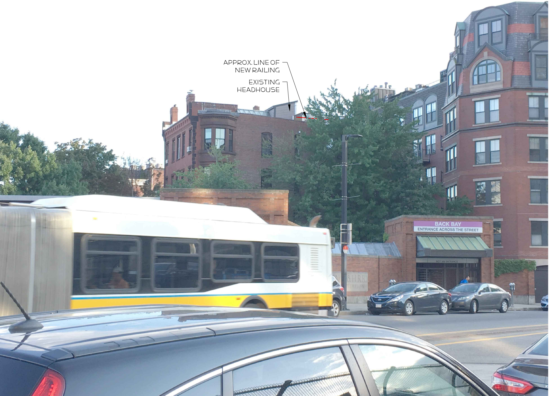
VIEW FROM OPPOSITE SIDE OF COLUMBUS AVENUE
