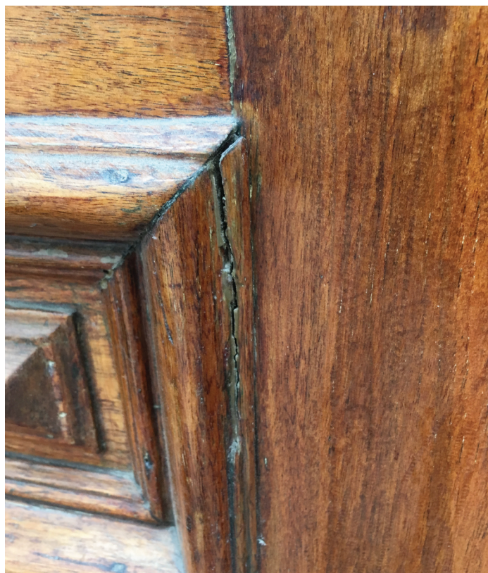
fractured molding
