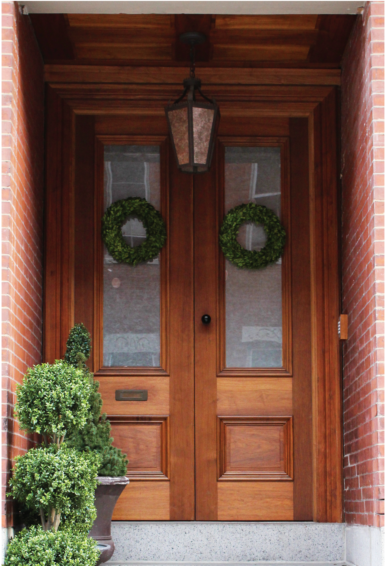
Newly made doors in American black walnut
