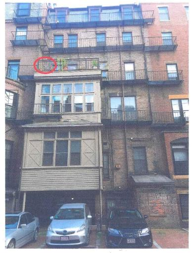
Location – on the third floor deck on the alley side of the building, where the old one has been since it was installed in 1993. Minimally visible from the street, tucked in the corner. Due to the construction of mini-splits, the condenser has to be very close to the same height as the units inside, so this unit has to be installed between the second and fourth floors. The third floor location (where it has been for 25 years) is optimal, and in addition is almost invisible from the street.
