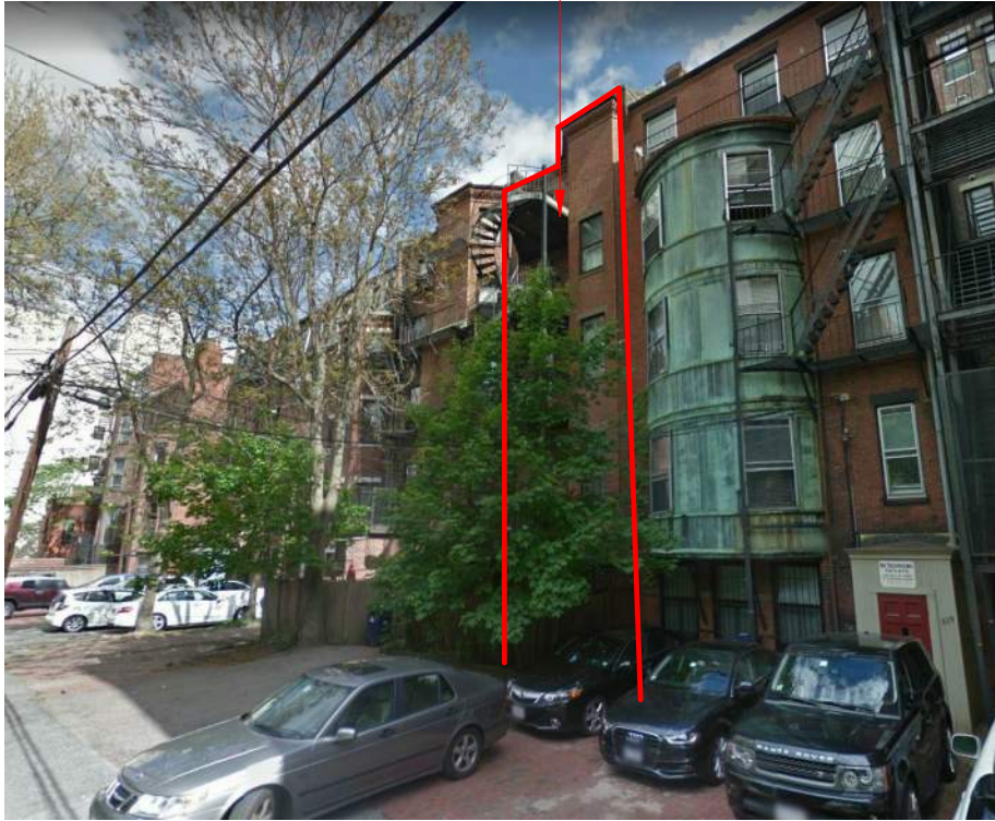
PUBLIC ALLEY 429 LOOKING EAST
