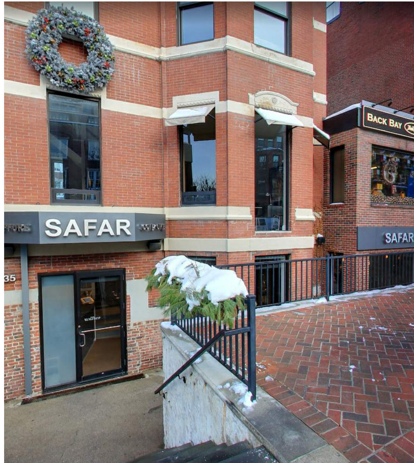
EXISTING BAY CONDITION #1 (UPPER PORTION)
