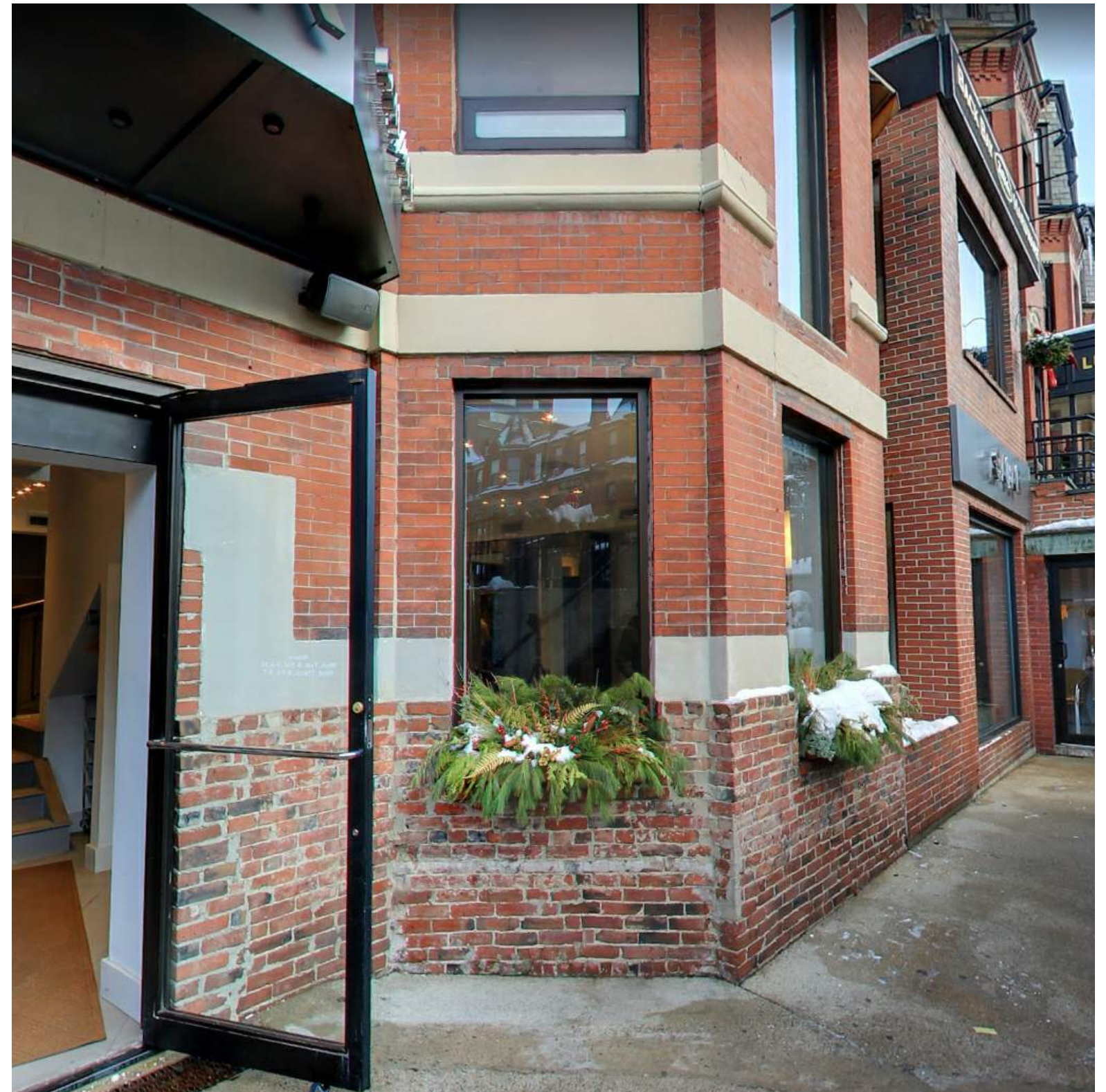
EXISTING BAY CONDITION #2 (LOWER PORTION)
