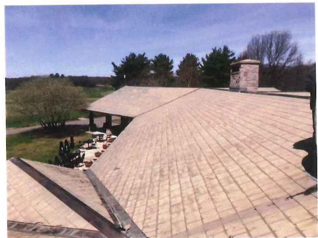
Partial view of roof
