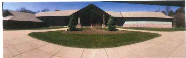
View of the north east elevation.
