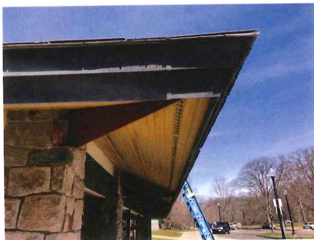
Typical roof overhang and vented soffit.
