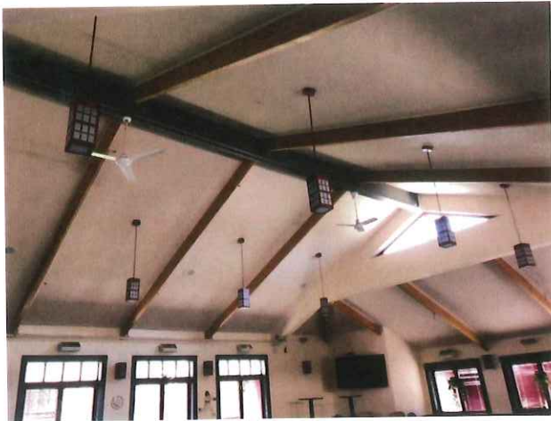
View of the typical roof construction from the interior vaulted ceiling.
