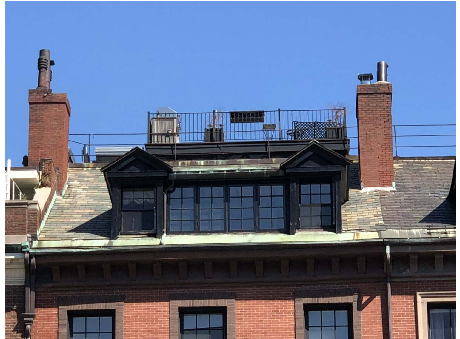
ZOOM-IN VIEW OF THE ROOF DECK FROM THE BOSTON PUBLIC GARDEN PHOTO TAKEN IN 2018
