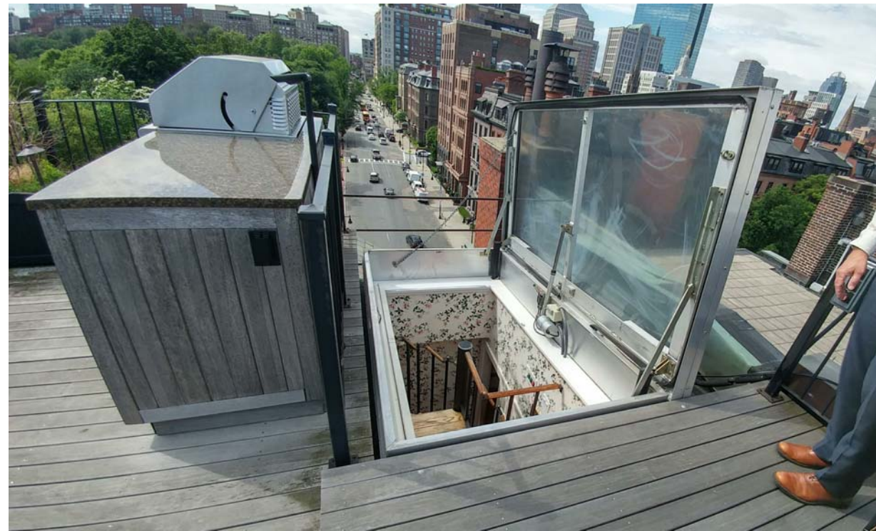
EXISTING SPIRAL STAIRS & ROOF HATCH
