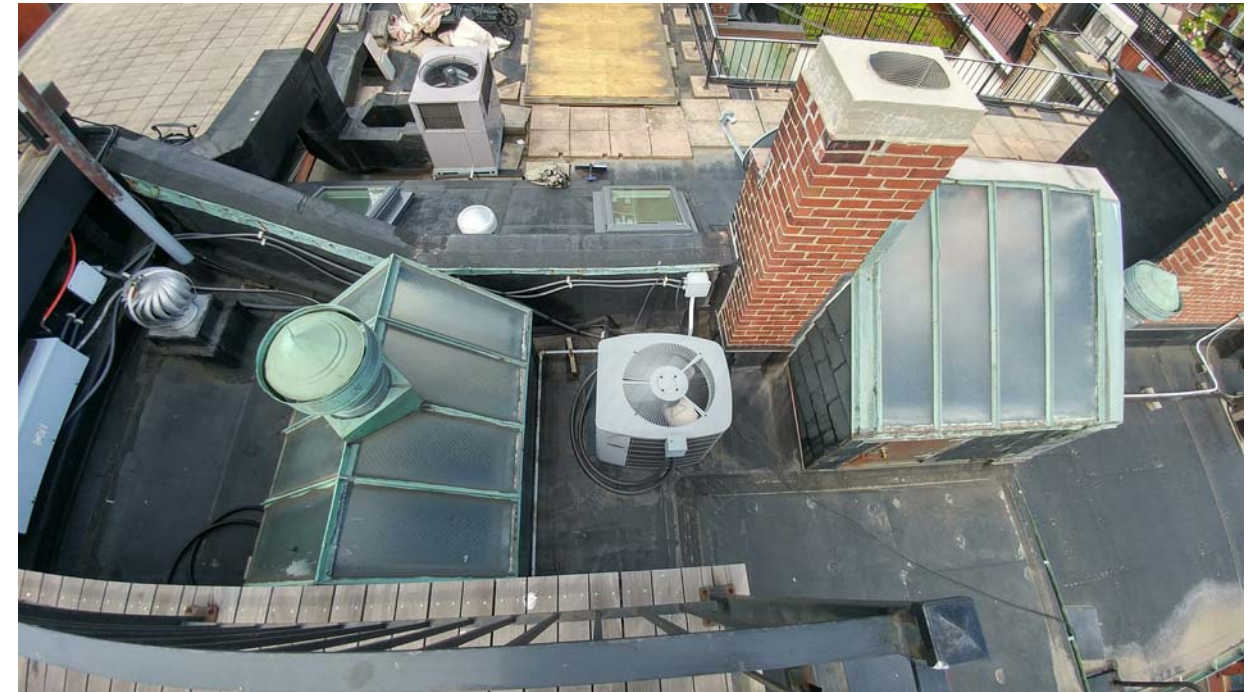
EXISTING WEST SIDE OF THE ROOFTOP
