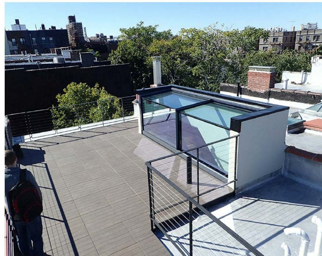
PROPOSED STAIR HATCH - GLASS BOX-TYPE SLIDING HATCH
