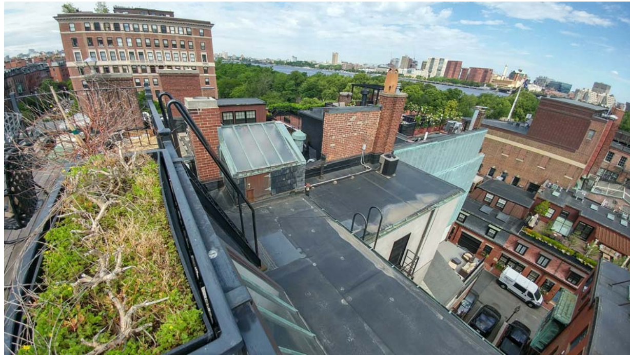
EXISTING ROOFTOP VIEW TO BEAVER PL.
