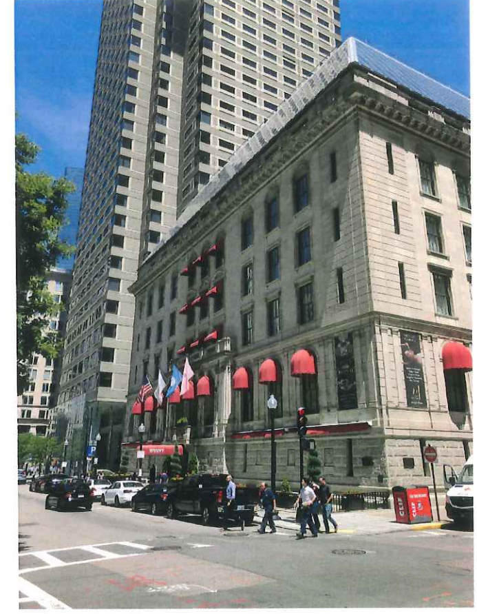
PEARL STREET FACADE
