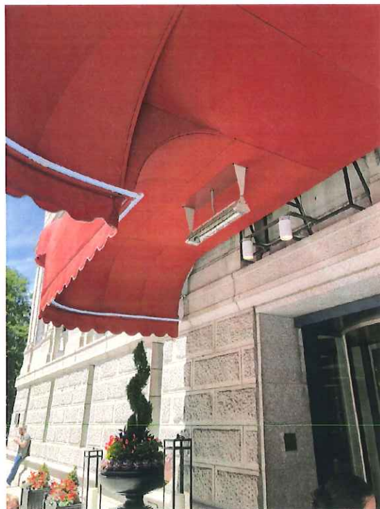
EXISTING CANOPY - UNDERSIDE
