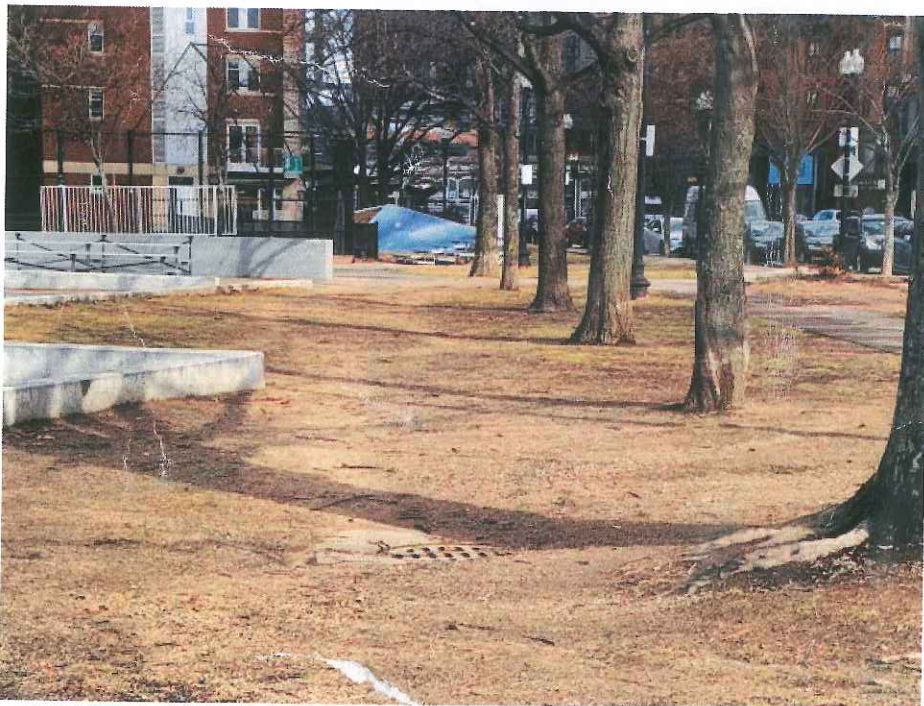
Washington Street: Repair storm drainage system in this area. Install new bituminous path along courts. Regrade lawn slightly to improve drainage and reseed.
