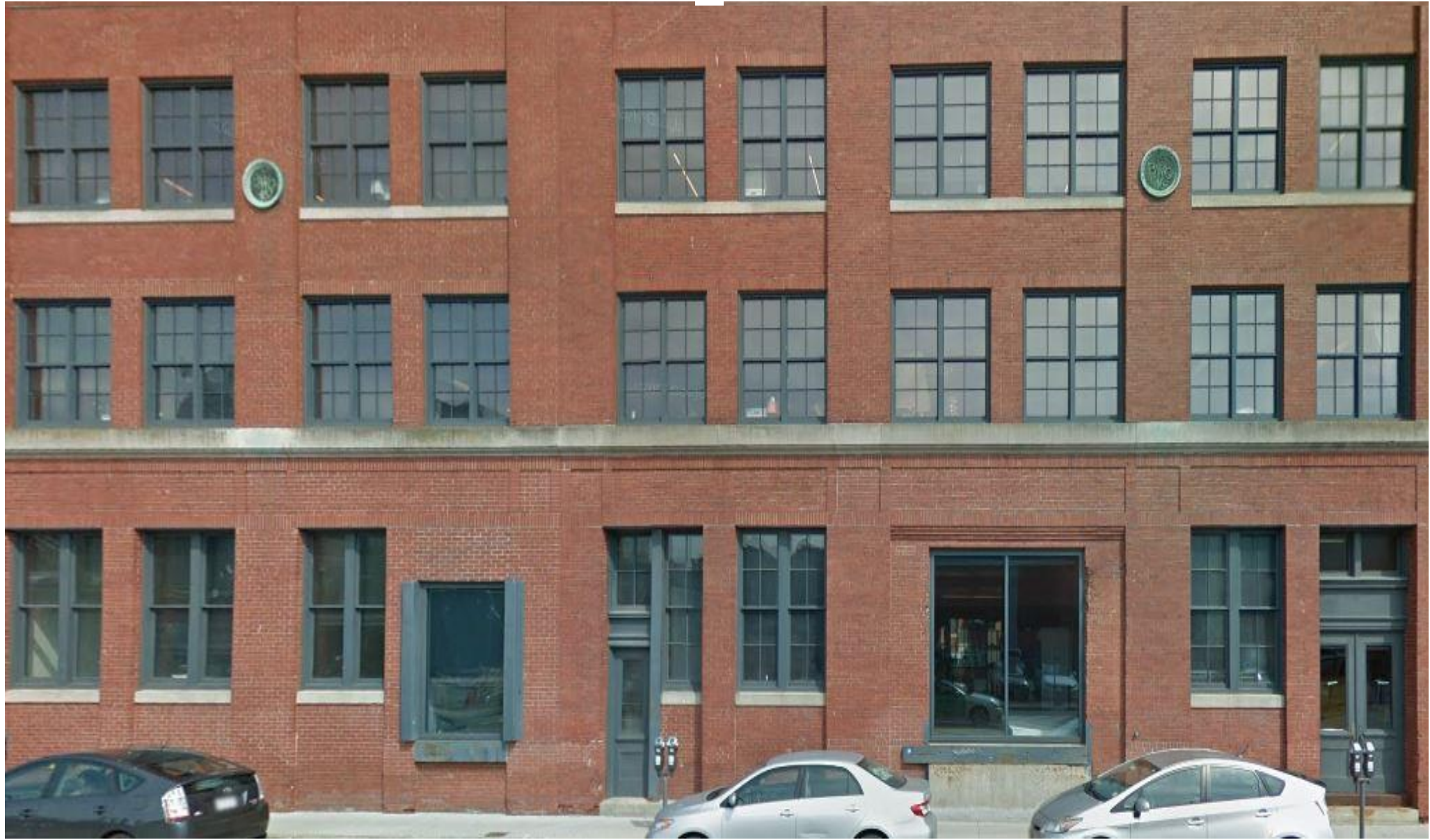
MIDDLE OF CHANNEL CENTER BLOCK
