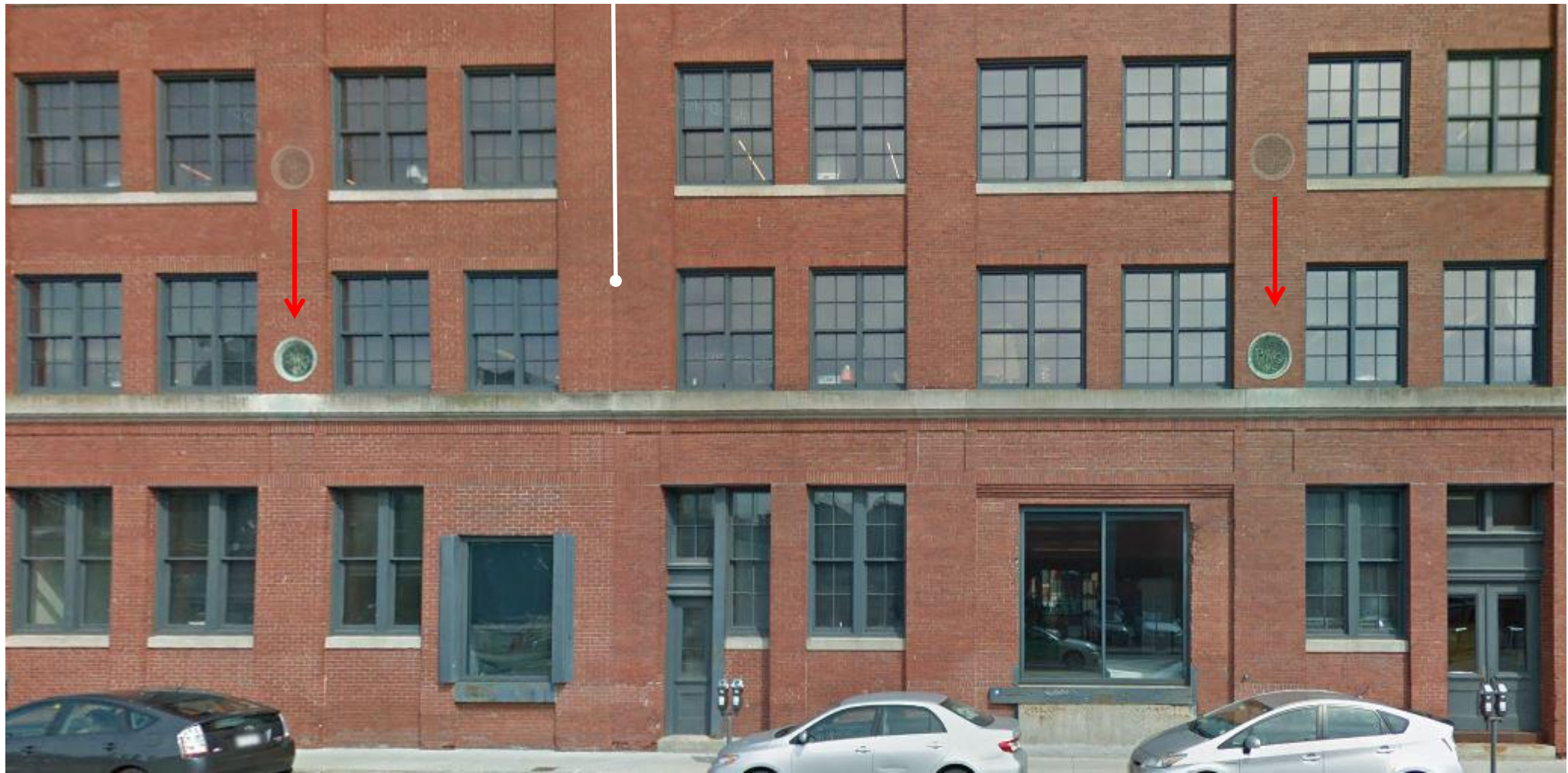
MIDDLE OF CHANNEL CENTER BLOCK
