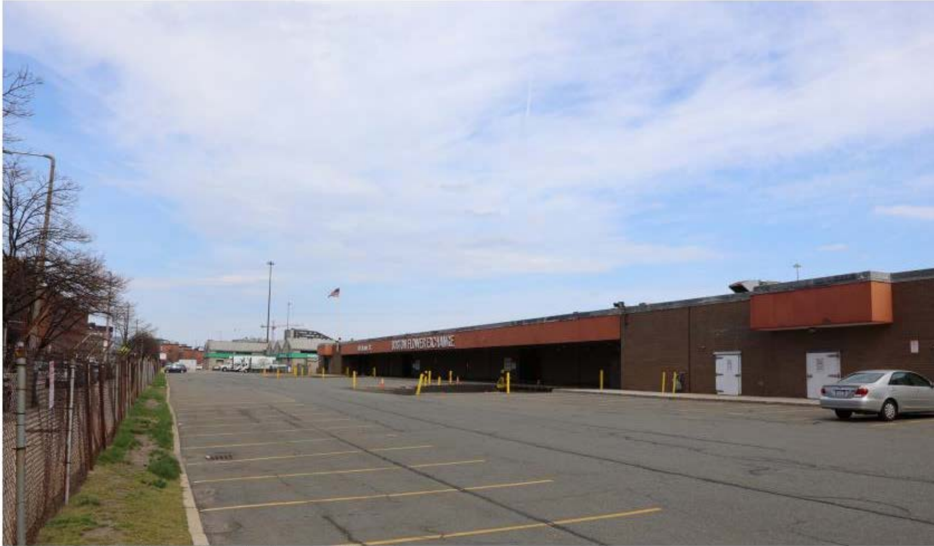
Photograph 1: View of site looking northeast
