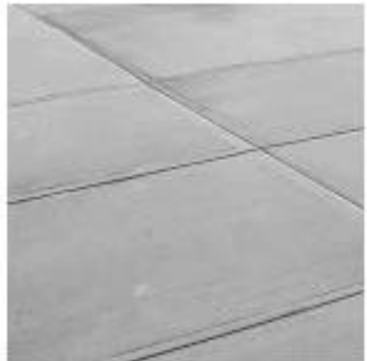
5. Cast-in-Place Concrete Pavement
