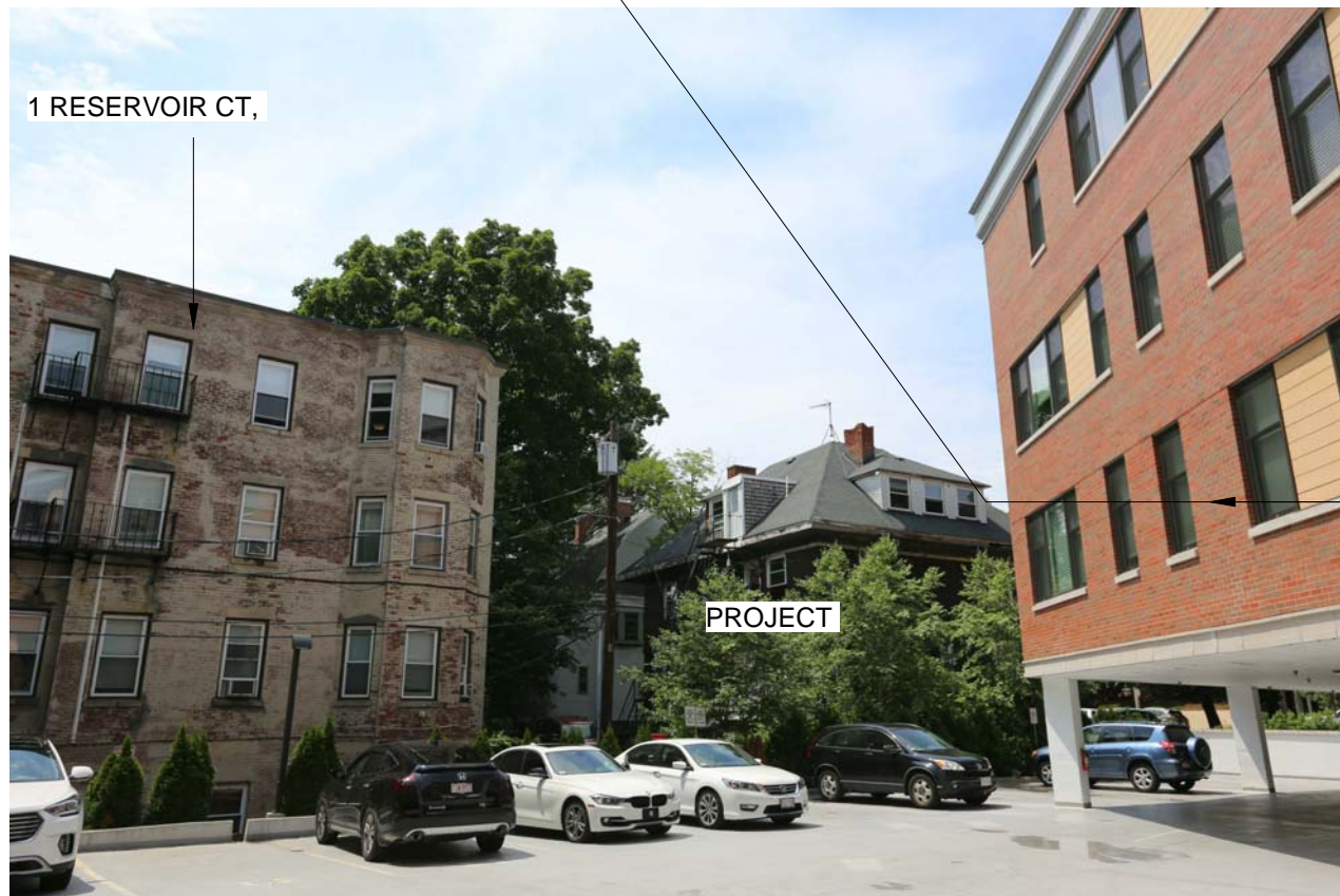
VIEW 2 LOOKING NORTHWEST FROM ADJACENT PARKING
