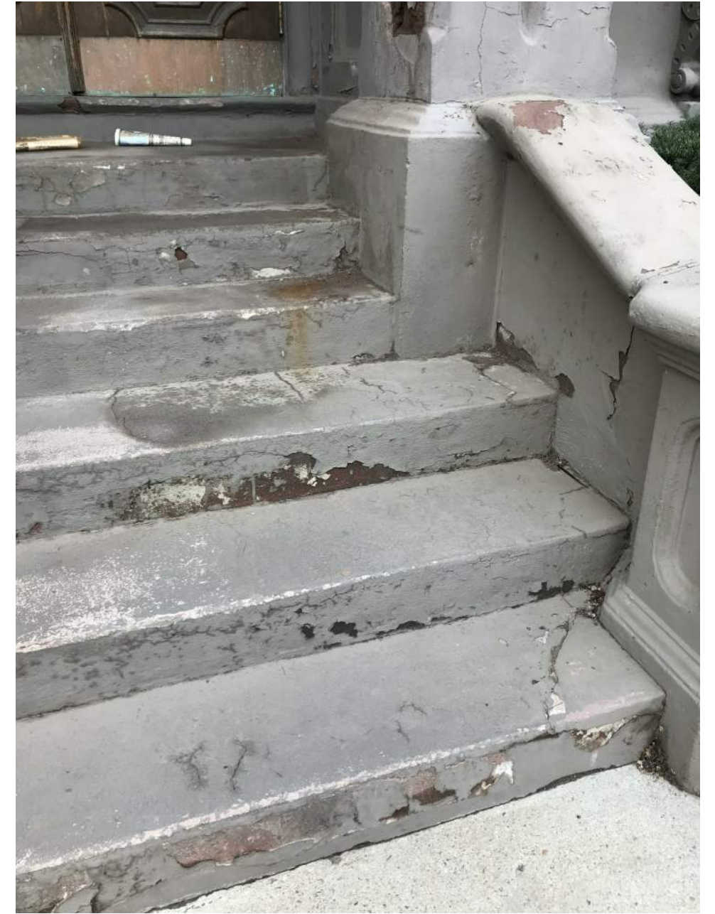
EXISTING FRONT STOOP TO BE REPAIRED AND RESTORED. PAINT HC-69.
