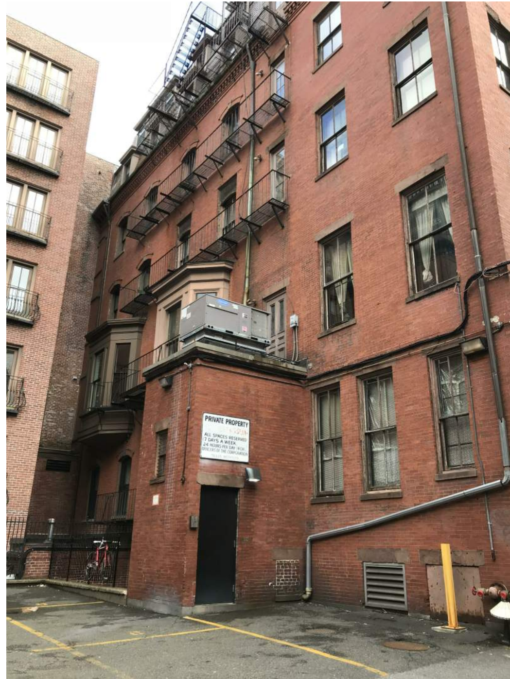
REAR FACADE - 10-11 ARLINGTON STREET
