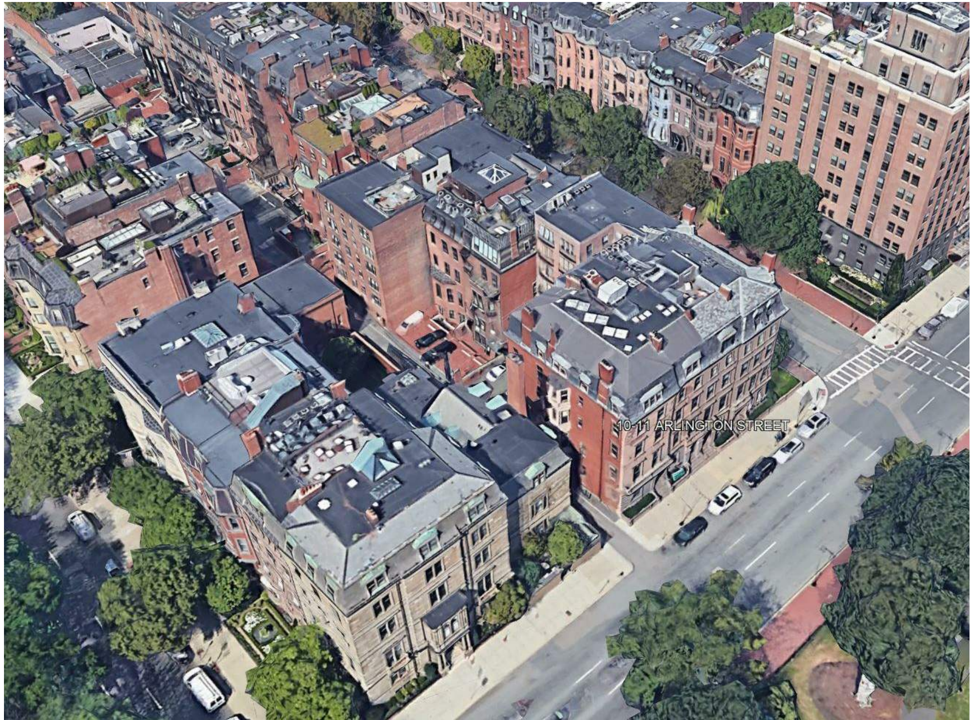
OVERHEAD VIEW OF 10-11 ARLINGTON STREET LOOKING NORTHWEST
