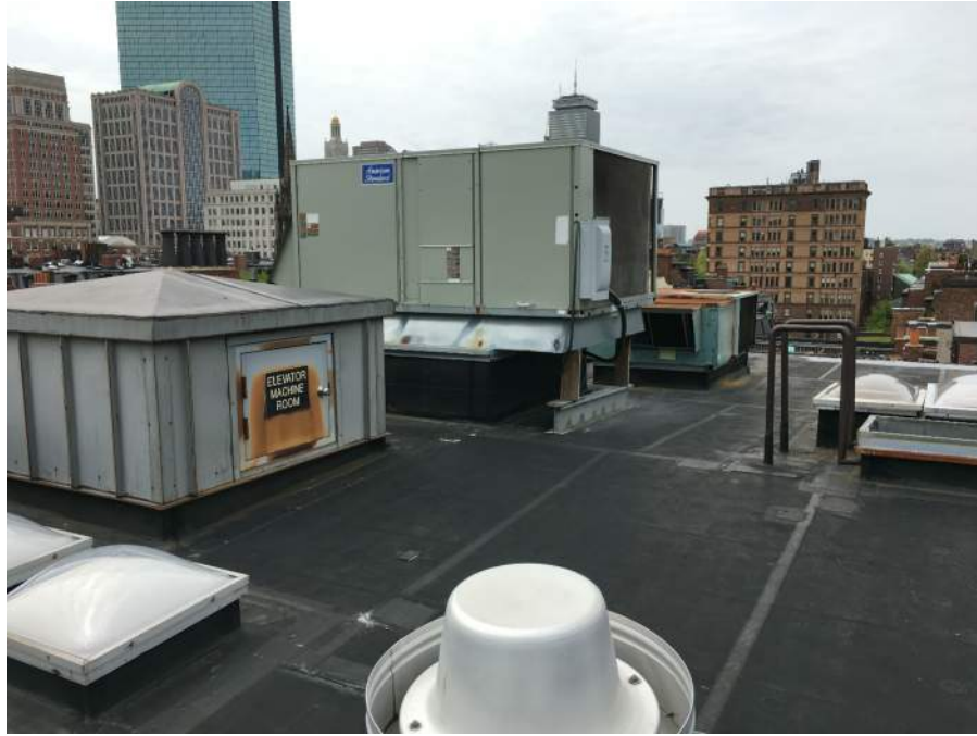
VIEW FROM NE CORNER OF 10-11 ARLINGTON STREET LOOKING WEST
