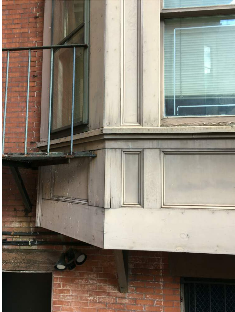
EXISTING NON-HISTORIC ORIEL SUPPORTED ON METAL BRACKETS
