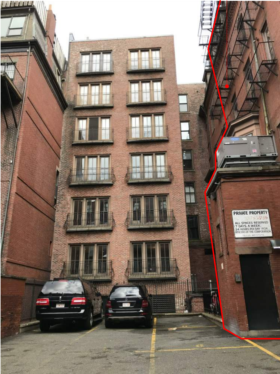
ALLEY CONDITION AT REAR OF 10-11 ARLINGTON STREET
