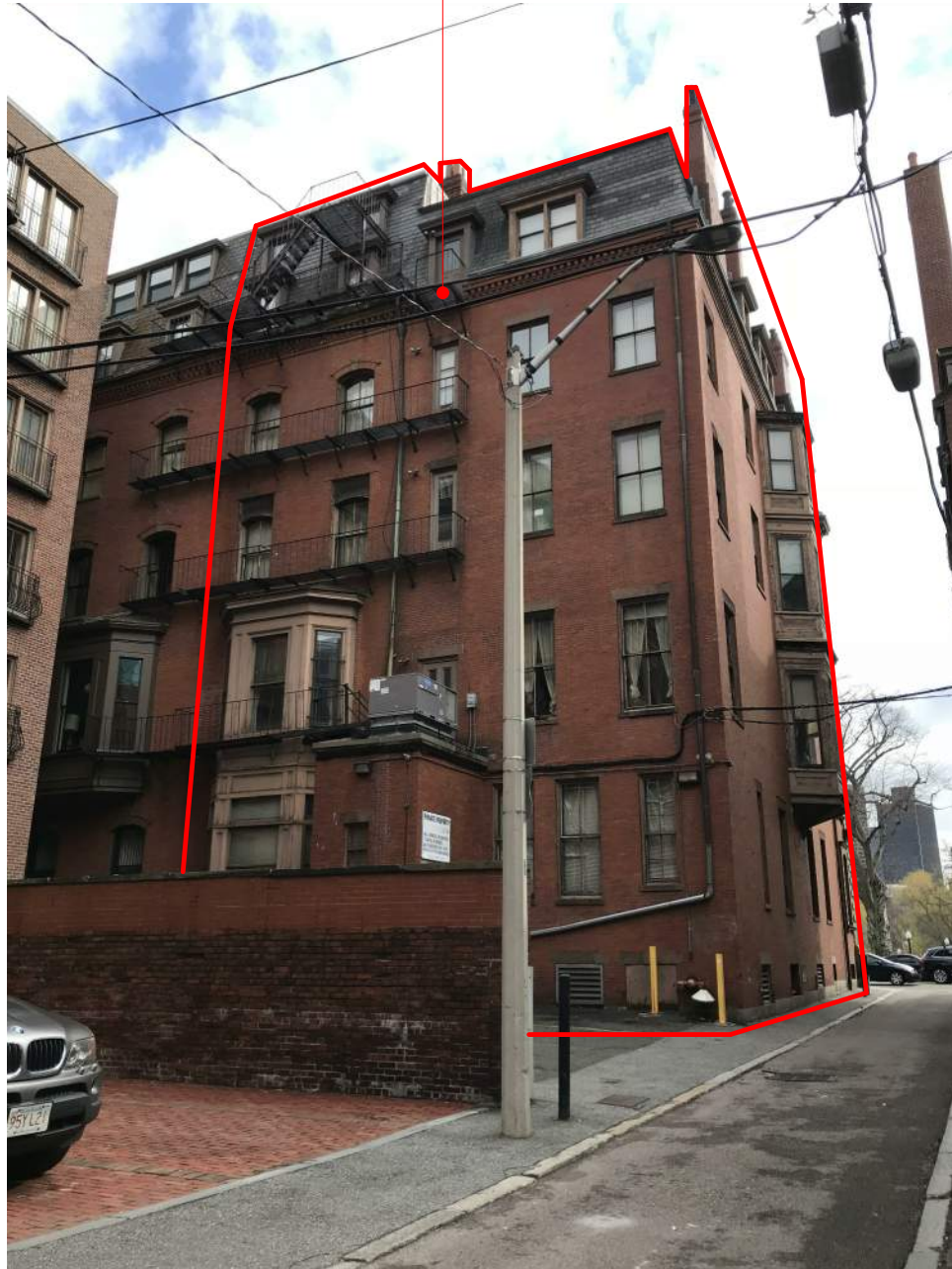
PUBLIC ALLEY 422 LOOKING EAST
