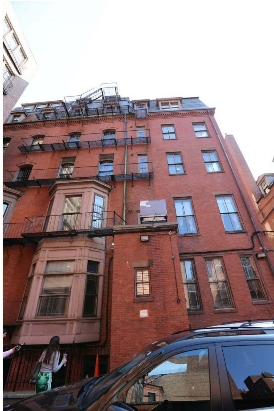
REAR FACADE - 10-11 ARLINGTON STREET
