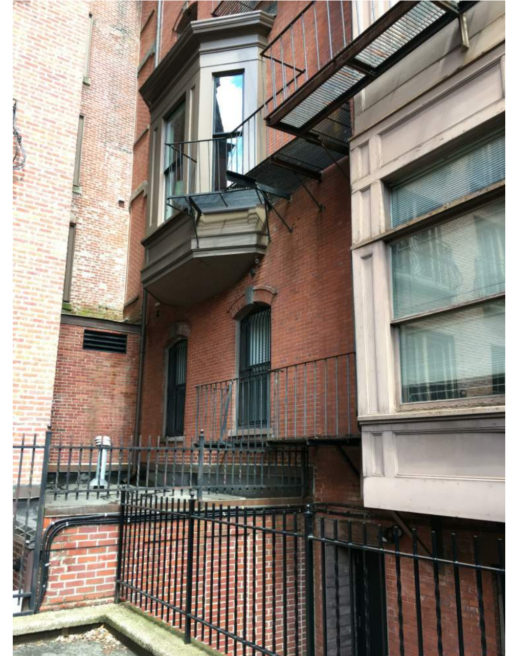
MATCHING SINGLE STORY ORIEL AT NEIGHBORING PROPERTY
