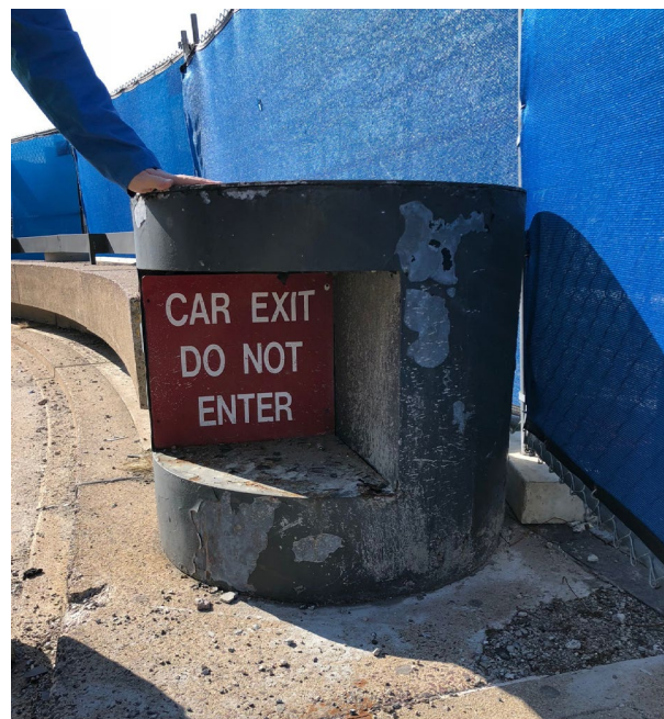
Existing Sign to be replaced
