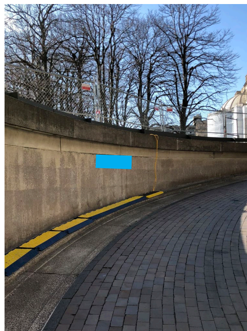
Located on interior face of spiral ramp wall.
