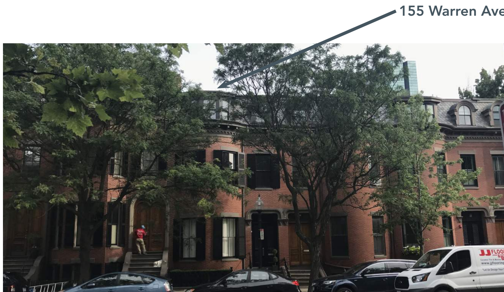
Streetscape across Warren Avenue
