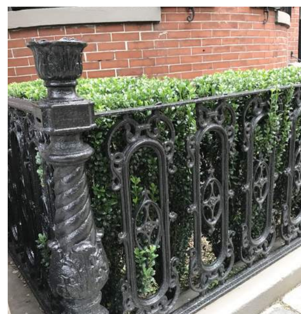
Existing Ornamental Rail
