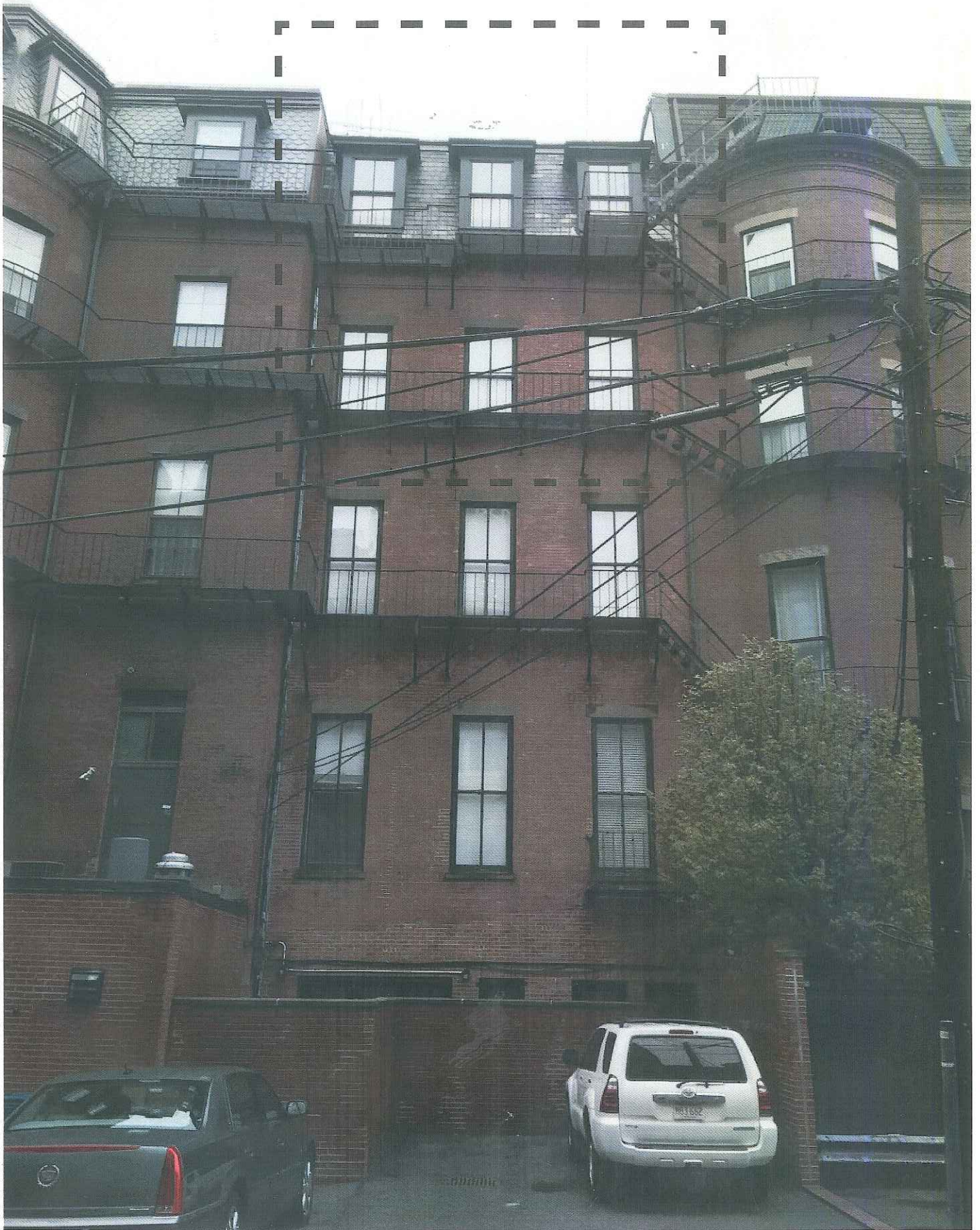
42 Commonwealth Ave. , Apt. 5 Rear View
