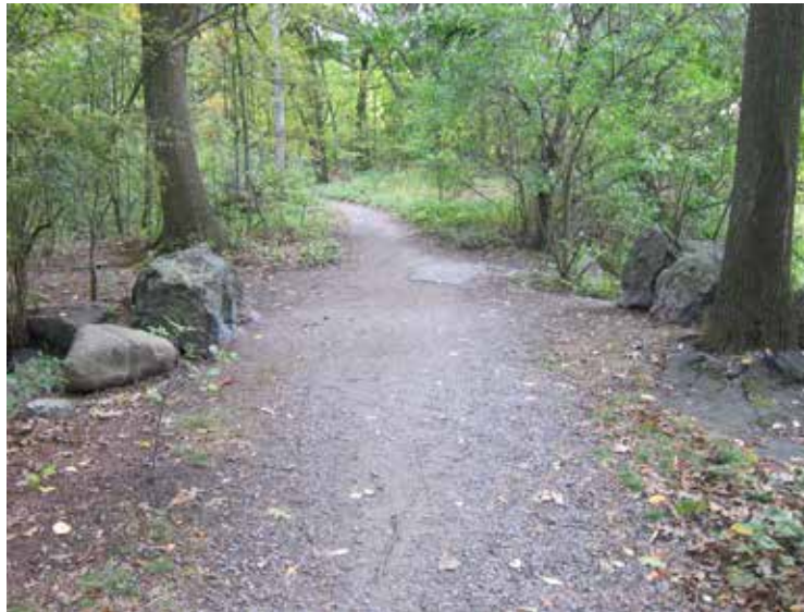
Main Path - Compacted earth and gravel
