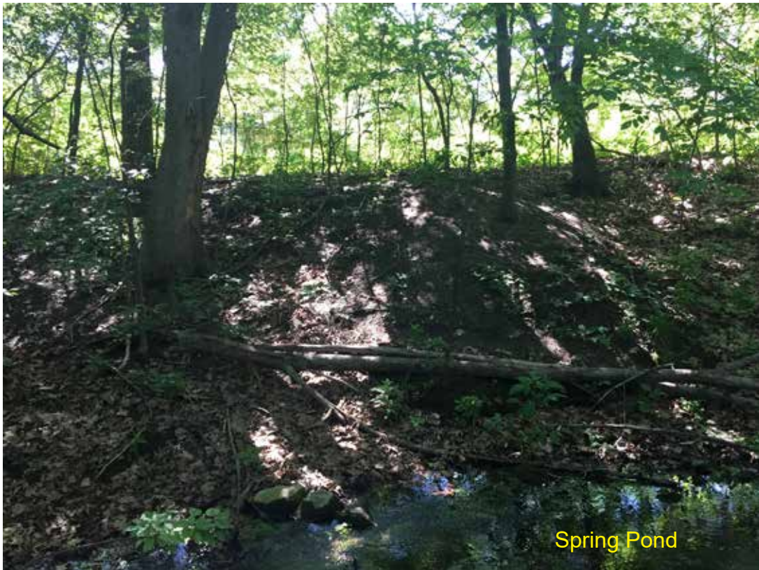
Area of bank stabilization, soil regeneration and supplemental planting
