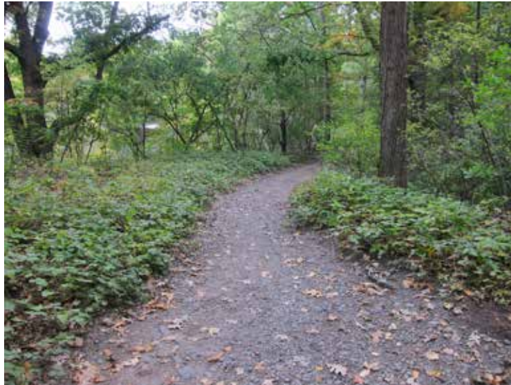
Main Path - Compacted earth and gravel
