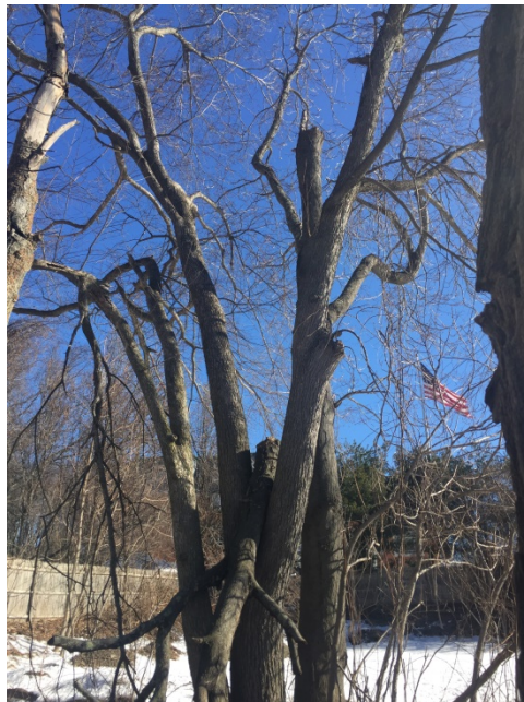
2 mature trees on slope near inlet to culvert
