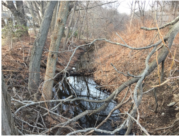
View upstream from culvert
