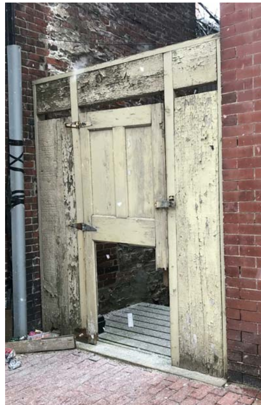
Photo of Existing Gate at 112 Myrtle St.
