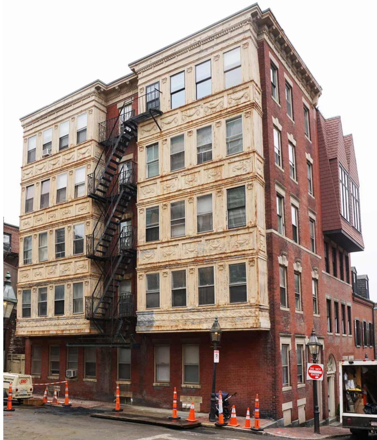
VIEW FROM CORNER OF GROVE STREET & MYRTLE STREET
