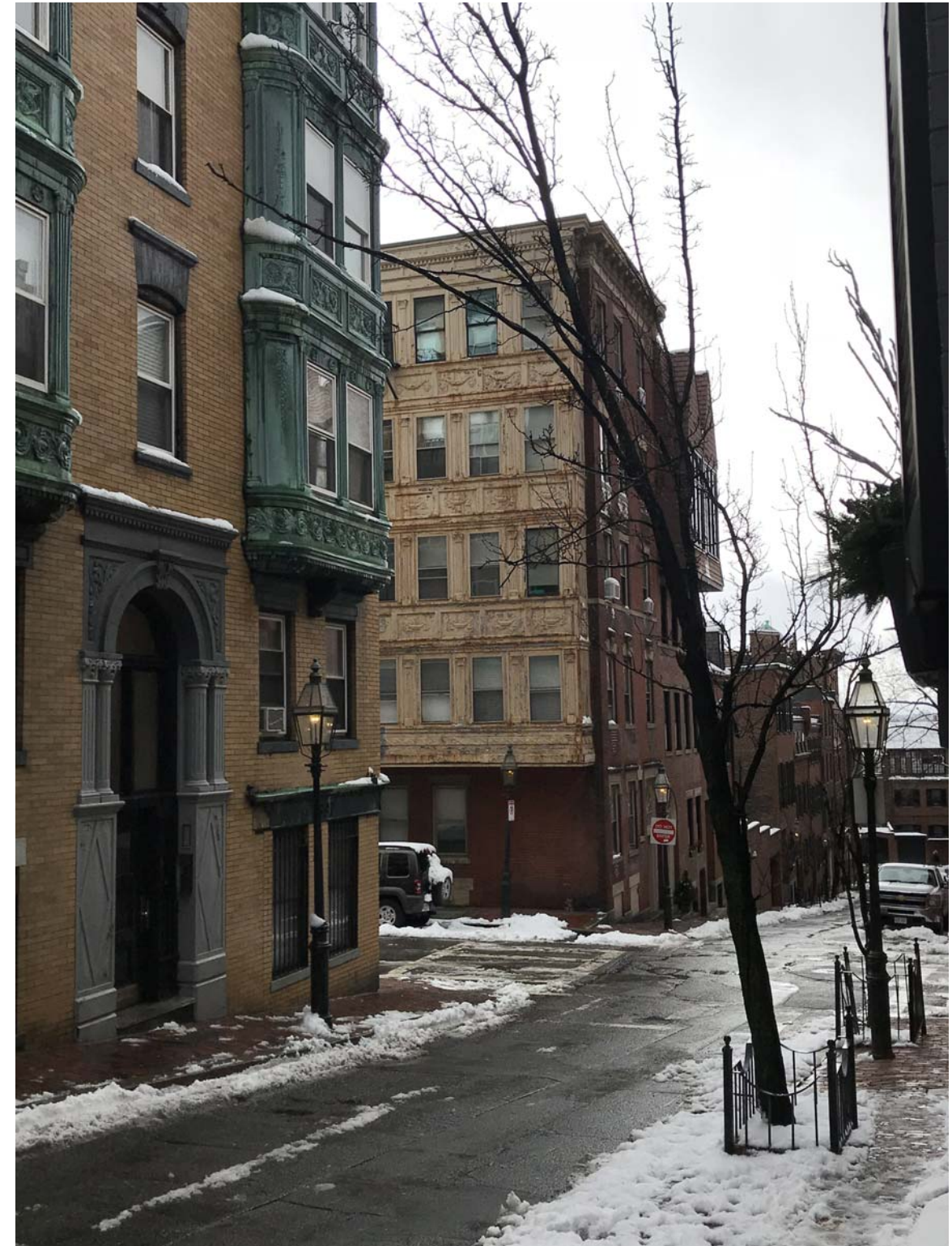
MOCK-UP PHOTO FROM MYRTLE STREET LOOKING WEST (MOCK-UP NOT VISIBLE)
