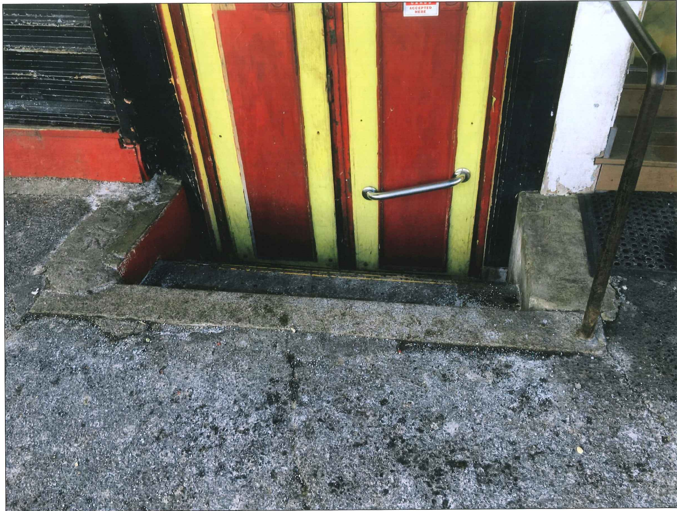
BLACKSTONE STREET IMAGES - EXISTING GRANITE TREADS (IMAGE 6)
