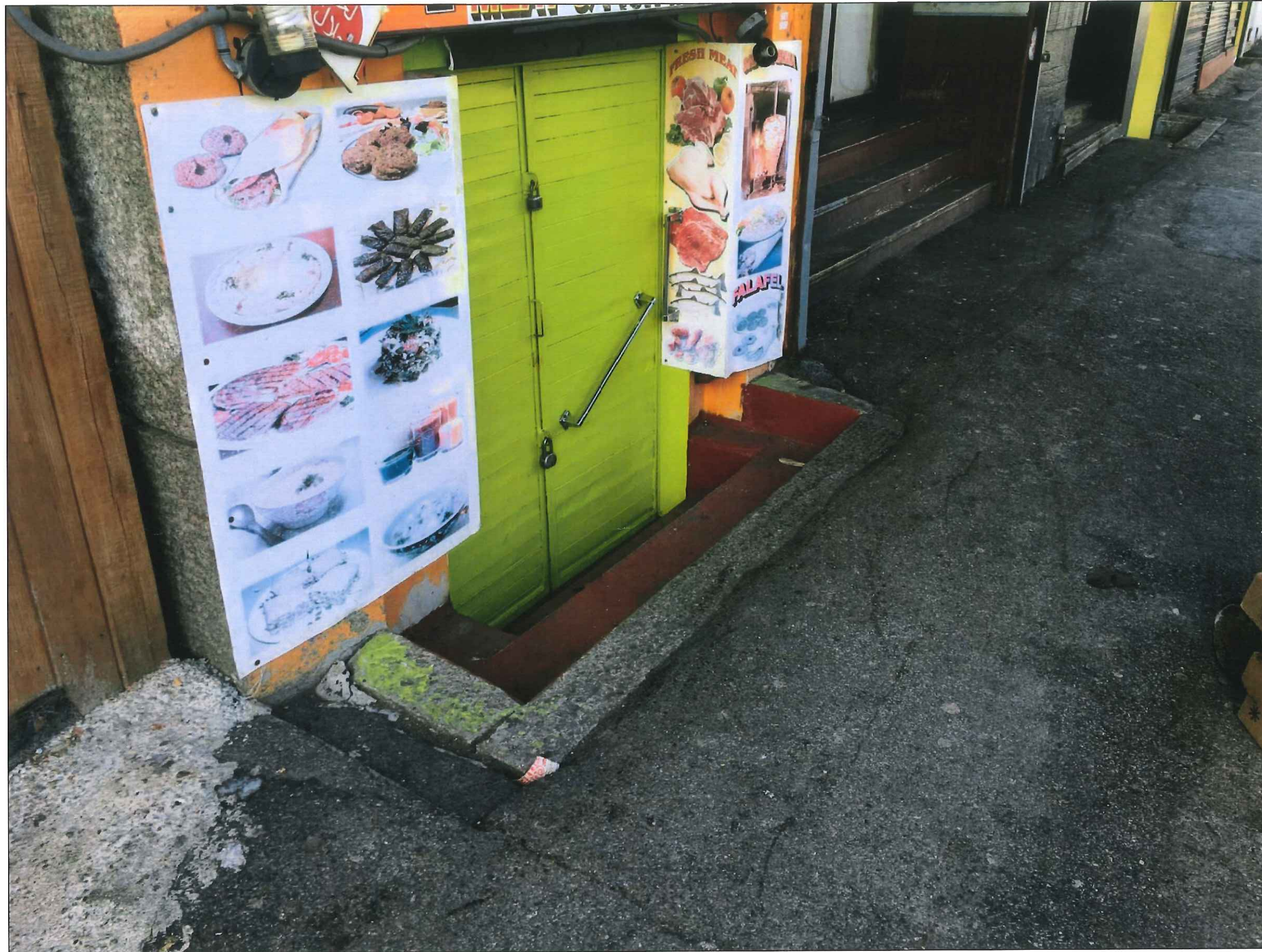
BLACKSTONE STREET IMAGES - EXISTING GRANITE TREADS (IMAGE 9)
