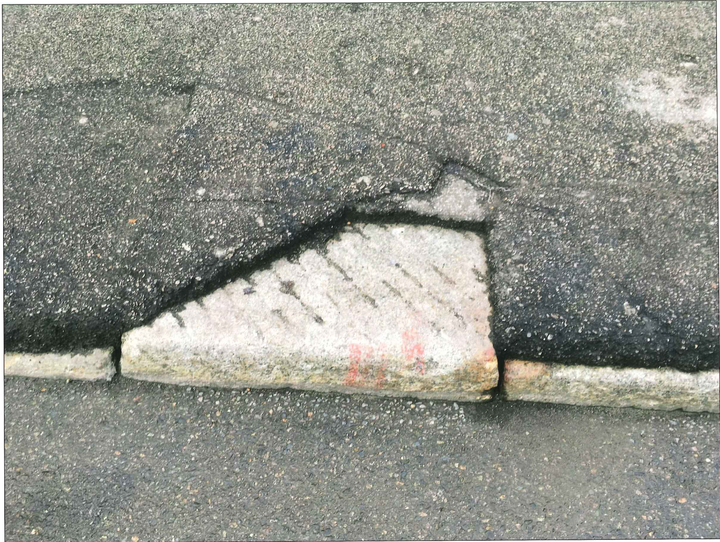
BLACKSTONE STREET IMAGES - EXISTING GRANITE EDGES (IMAGE 10 B)
