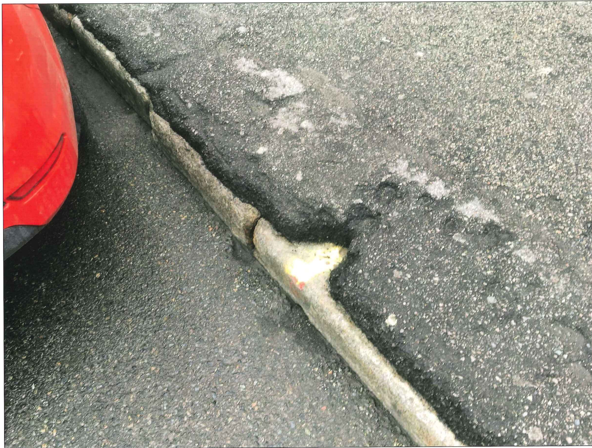
BLACKSTONE STREET IMAGES - EXISTING GRANITE EDGES (IMAGE 10 C)
