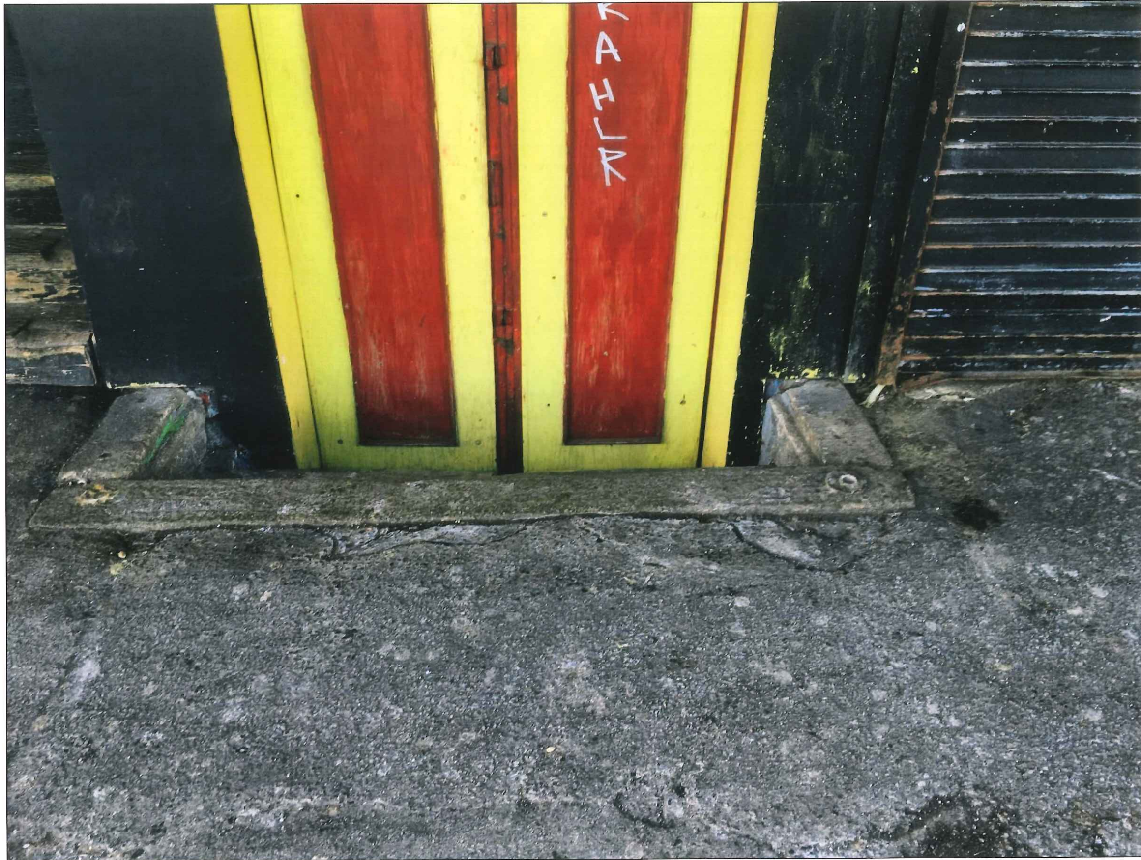
BLACKSTONE STREET IMAGES - EXISTING GRANITE TREADS (IMAGE 8)
