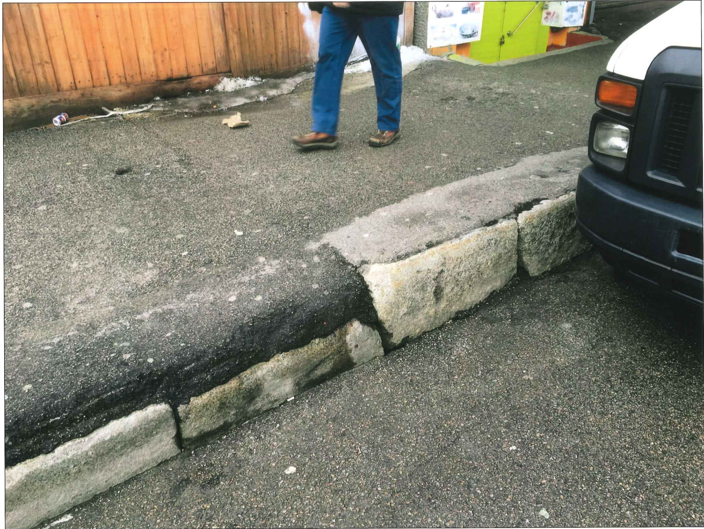
BLACKSTONE STREET IMAGES - EXISTING GRANITE EDGES (IMAGE 10 A)
