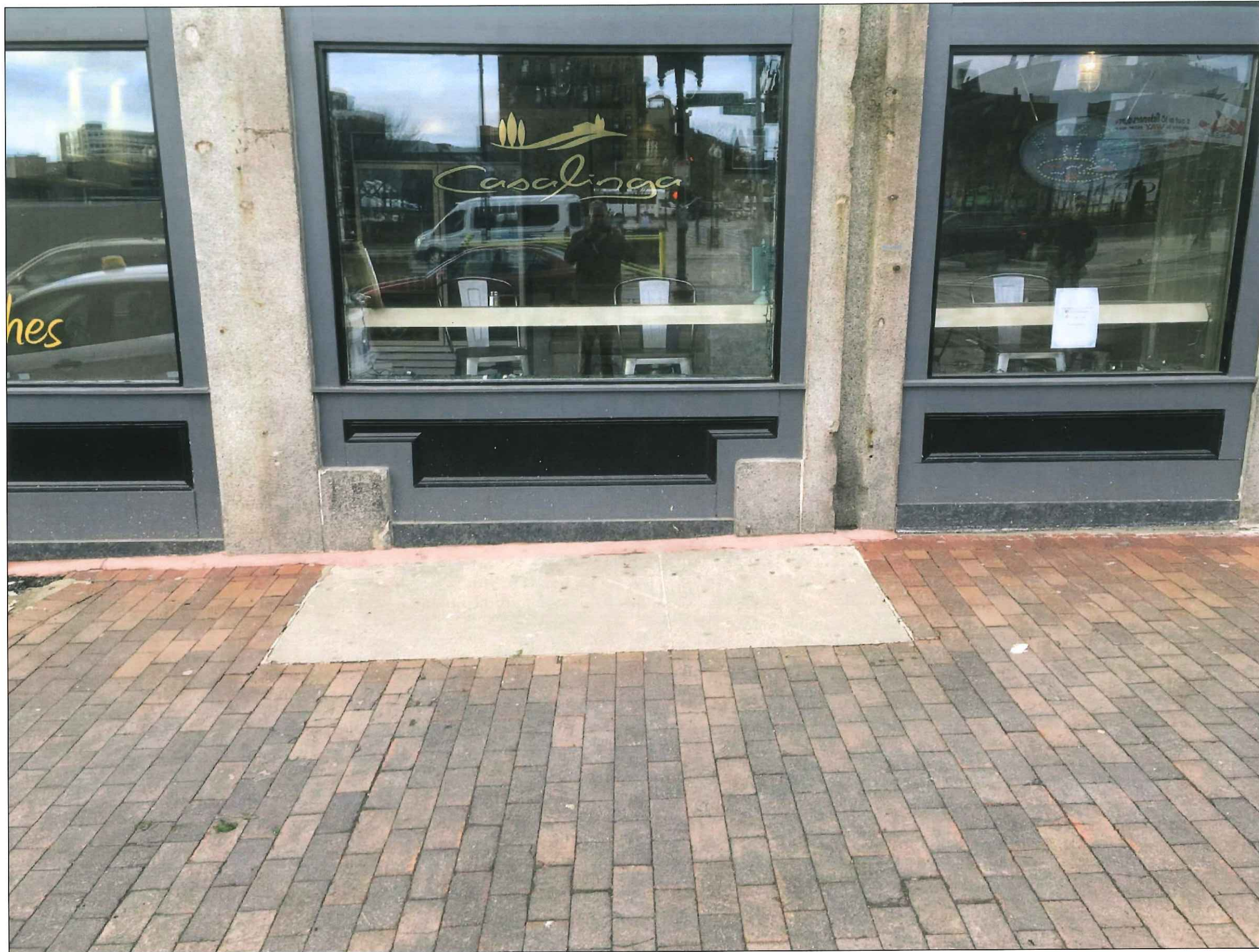
BLACKSTONE STREET IMAGES - EXISTING CONCRETE SLAB (IMAGE 1)
