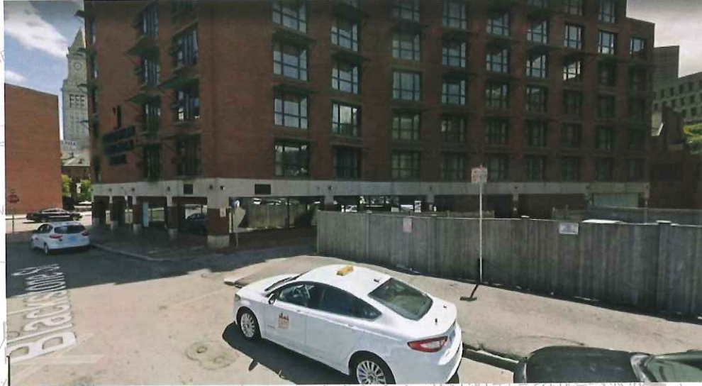
D - Existing Bituminous Sidewalk and Brick Sidewalks
