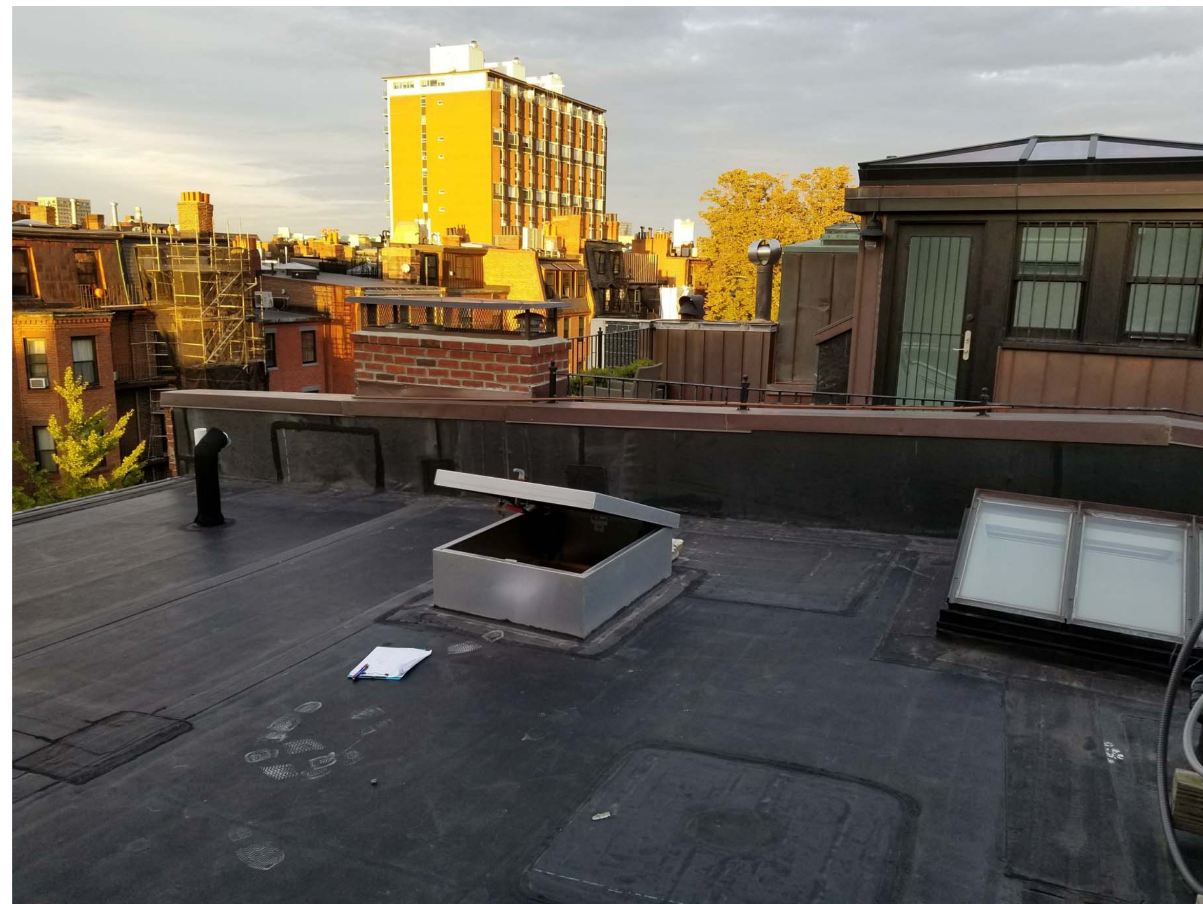
EXISTING - LOOKING NE TOWARDS 315 MARLBOROUGH
