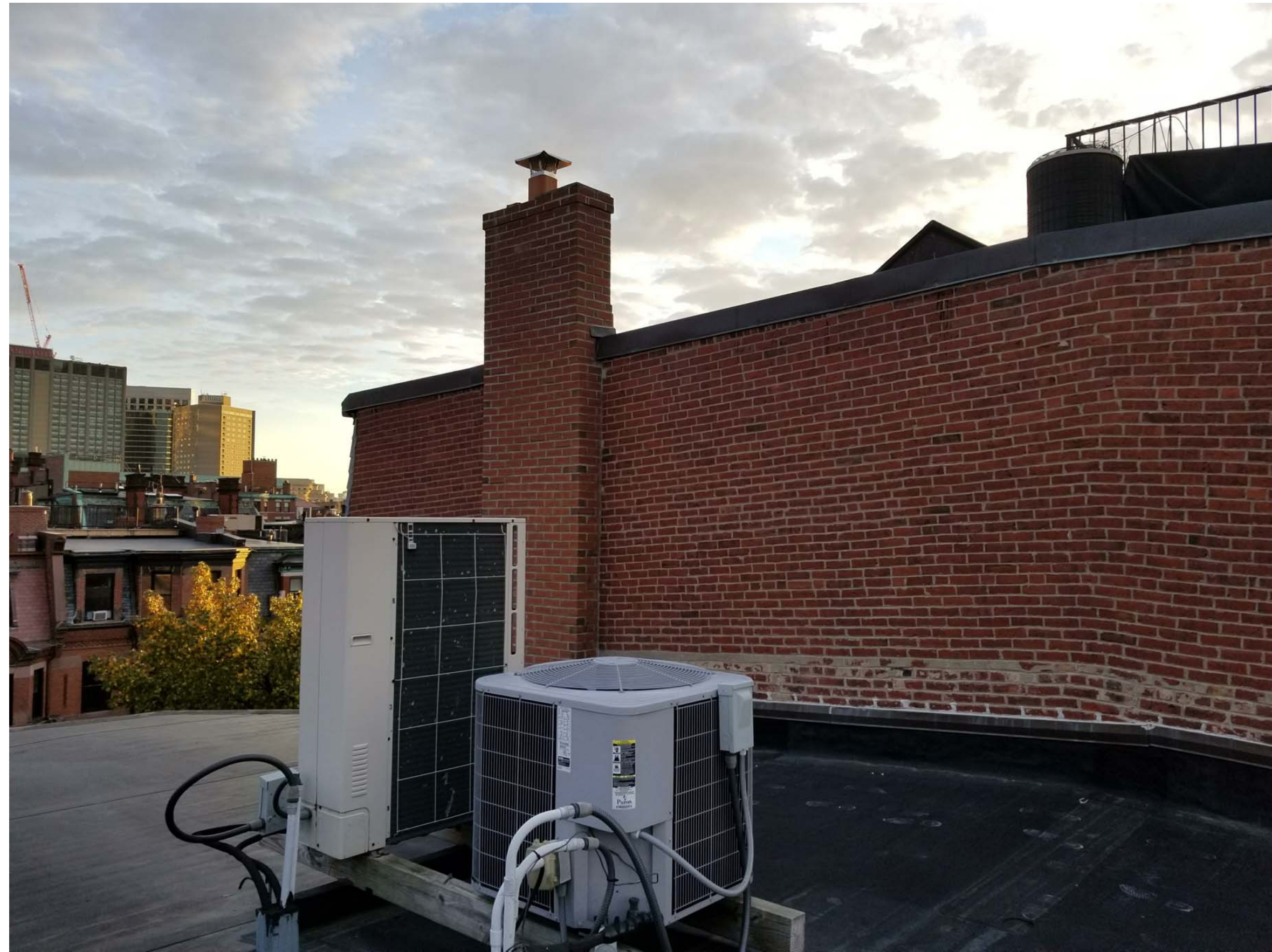
EXISTING - LOOKING SW TOWARDS 319 MARLBOROUGH
