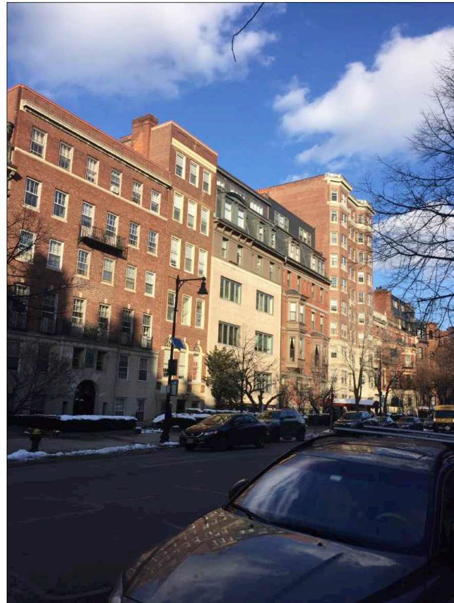
20 Existing Street View corner of Beacon & Exeter Street Scale: 1/8" = 1'-0"
