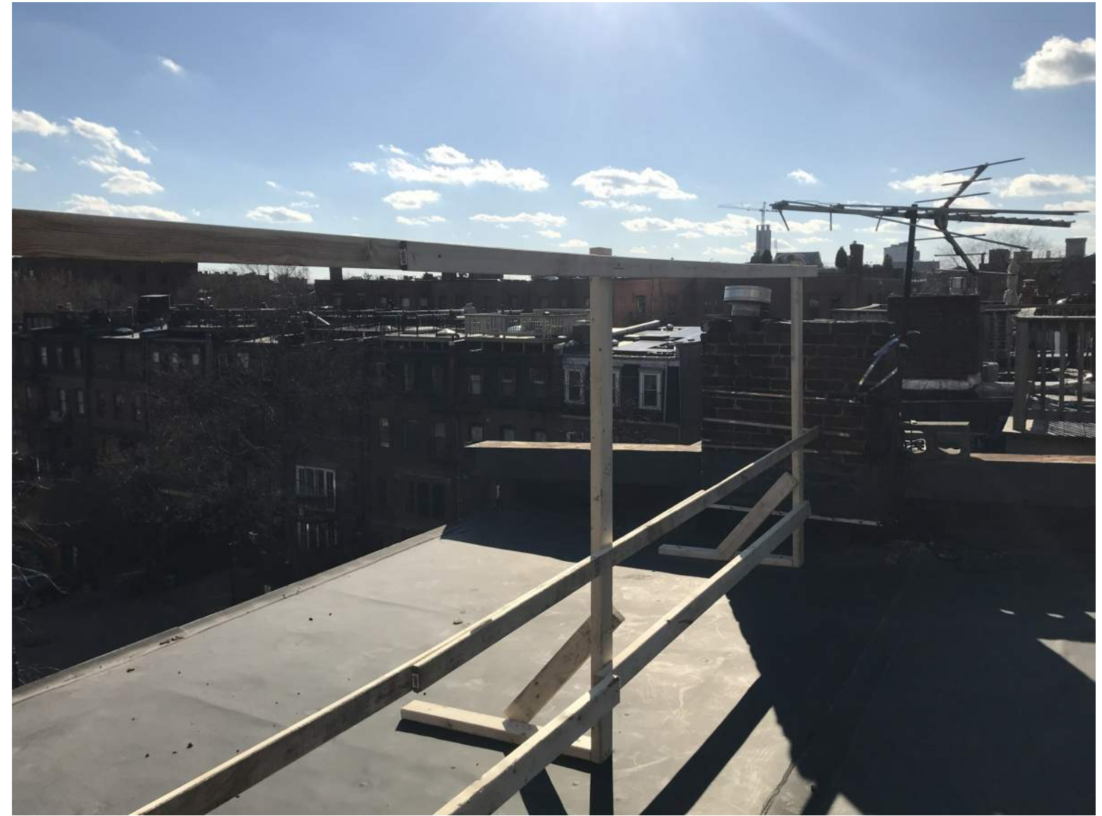
MOCK UP ON REAR OF BUILDING
