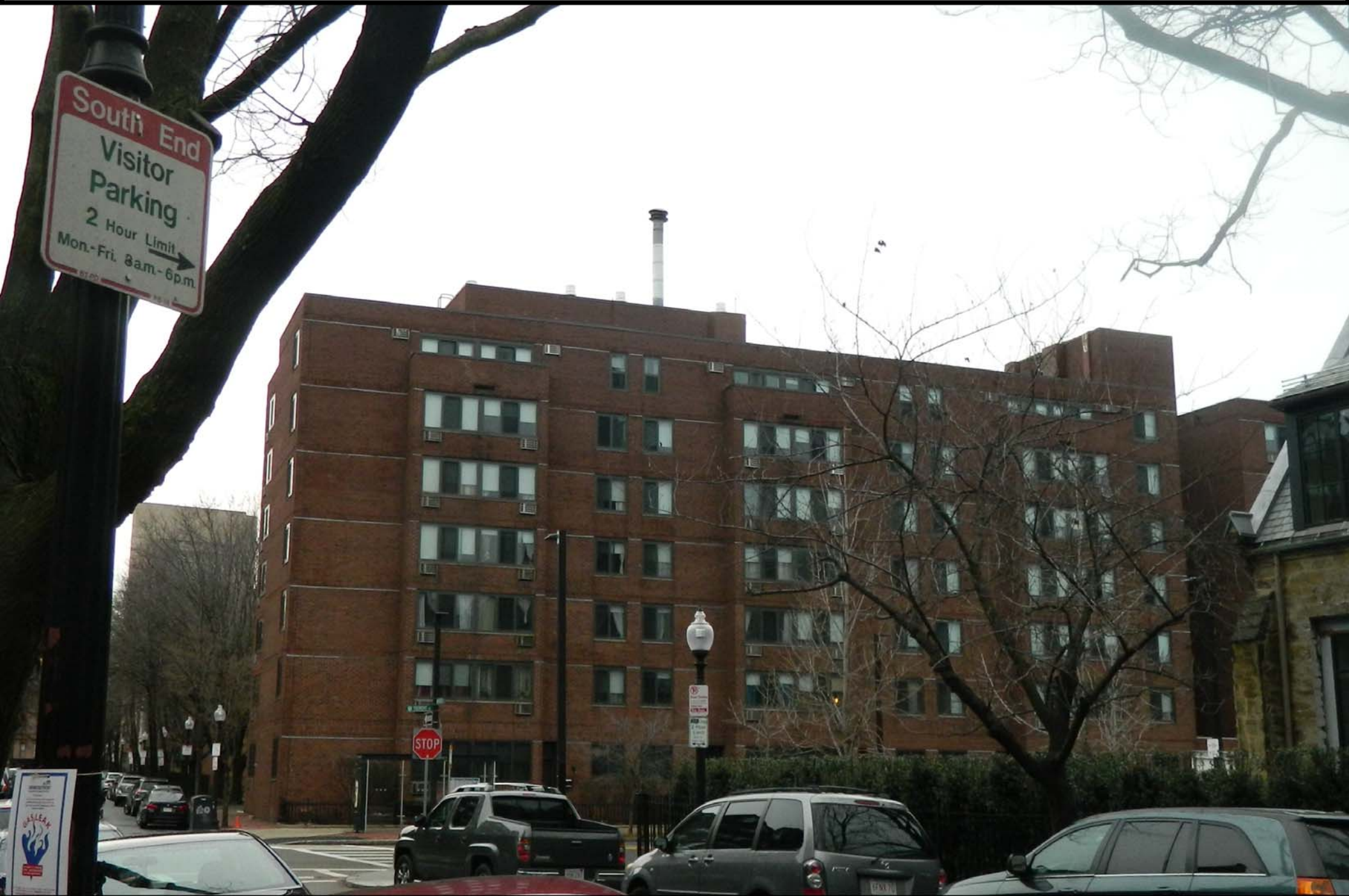
Photo taken from Worcester Street, 100 feet South of the existing building
