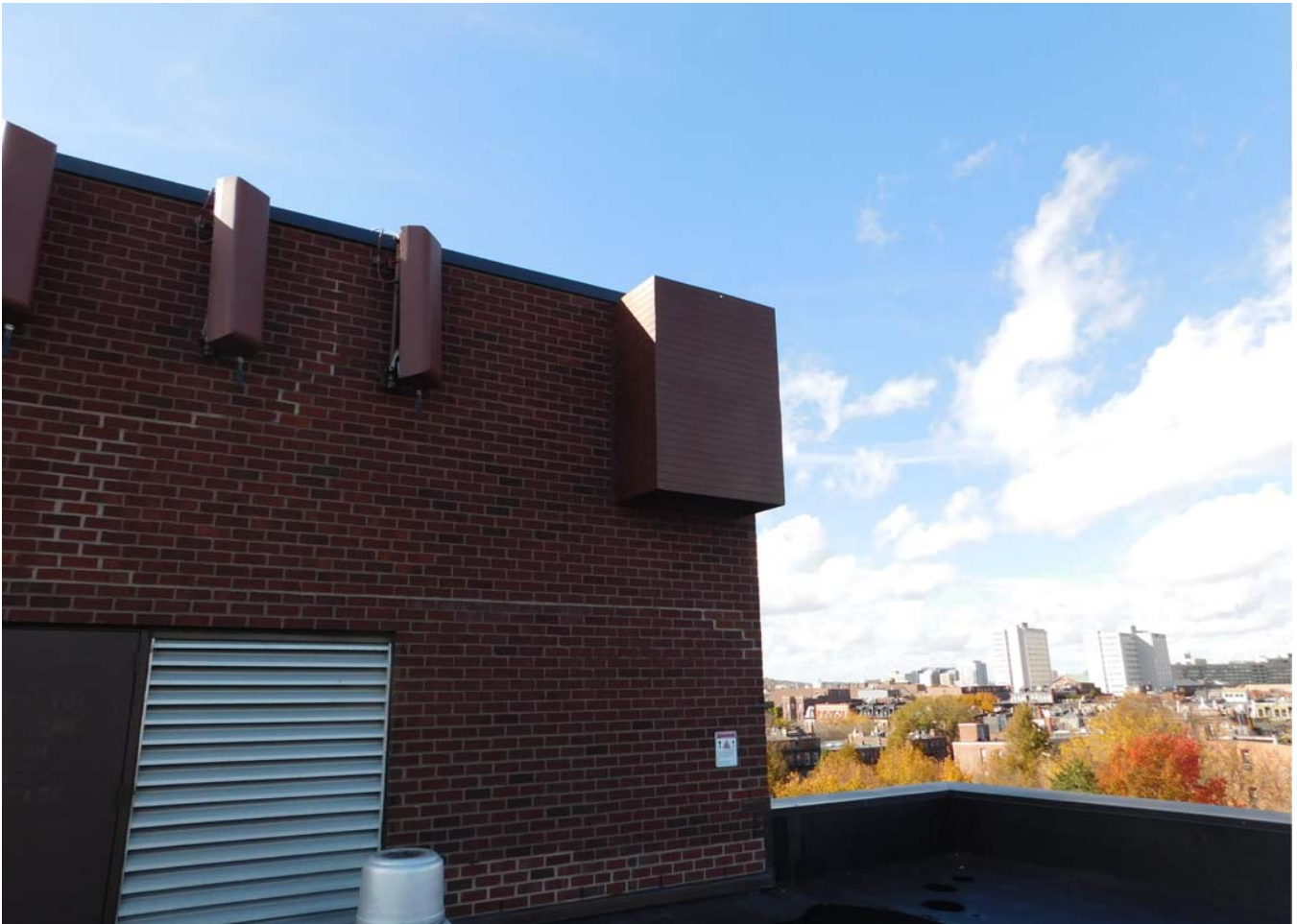
Existing Alpha Sector Antenna RF Enclosure
