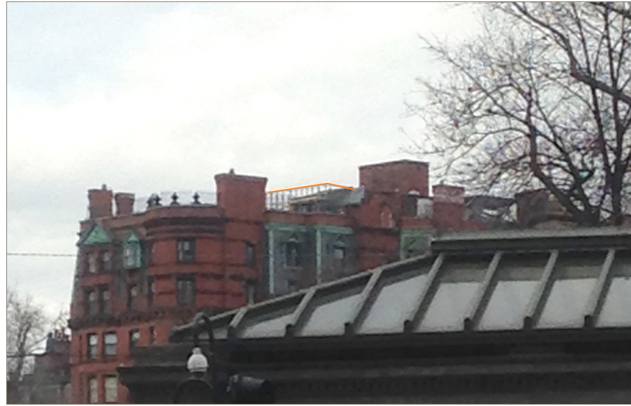
MOCK-UP FROM DOWNTOWN CROSSING
