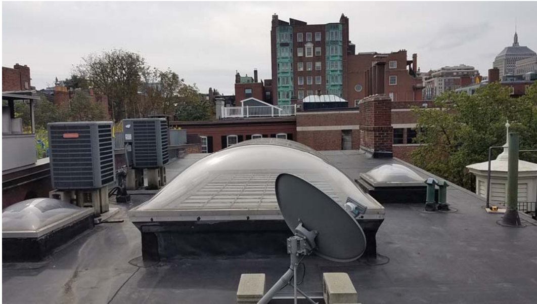
View of Existing Acrylic Domed Skylights Looking South
