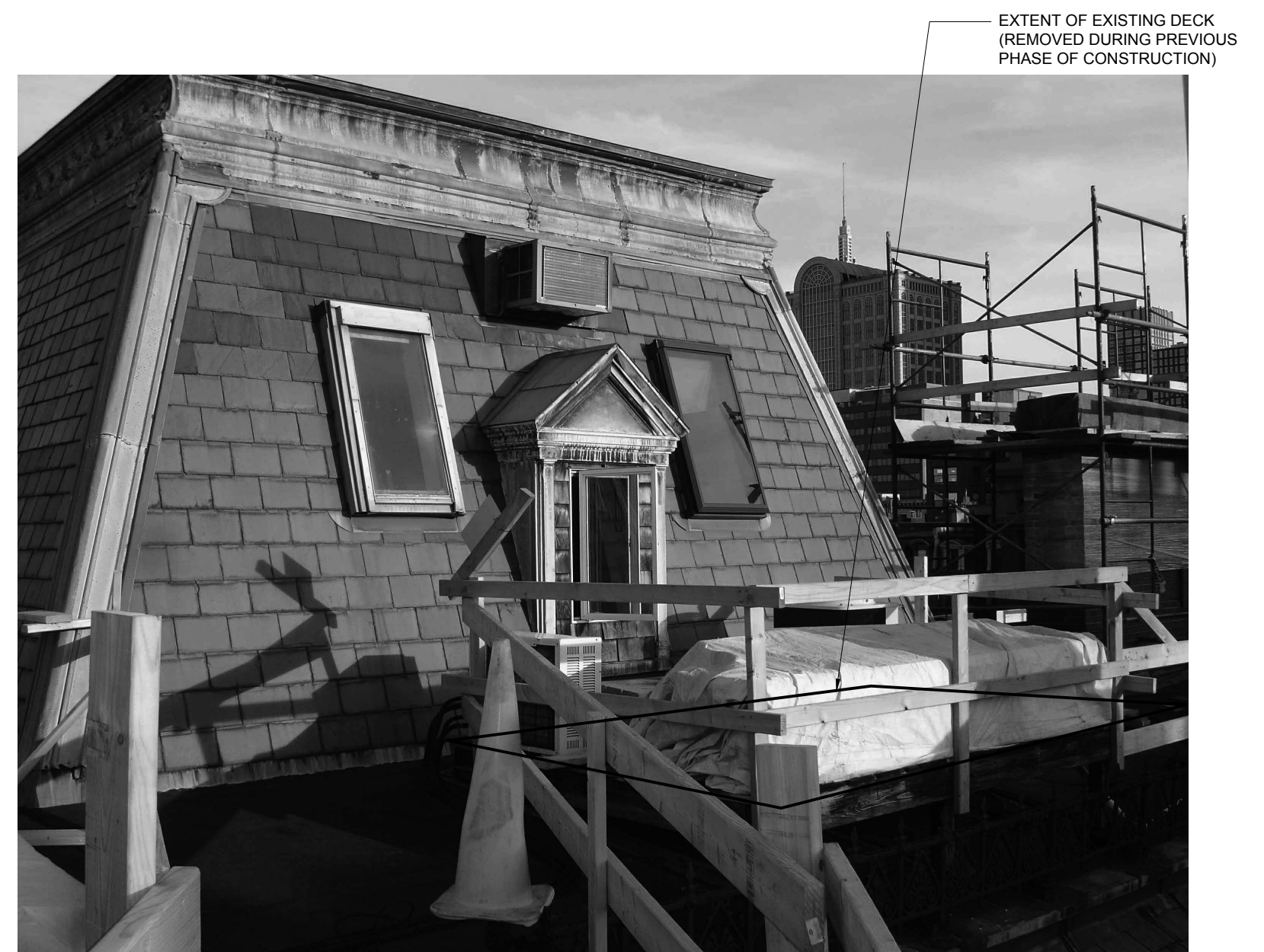
01 EXISTING CONDITIONS OF TOWER ROOF ACCESS N.T.S.
