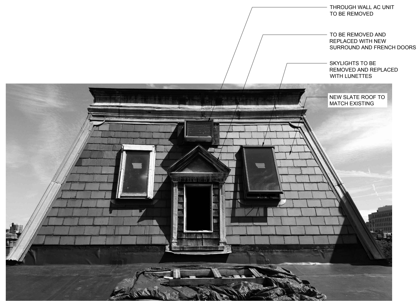
01 EXISTING CONDITIONS OF TOWER ROOF ACCESS N.T.S.
