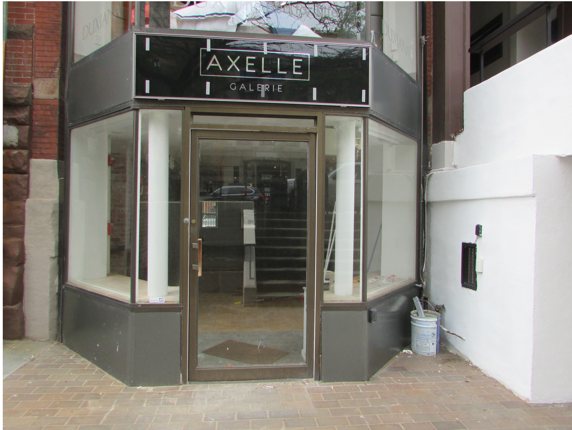
EXISTING CONDITIONS: STOREFRONT
