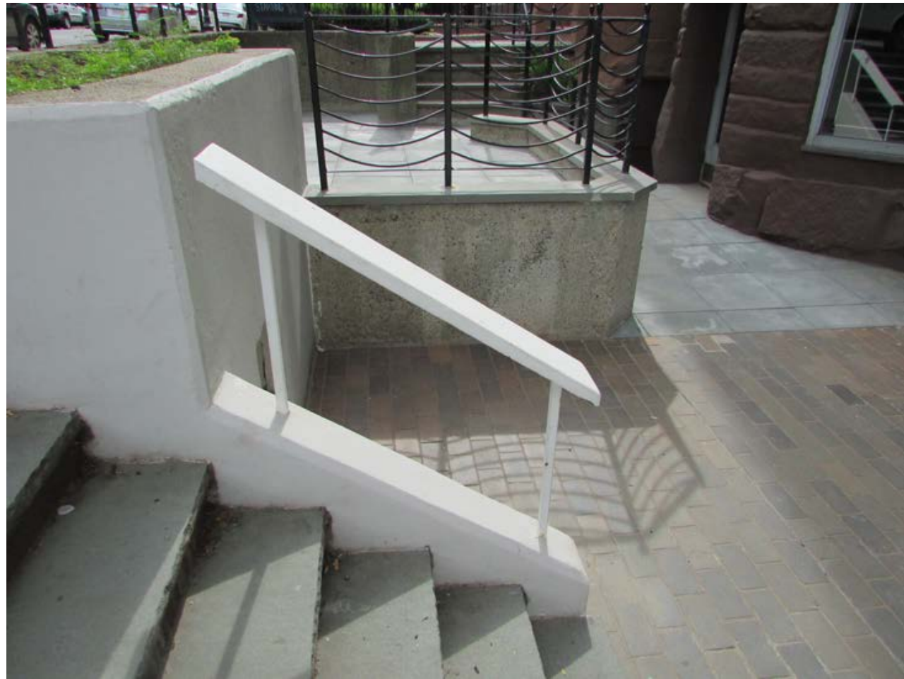
EXISTING CONDITIONS: PATIO
