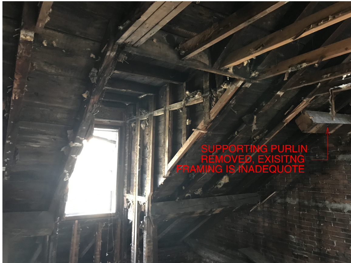
ROOF AT FRONT DORMER
