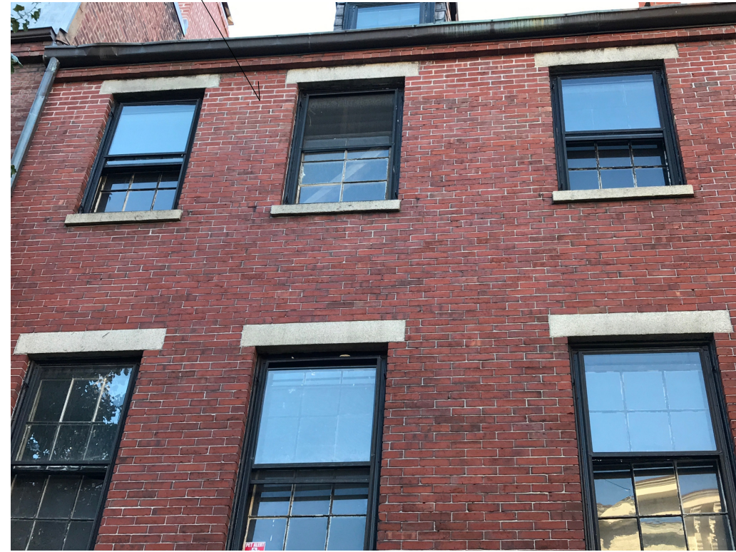
EXISTING BRICK FACADE
