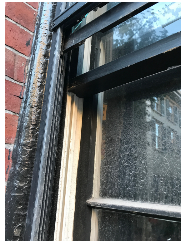
FIRST FLOOR WINDOW CASING
