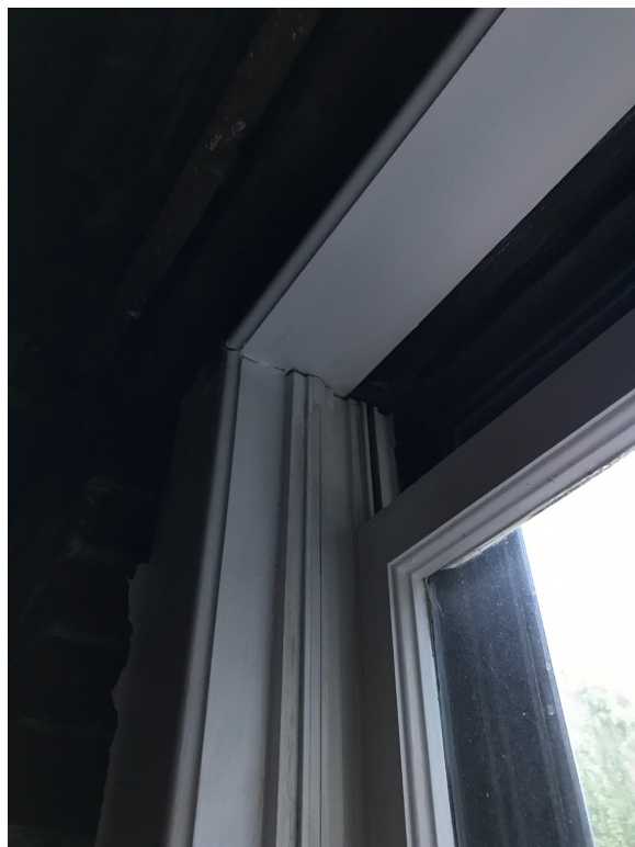
EXISTING REPLACEMENT WINDOWS
