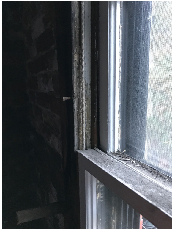
ORIGINAL FRAME WITH REPLACEMENT WOOD WINDOW SASH
