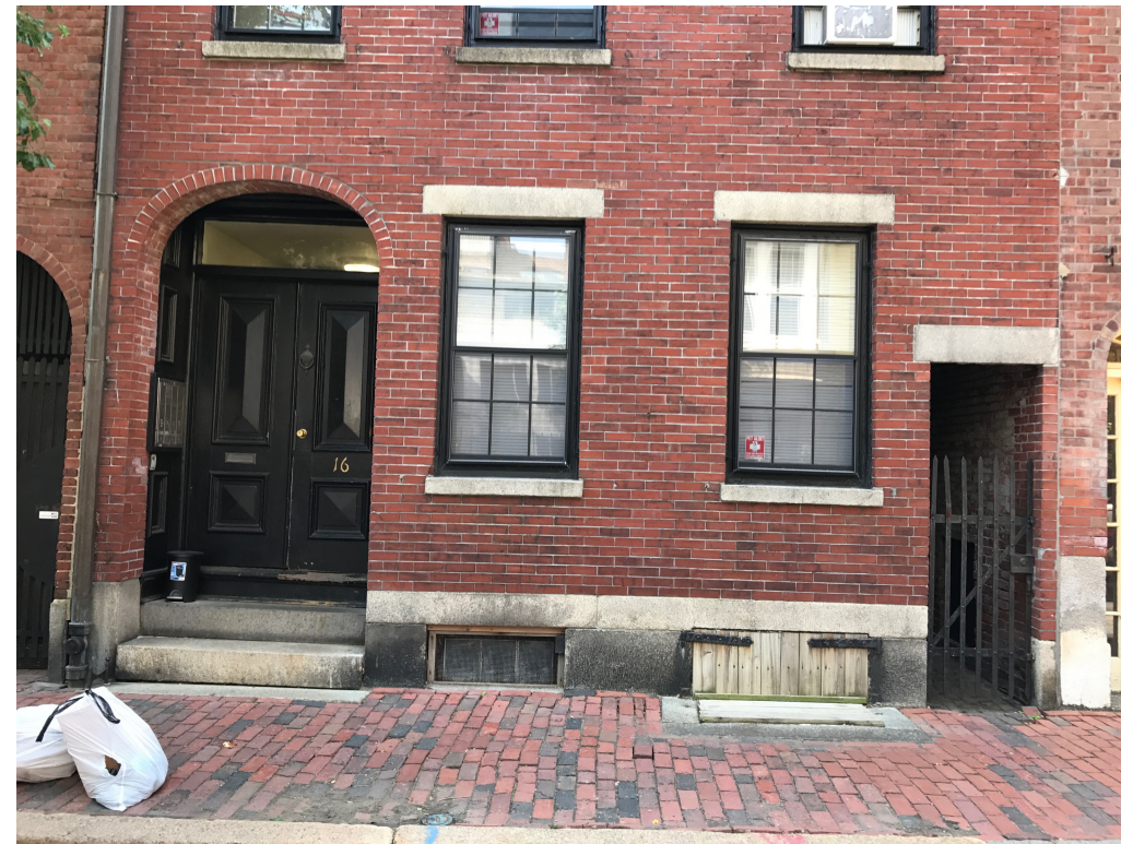
FRONT DOOR AND PASSAGE WAY GATE
