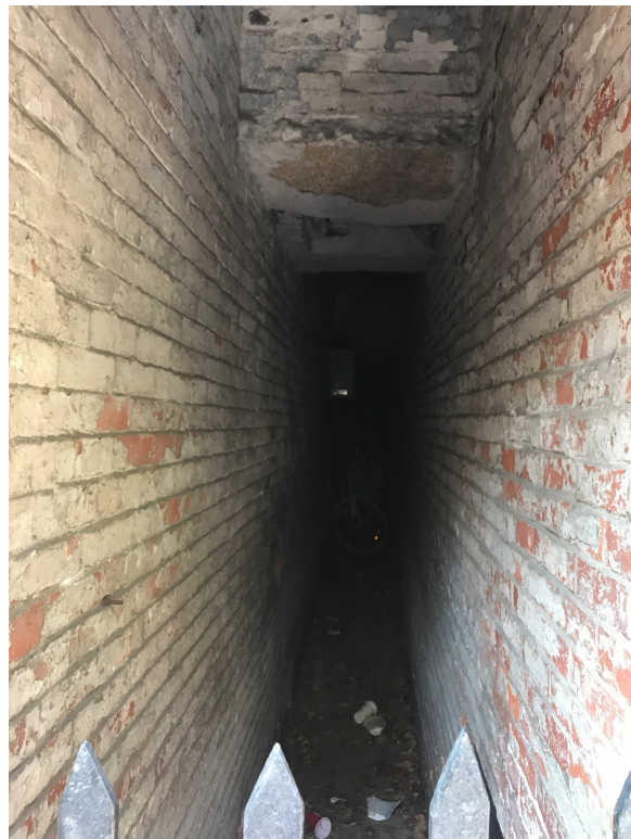
PASSAGE WAY TO REAR COURTYARD (SHED BLOCKED VIEW)
