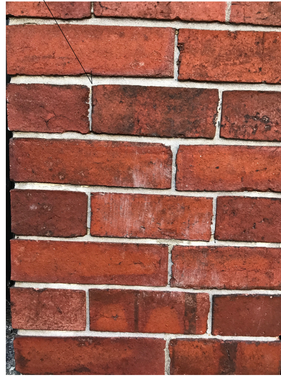
EXISTING BRICKS AND MORTAR JOINTS
