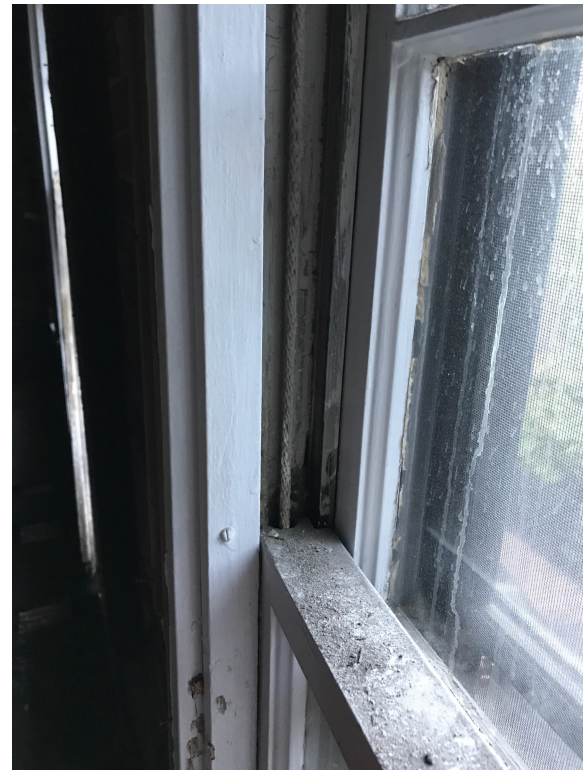
ORIGINAL FRAME WITH REPLACEMENT WOOD WINDOW SASH, NEW STOPS
