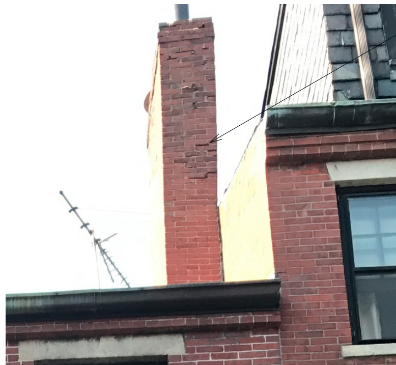
CHIMNEY: CRACKED AND LEANING
