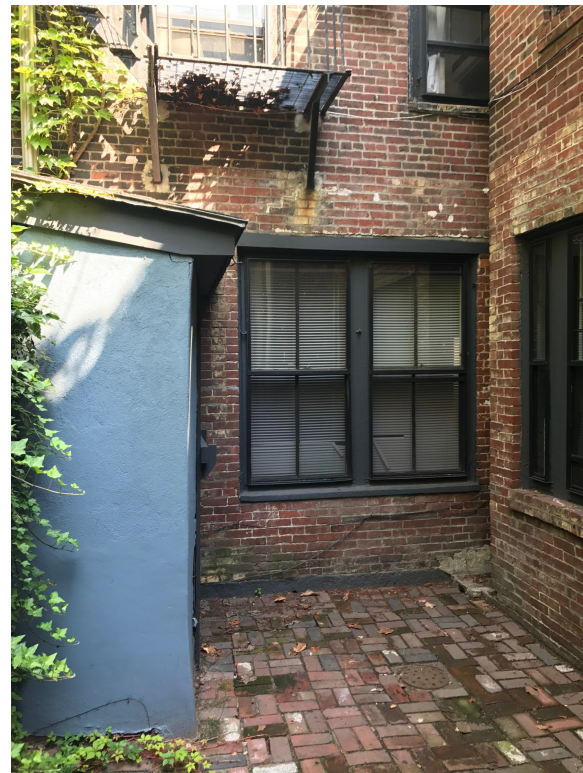
SHED AT REAR WHICH PREVIOUSLY BLOCKED VIEW FROM PINCKNEY TO COURTYARD
