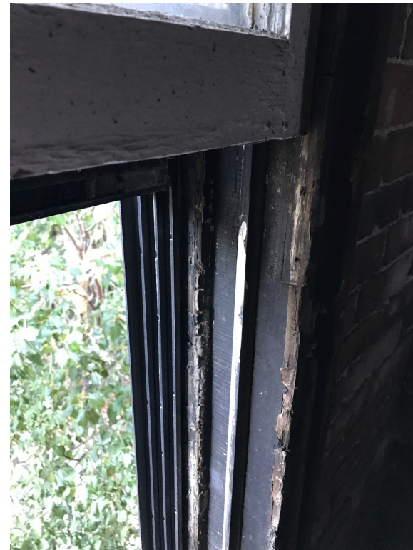
ORIGINAL FRAME WITH REPLACEMENT WOOD WINDOW SASH
