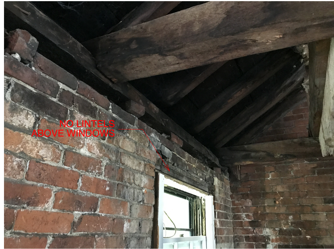
ROOF/WALL INTERSECTION
