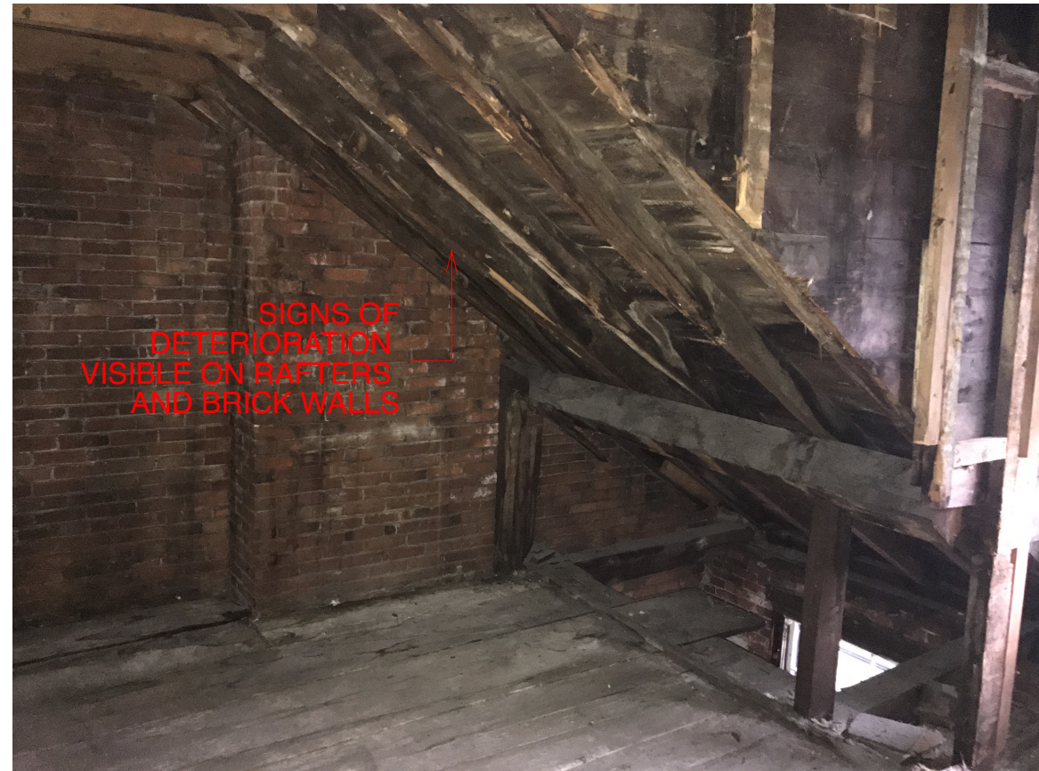
ROOF AT FRONT CHIMNEY
