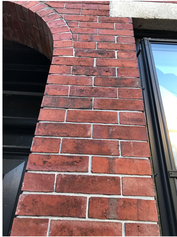
EXISTING BRICKS AND MORTAR JOINTS
