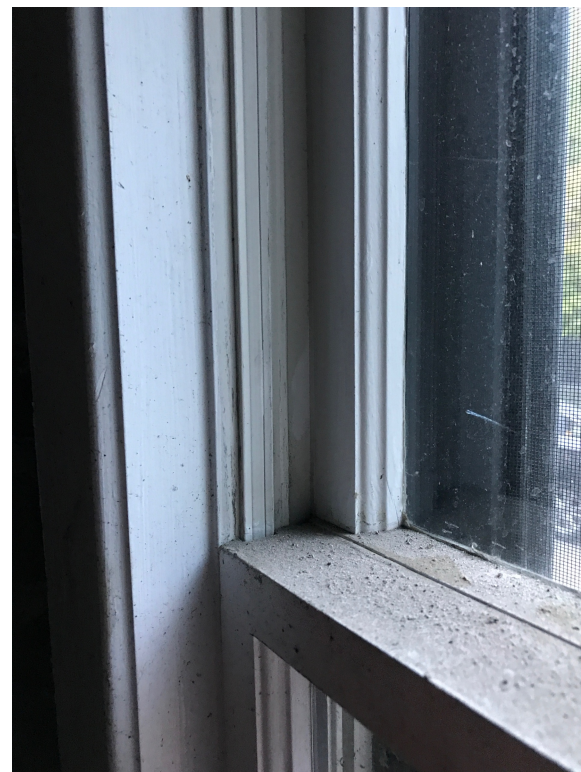
EXISTING REPLACEMENT WINDOWS
