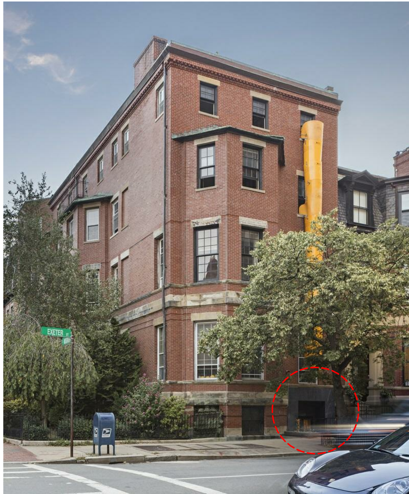
PHOTO 1. VIEW FROM CORNER OF EXETER AND MARLBOROUGH ST
