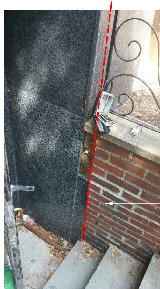
PHOTO 1. EXISTING BRICK CHEEK WALL
