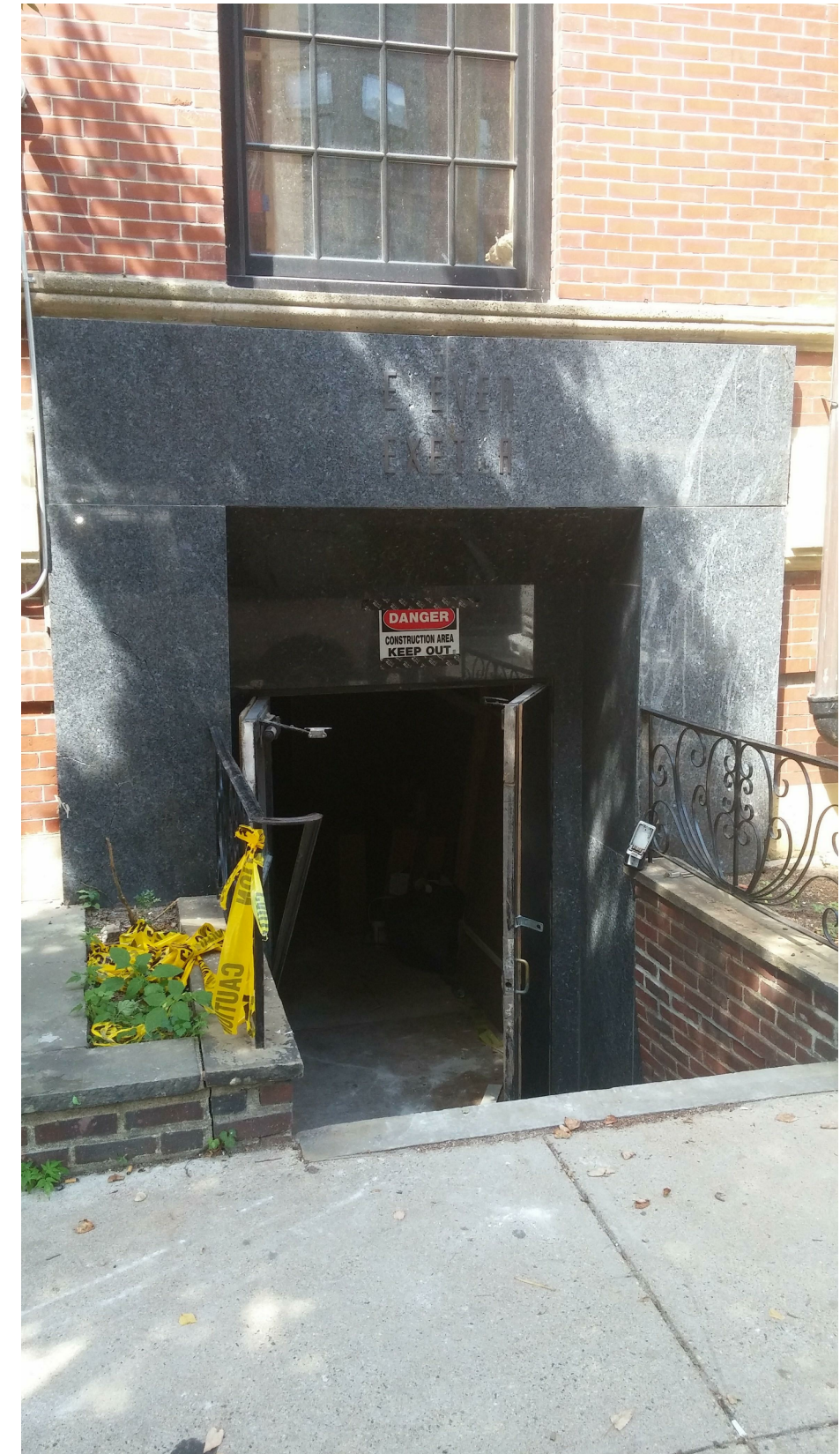
PHOTO 2. GRANITE CLADDING AT 11 EXETER ENTRY BEFORE CONSTRUCTION
