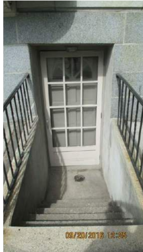
Front basement door, Beacon St.
