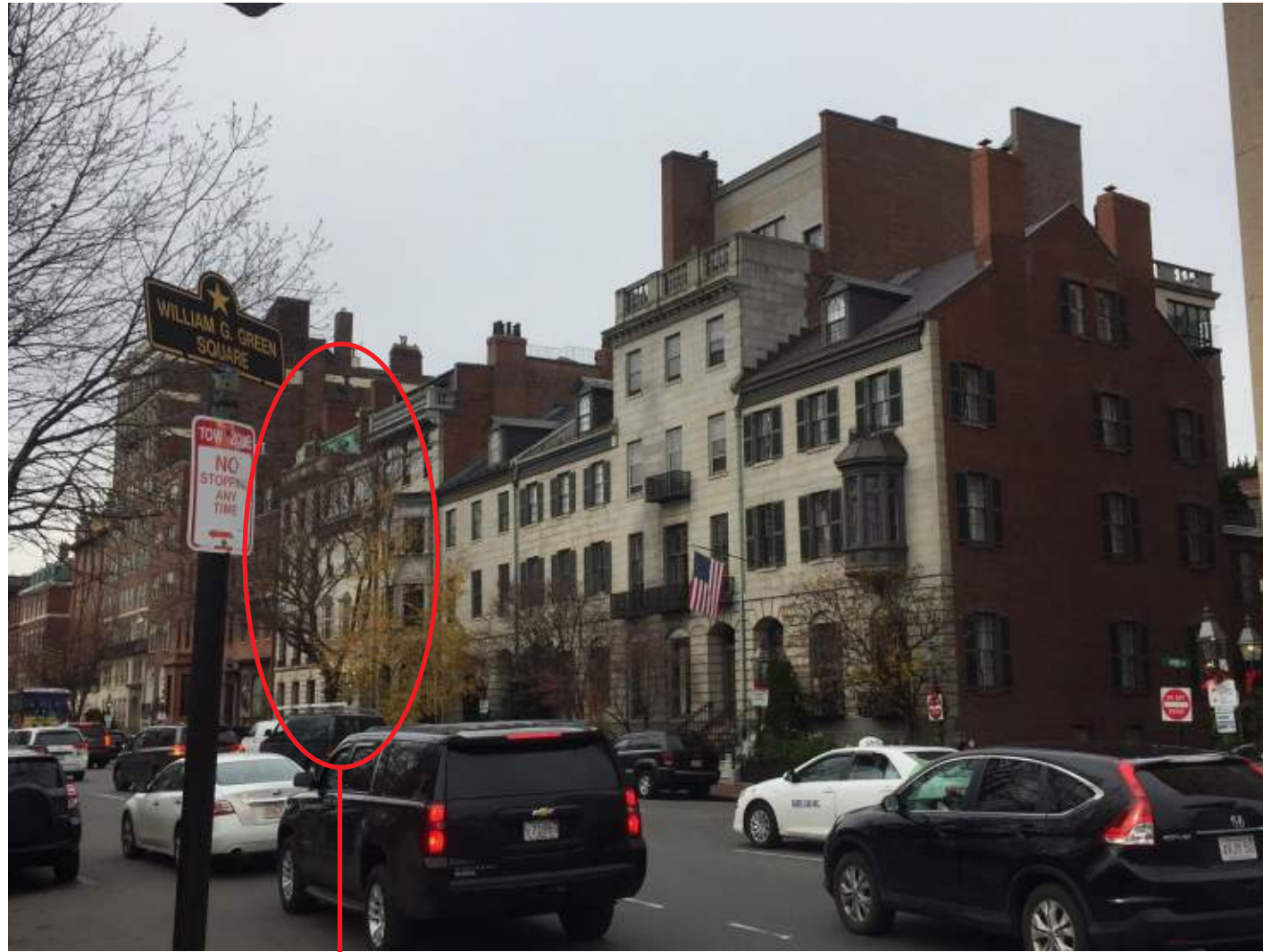
75 Beacon street existing facade
