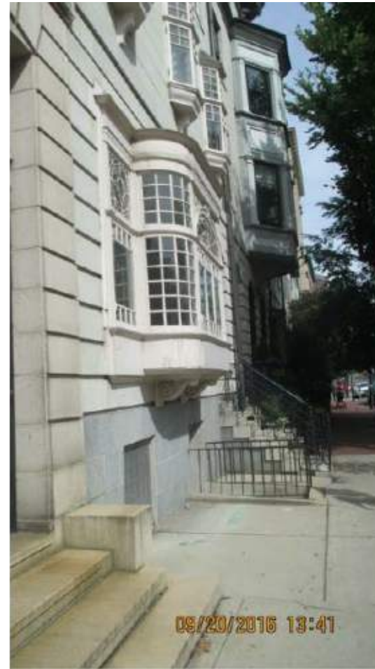
Bay window, 1st floor, Beacon St
