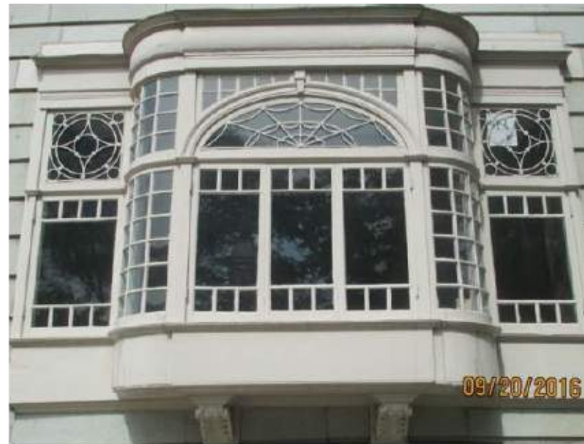
Bay Window, 1st floor, Beacon St.
