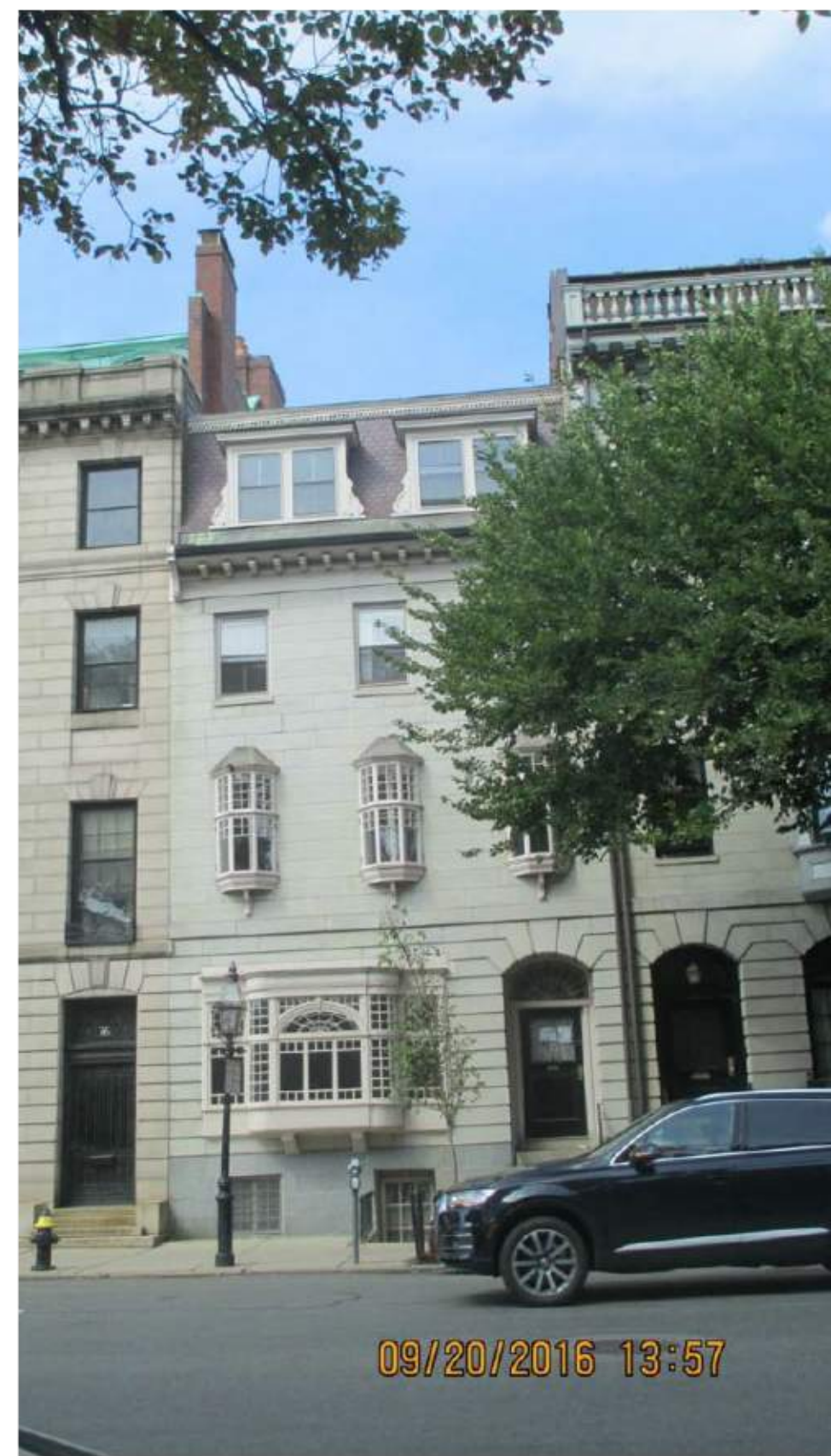
Front Elevation, Beacon St.
